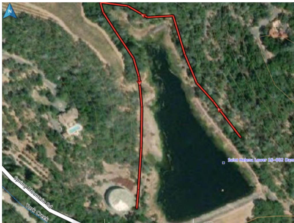
Lower Reservoir Trail
