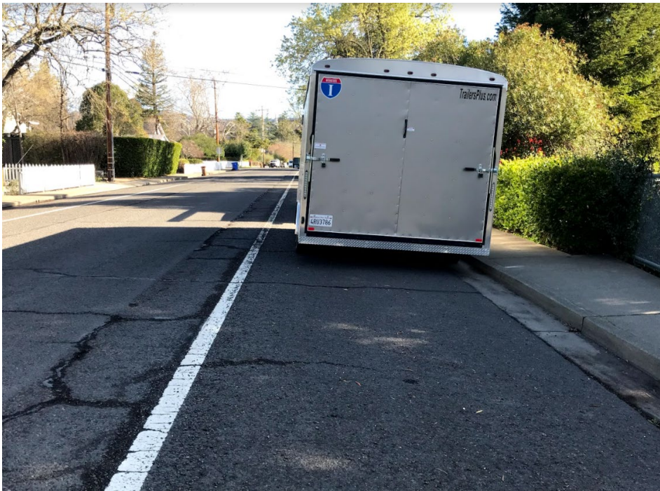
Spring St: A wide parking lane requires bicyclists to travel in rutted pavement in the travel lane.
