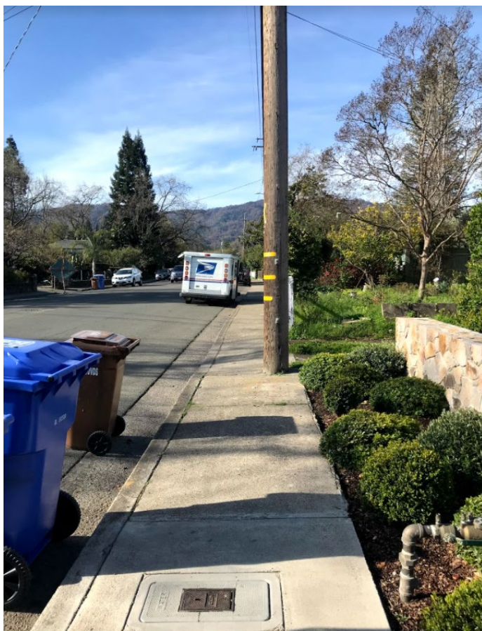
Spring St: Sidewalks are substandard width and are obstructed by utility poles.
