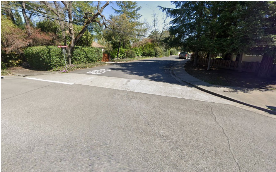
Spring St and Crane Ave: Curb ramps are absent at this unmarked crossing, and the stop bar is located after the crosswalk.
