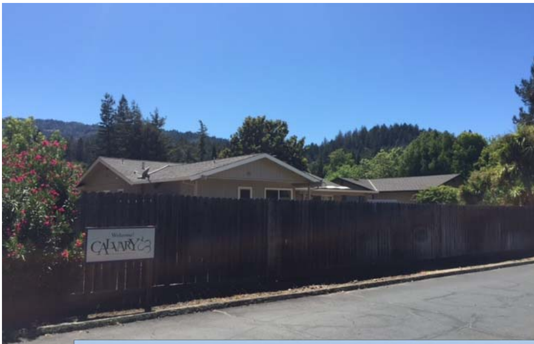
Photo 4. View of rear of property from Calvary driveway.
