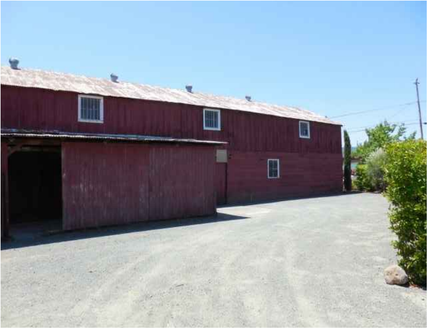
3 EXISTING BUILDING E - STORAGE BARN & COVERED WORK AREA EAST ELEVATION VIEW
