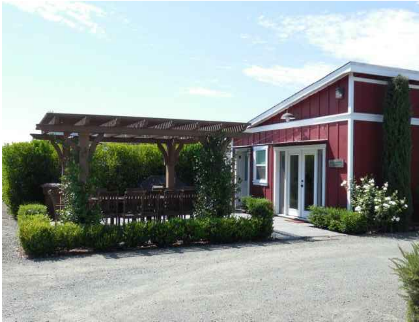
EXISTING BUILDING D - STORAGE #2 & PERGOLA NORTHEAST ELEVATION VIEW
