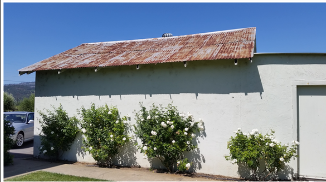
Figure 5. Garage to be demolished, showing addition at rear.
