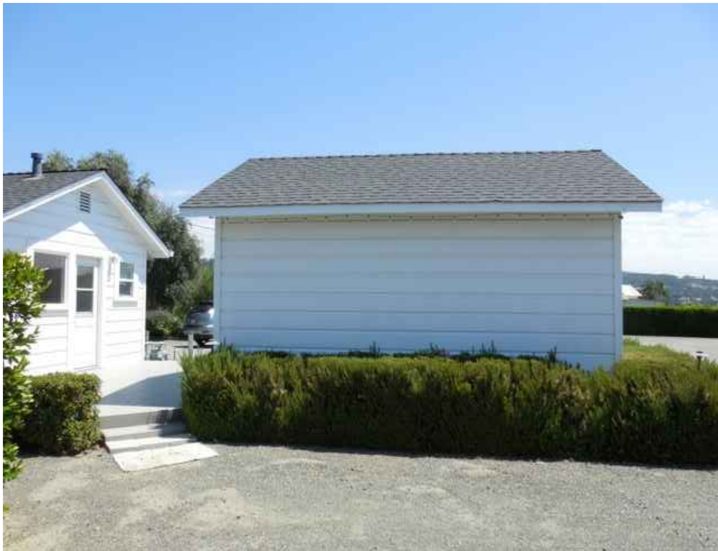
6 EXISTING BUILDING C - GUEST BEDROOM WEST ELEVATION VIEW
