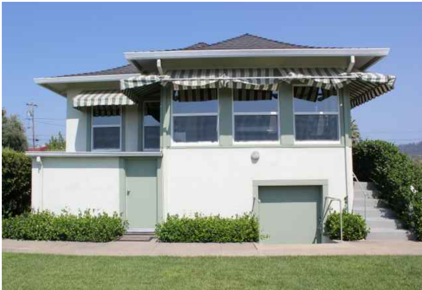
3 EXISTING BUILDING A - MAIN RESIDENCE SOUTH ELEVATION VIEW
