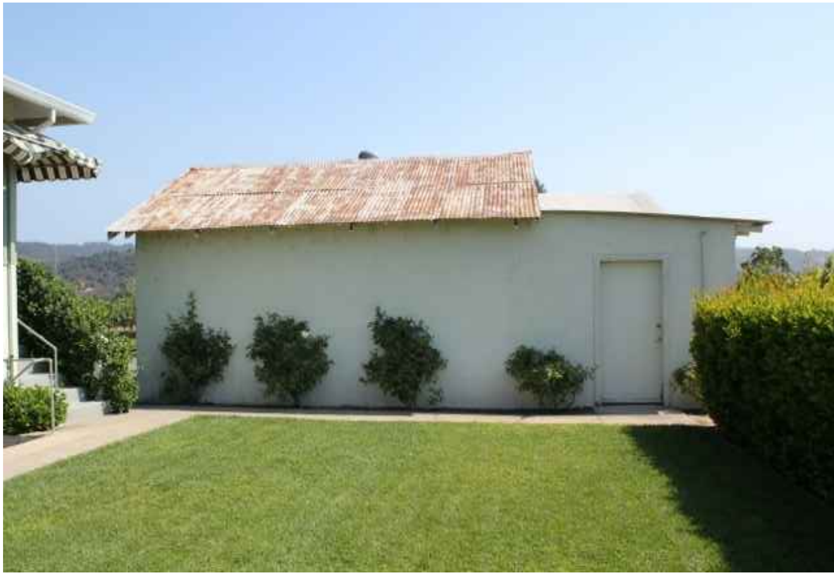
2 EXISTING GARAGE WEST ELEVATION VIEW
