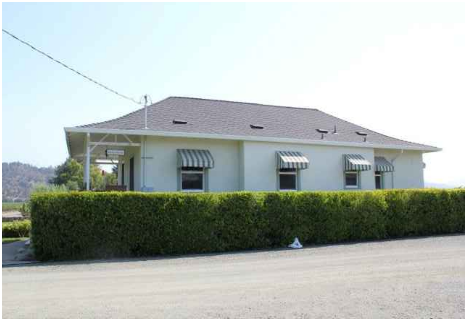
2 EXISTING BUILDING A - MAIN RESIDENCE WEST ELEVATION VIEW
