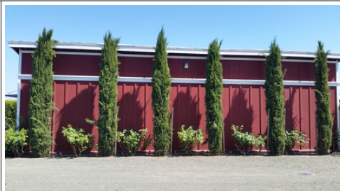
Figure 7. Non-historic storage shed to be relocated.
