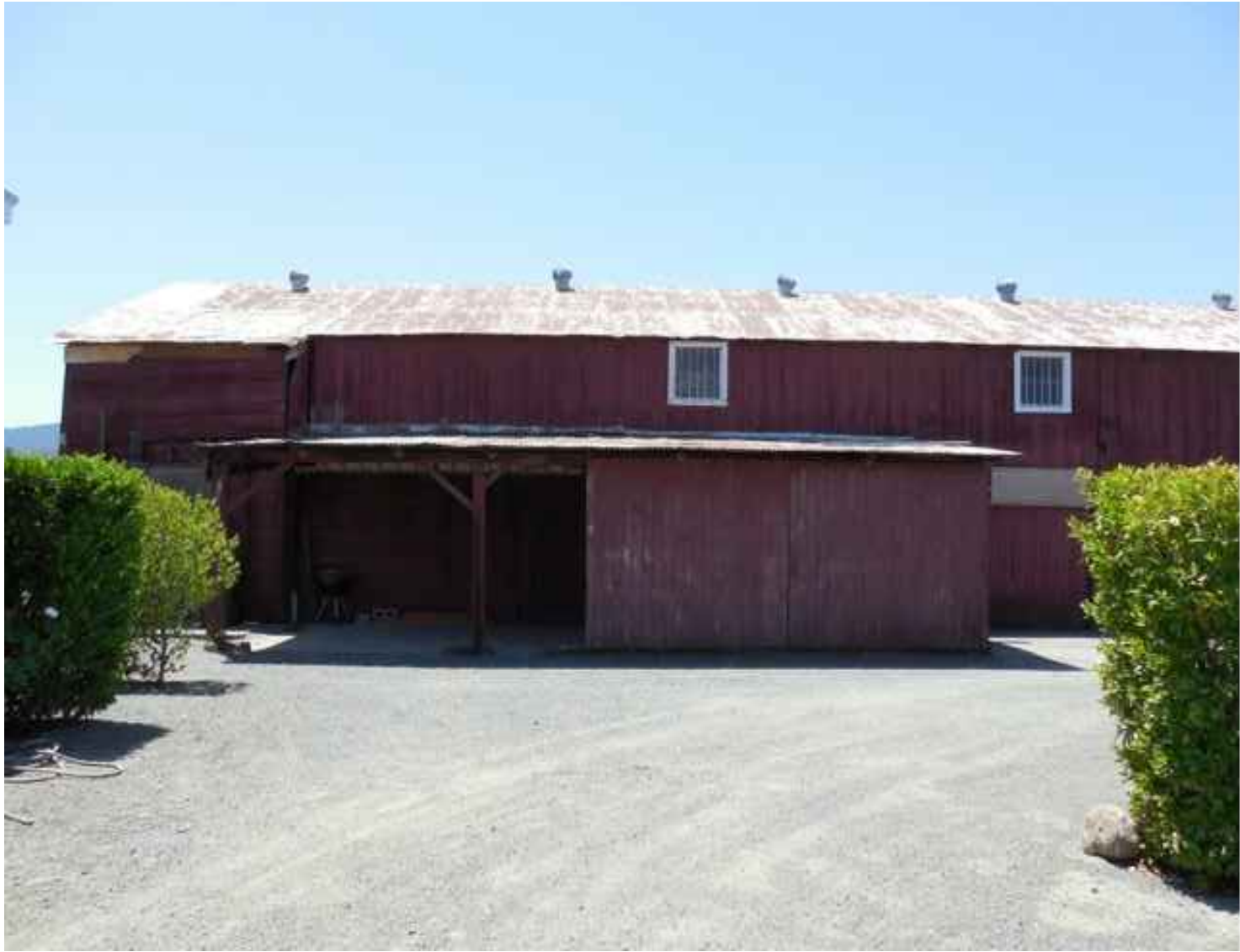
2 EXISTING BUILDING E - STORAGE BARN & COVERED WORK AREA EAST ELEVATION VIEW
