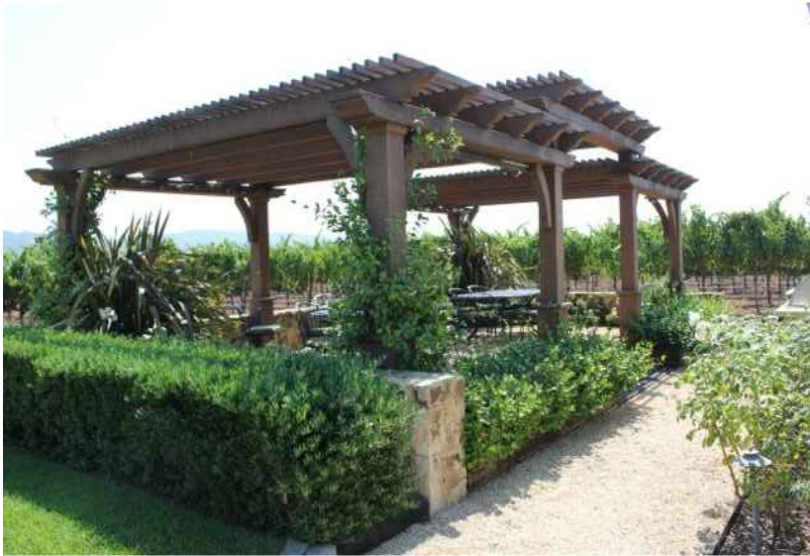
6 EXISTING PERGOLA NORTHWEST ELEVATION VIEW
