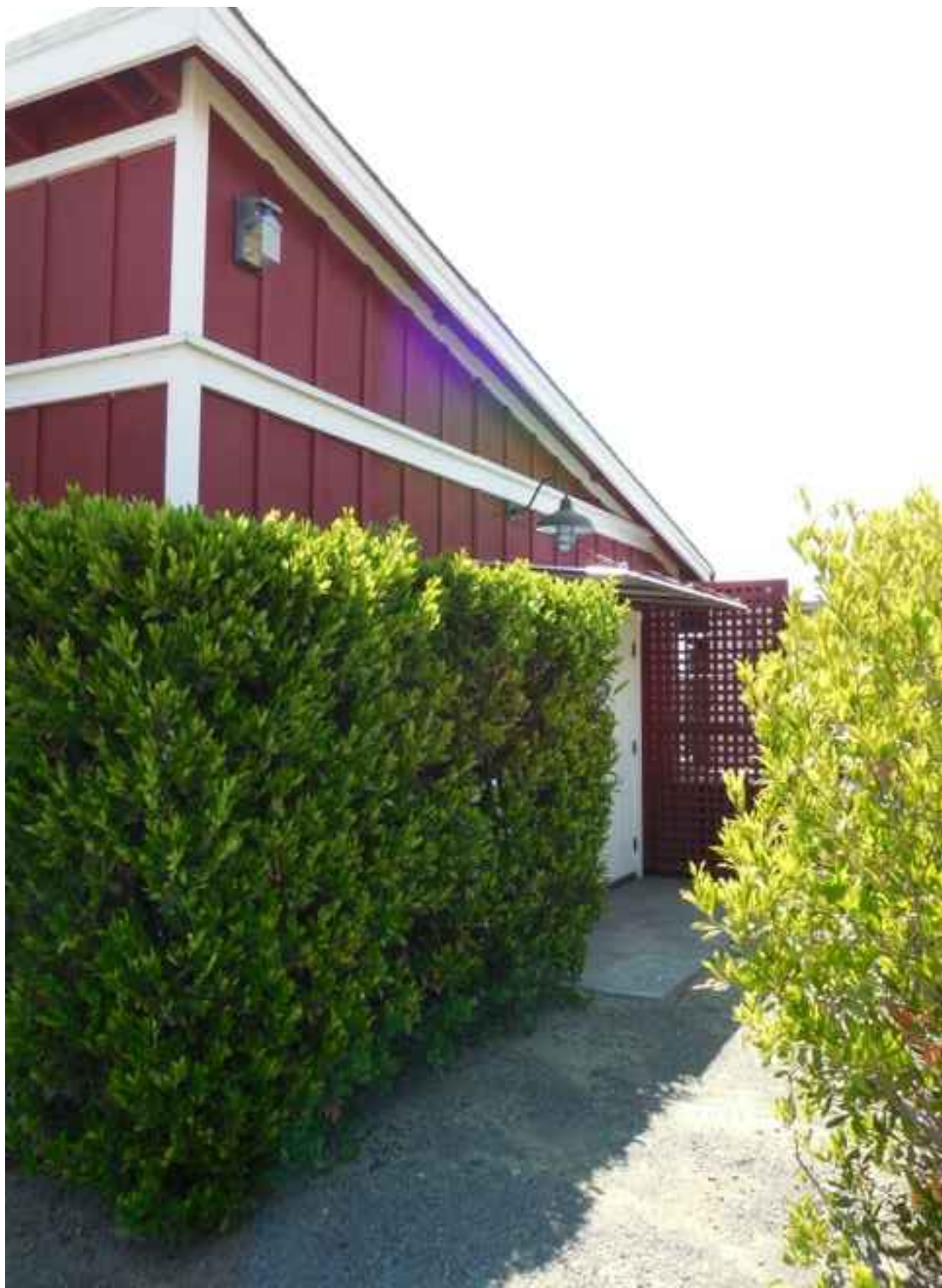
EXISTING BUILDING D - STORAGE #2 NORTHWEST ELEVATION VIEW
