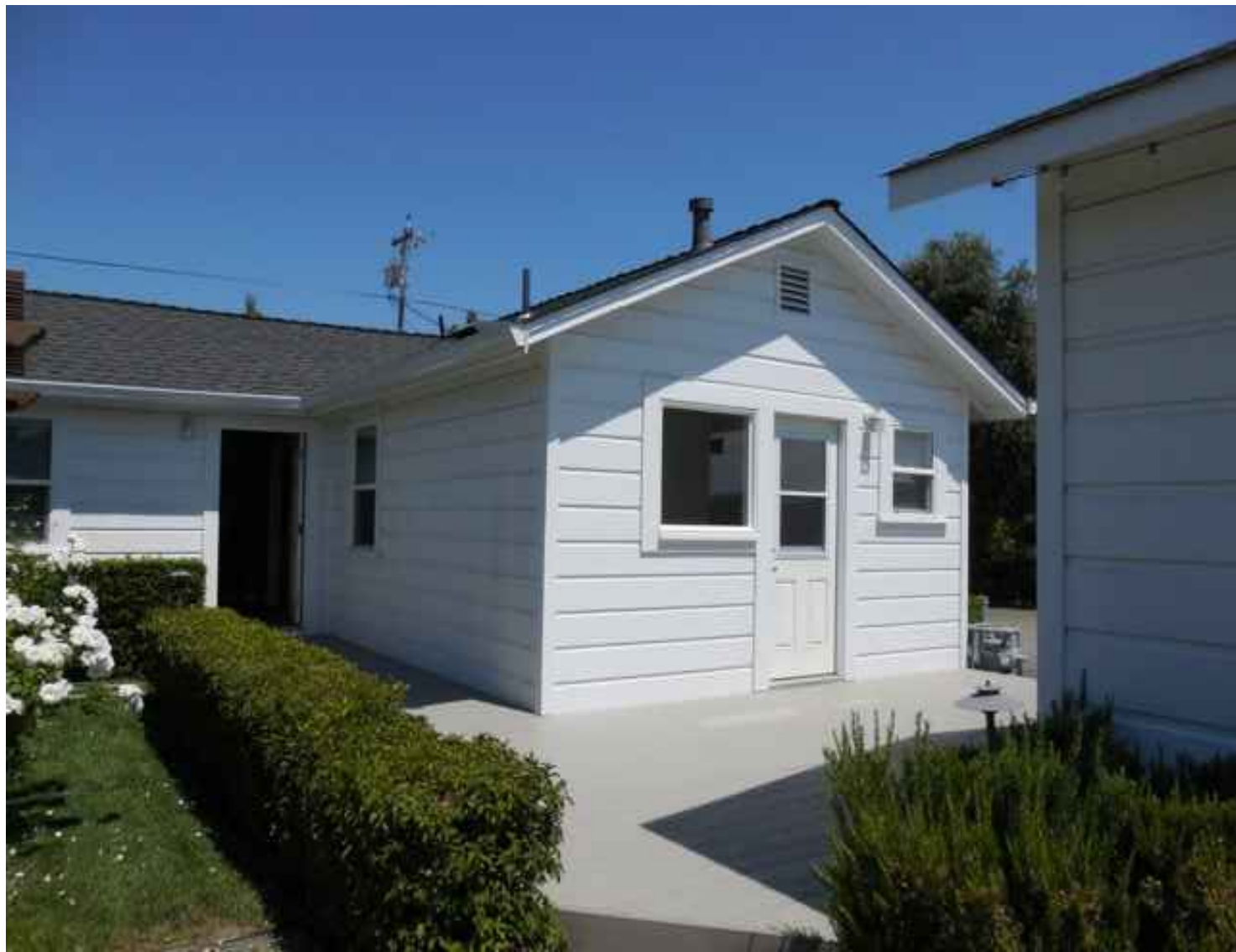
5 EXISTING BUILDING B - SECOND RESIDENCE SOUTHWEST ELEVATION VIEW
