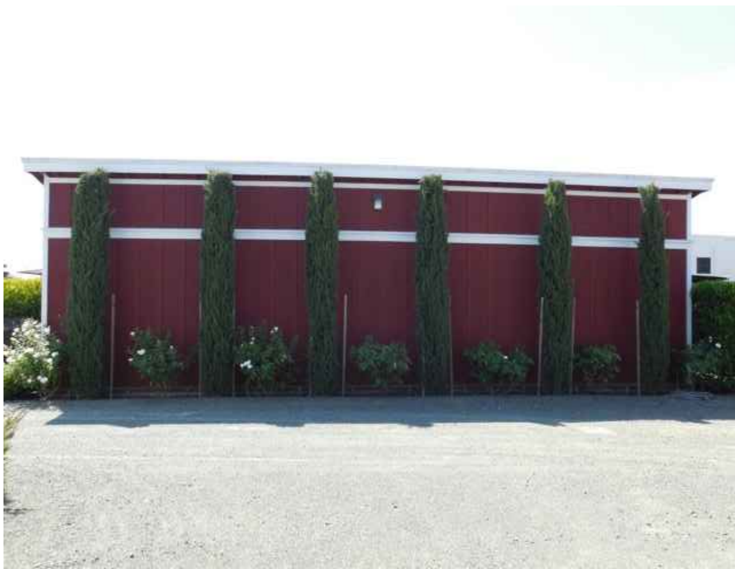
EXISTING BUILDING D - STORAGE #2 NORTH ELEVATION VIEW
