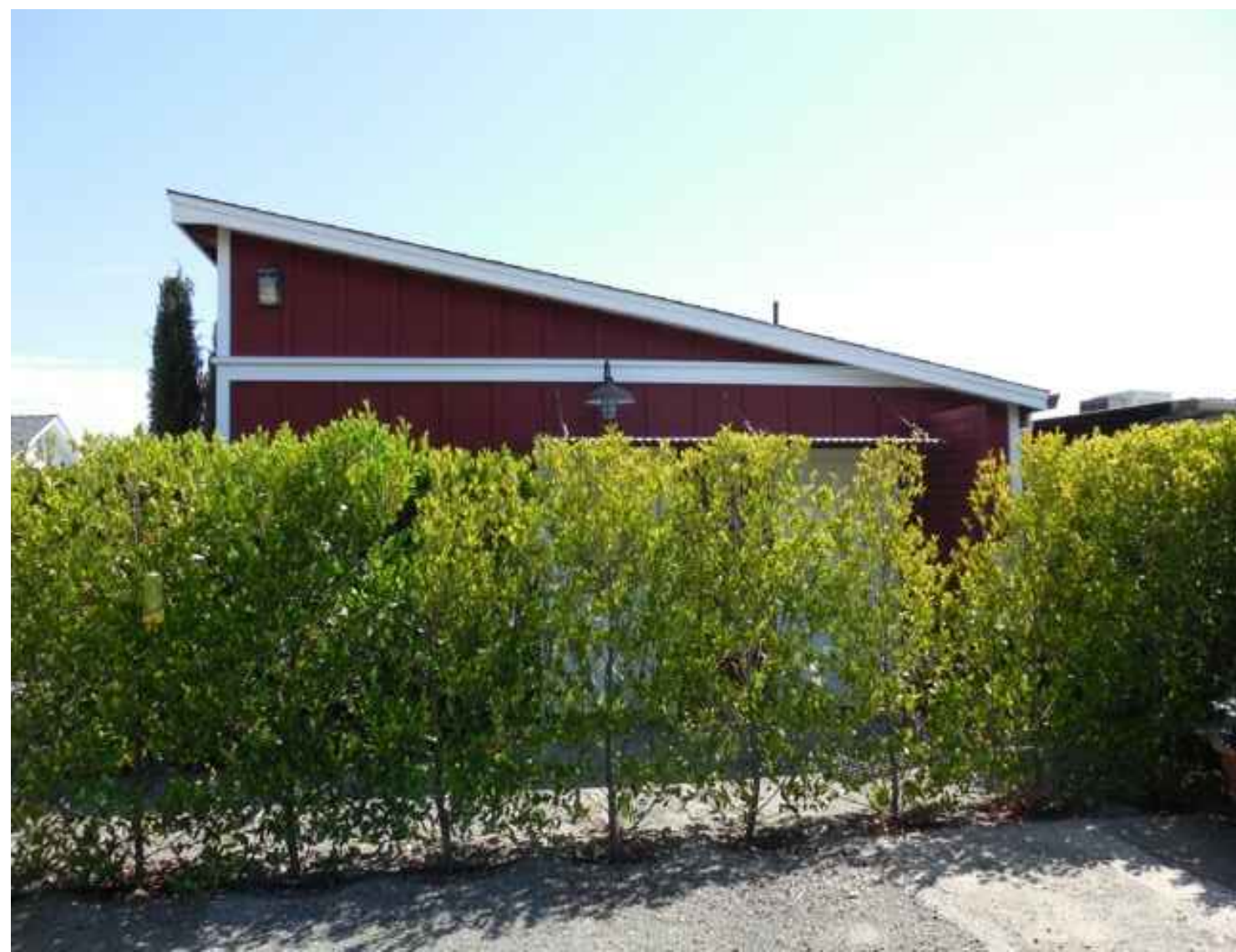
EXISTING BUILDING D - STORAGE #2 WEST ELEVATION VIEW
