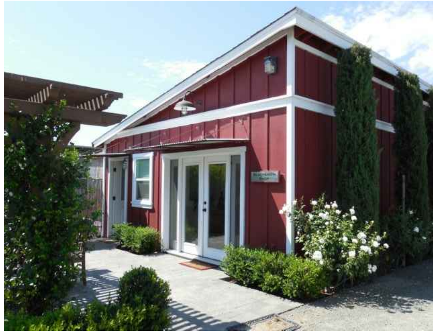
EXISTING BUILDING D - STORAGE #2 NORTHEAST ELEVATION VIEW
