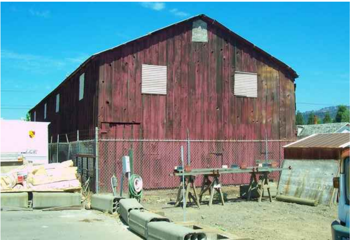
6 EXISTING BUILDING E - STORAGE BARN SOUTH ELEVATION VIEW
