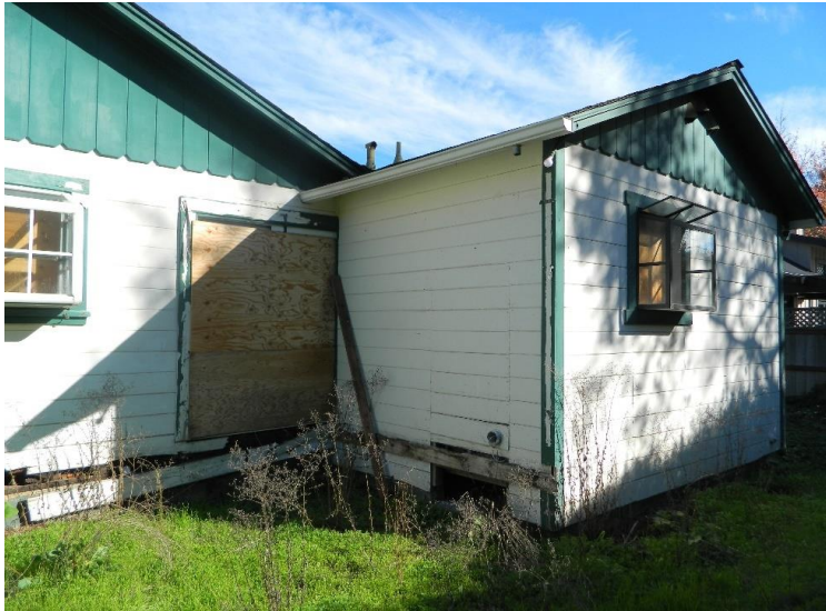
Figure 16. Parallel gable addition, facing east.
