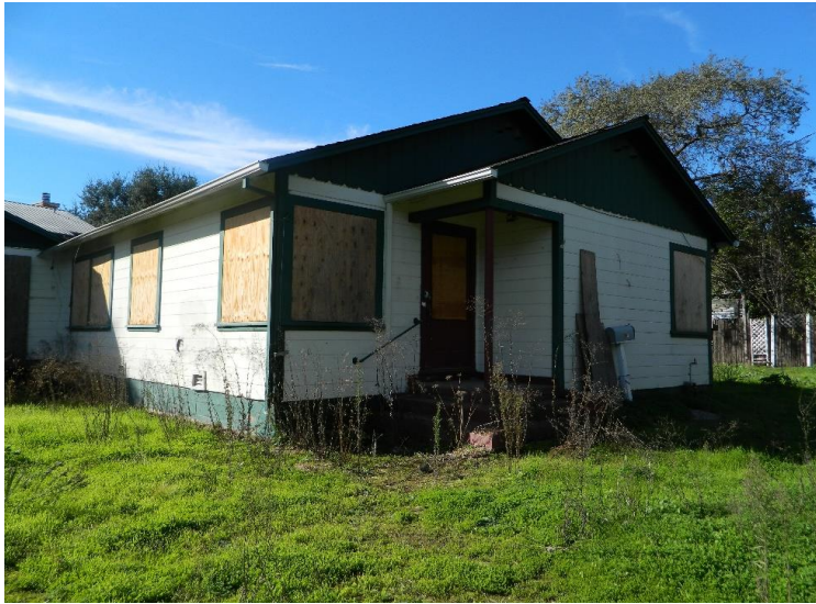
Figure 7. Northeast elevation, facing west.
