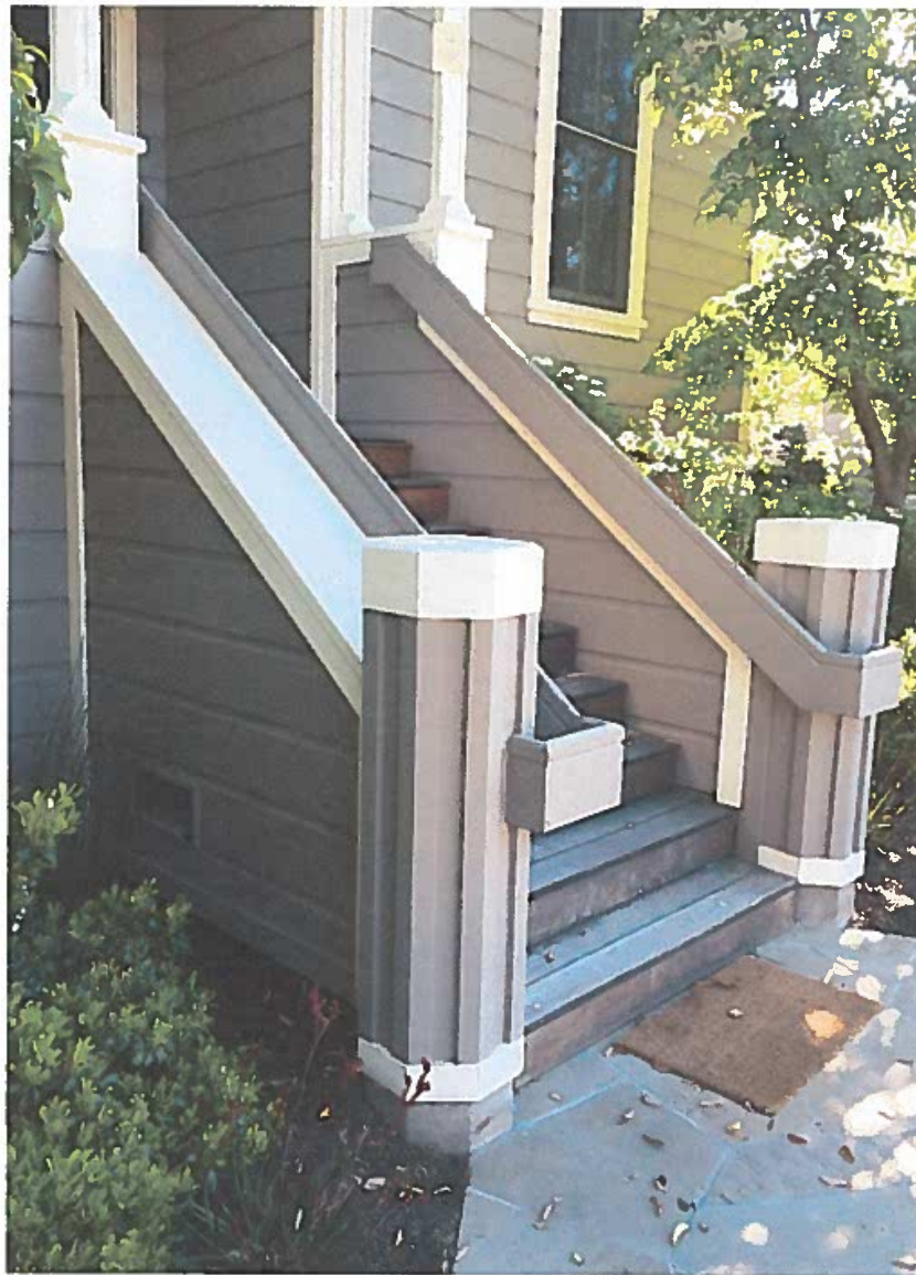
Photo 3: Detail of front stairs to be removed/replaced.
