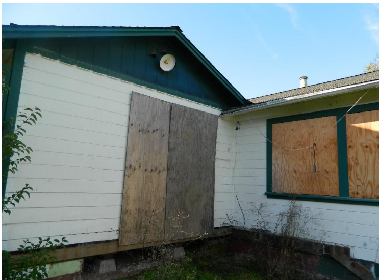
Figure 13. Southeast elevation, showing parallel gable addition.
