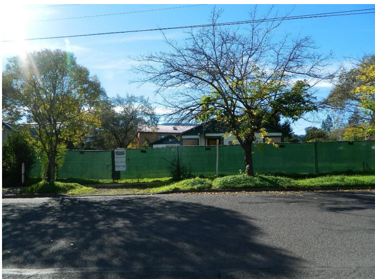
Figure 6. Ca. 1952 house, facing southwest.
