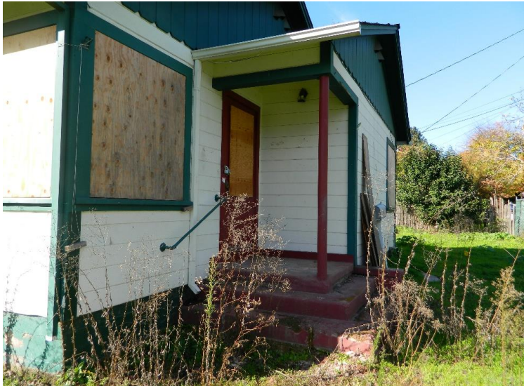
Figure 8. Northeast elevation, showing the porch stoop.
