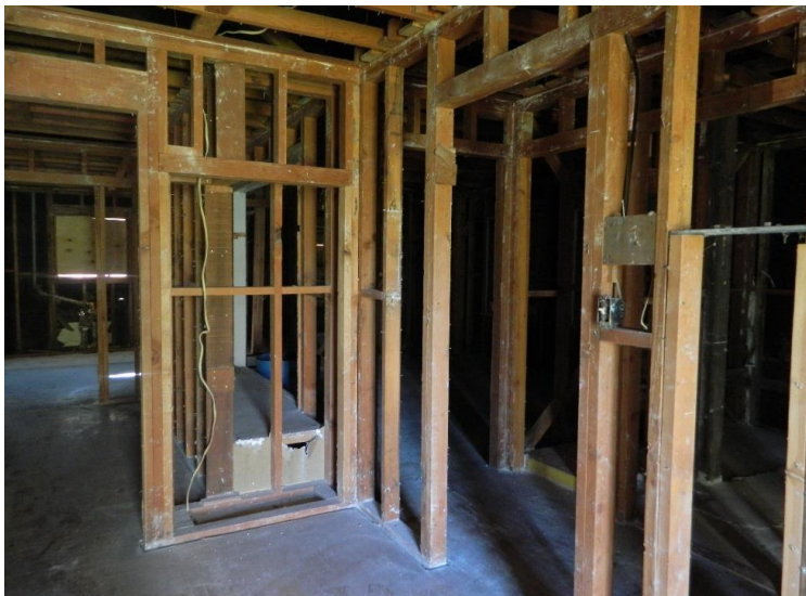
Figure 19. Interior view from the front door.
