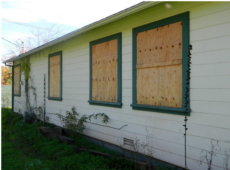
Figure 18. Northwest elevation, facing east.
