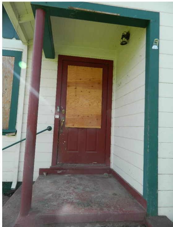
Figure 9. Front door, facing southwest.
