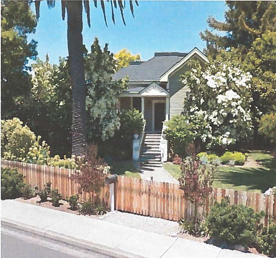
Photo 1: Front/West Elevation – existing stairs to be removed/replaced.
