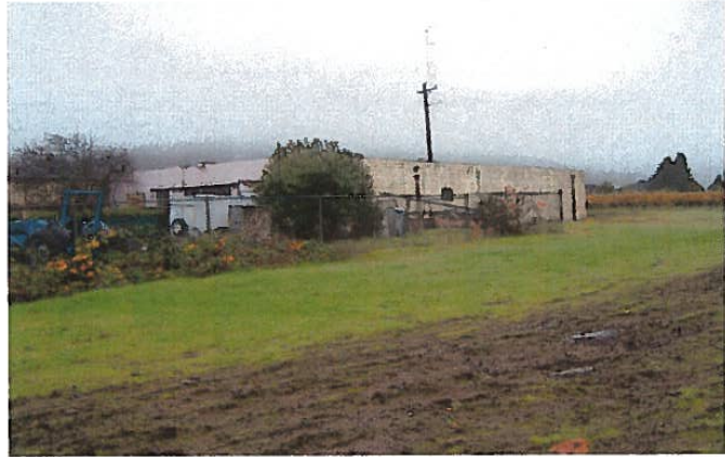
PHOTOGRAPH 1: LOOKING NORTHWEST ACROSS THE CENTRAL PORTION OF THE SITE.
