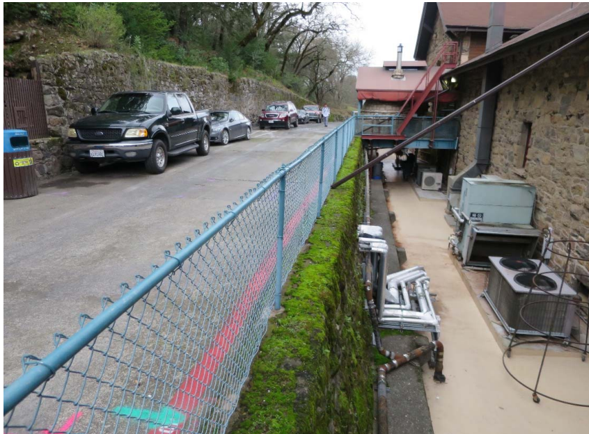
Image 3. Existing breezeway/rear elevation of Greystone building – View from southwest
