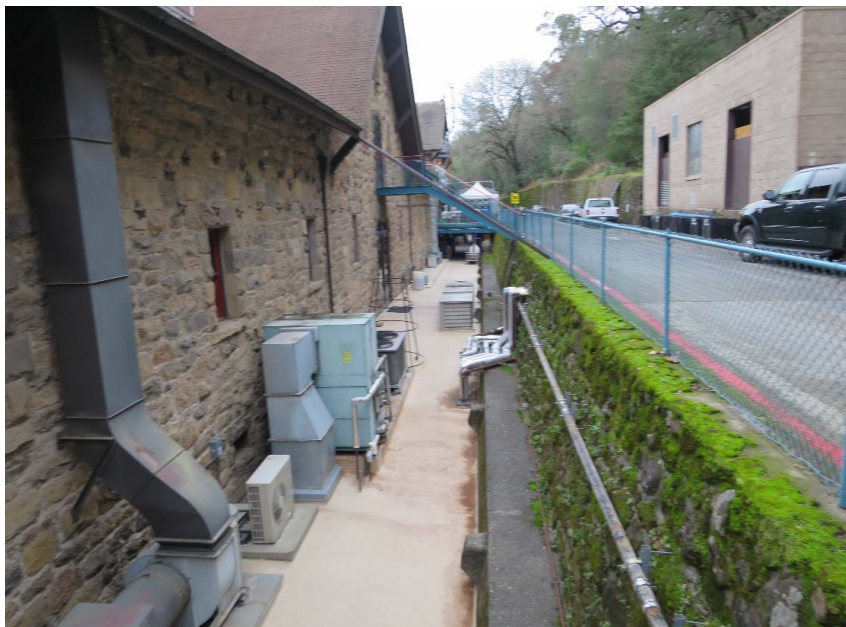
Image 2. Existing breezeway – View from northwest
