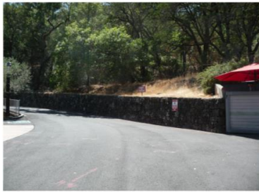
2 CAVE PORTAL EXISTING CONDITIONS
