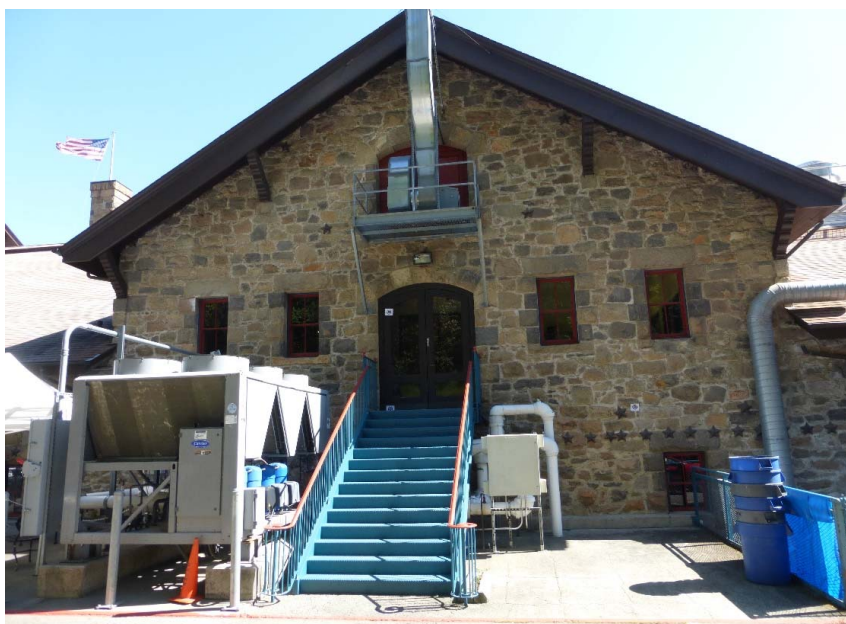
Image 7. Existing stair and mechanical equipment at south gable – view from west
