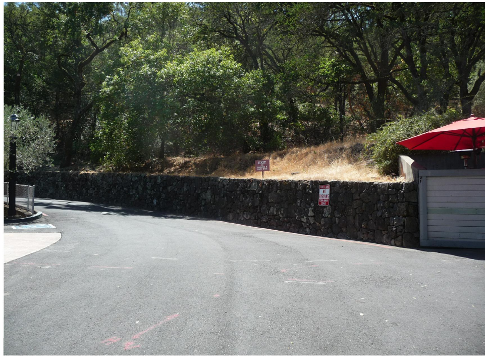
2 CAVE PORTAL EXISTING CONDITIONS
