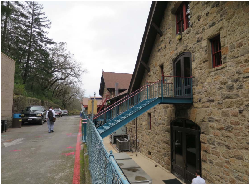
Image 4. Existing stairs at central gable – View from southwest
