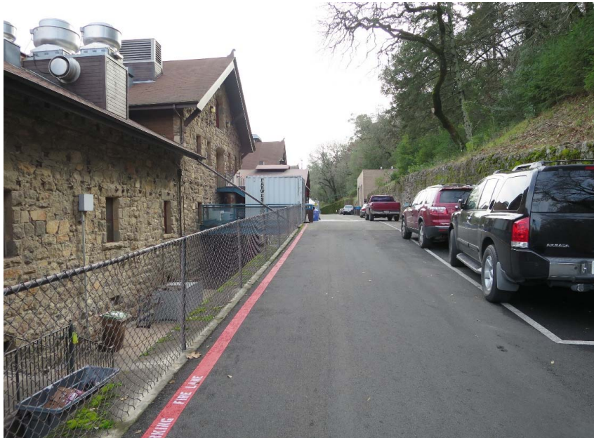
Image 1. Existing Rear Elevation of Greystone Building – view from northwest
