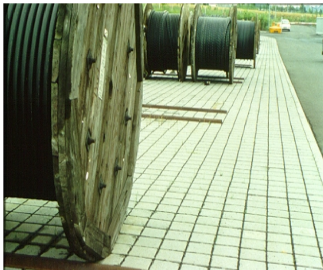
Figure 2. SF-Rima ™ in Storage Yard to Provide Permeable Pavement
