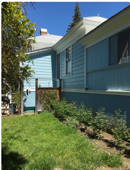
Right rear of house
