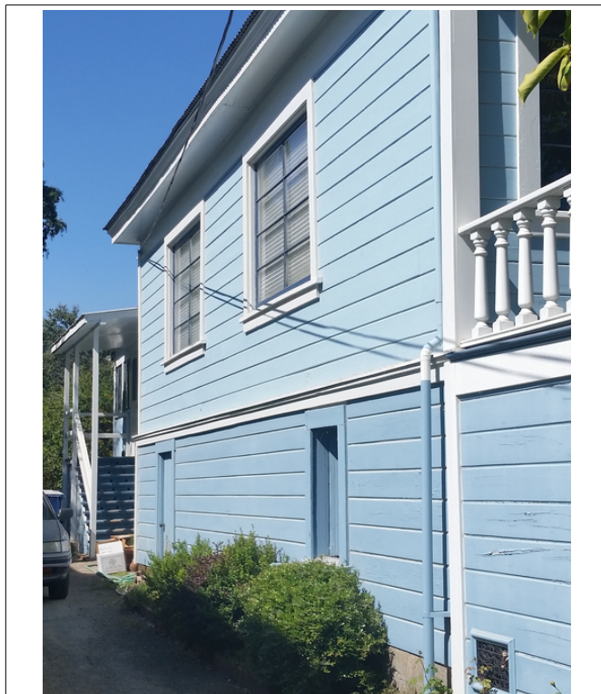
Figure 3. Large fixed wood and glass windows added to the east elevation.
