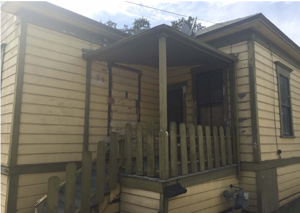
Photo 2. Front porch and entry before demolition.
