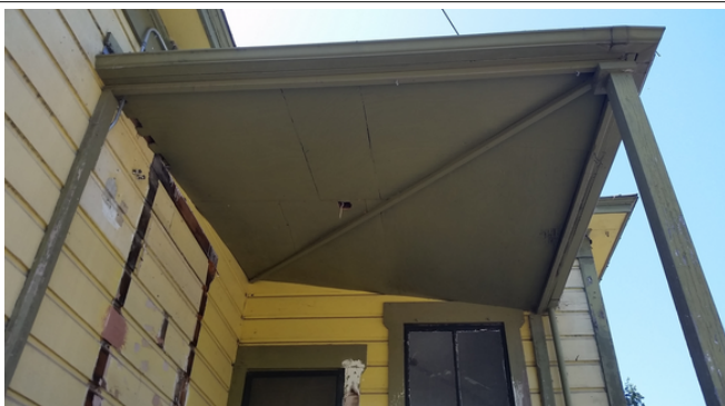
Figure 2. Porch showing original door location.
