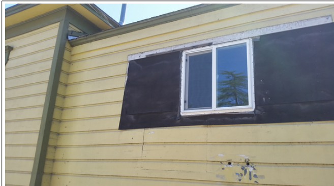
Figure 4. Non-historic rear addition.
