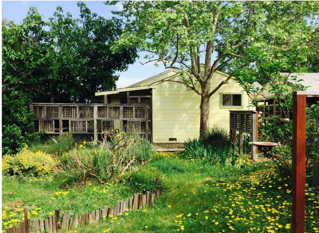
8 VIEW FACING SOUTHEAST
