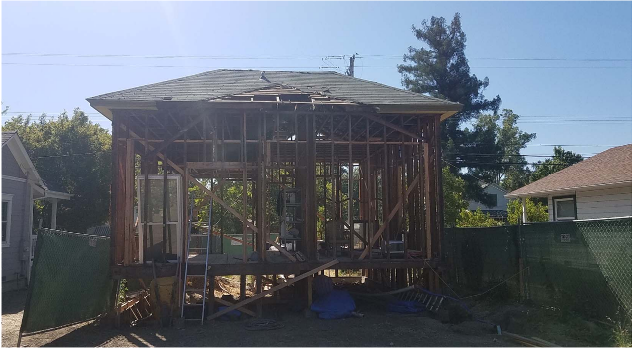
Photo 5. Rear of home as it exists today.
