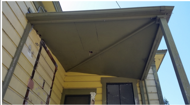
Figure 2. Porch showing original door location.
