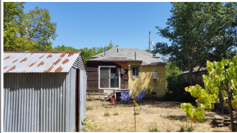
Figure 7. Non-historic shed and rear of the house.
