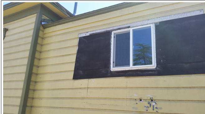
Figure 4. Non-historic rear addition.
