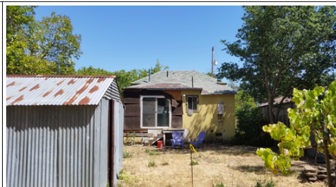
Figure 7. Non-historic shed and rear of the house.
