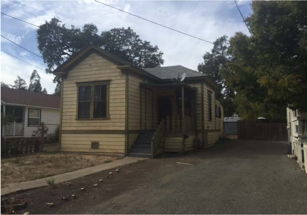
Photo 1. View of front of home and driveway before demolition.
