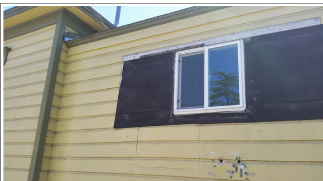
Figure 4. Non-historic rear addition.
