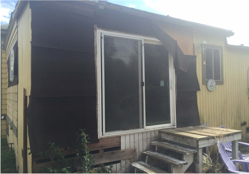
Photo 3. Rear of home before demolition.
