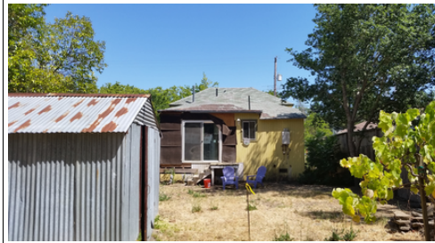
Figure 7. Non-historic shed and rear of the house.
