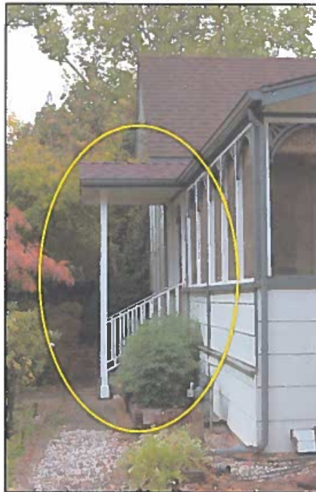
new front porch and steps
