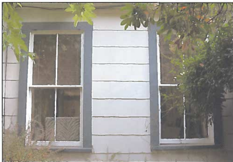
Figure 28: Two original windows, south elevation
