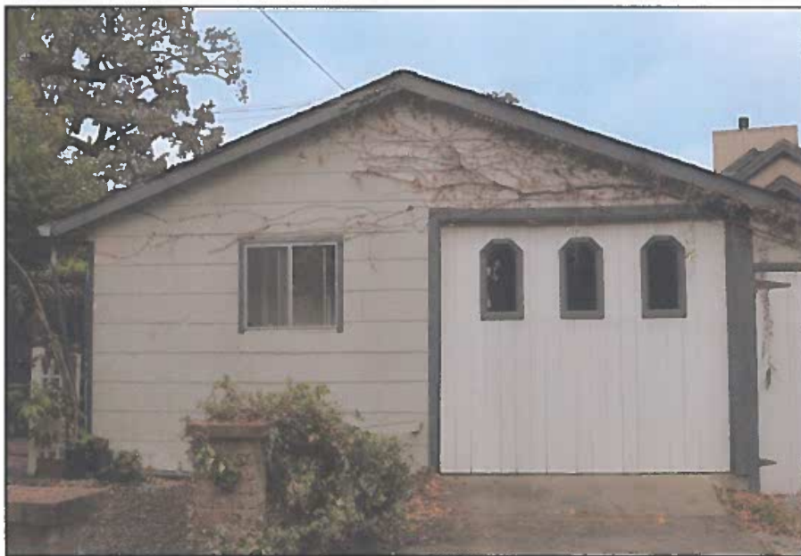
Figure 32: Garage, east elevation
