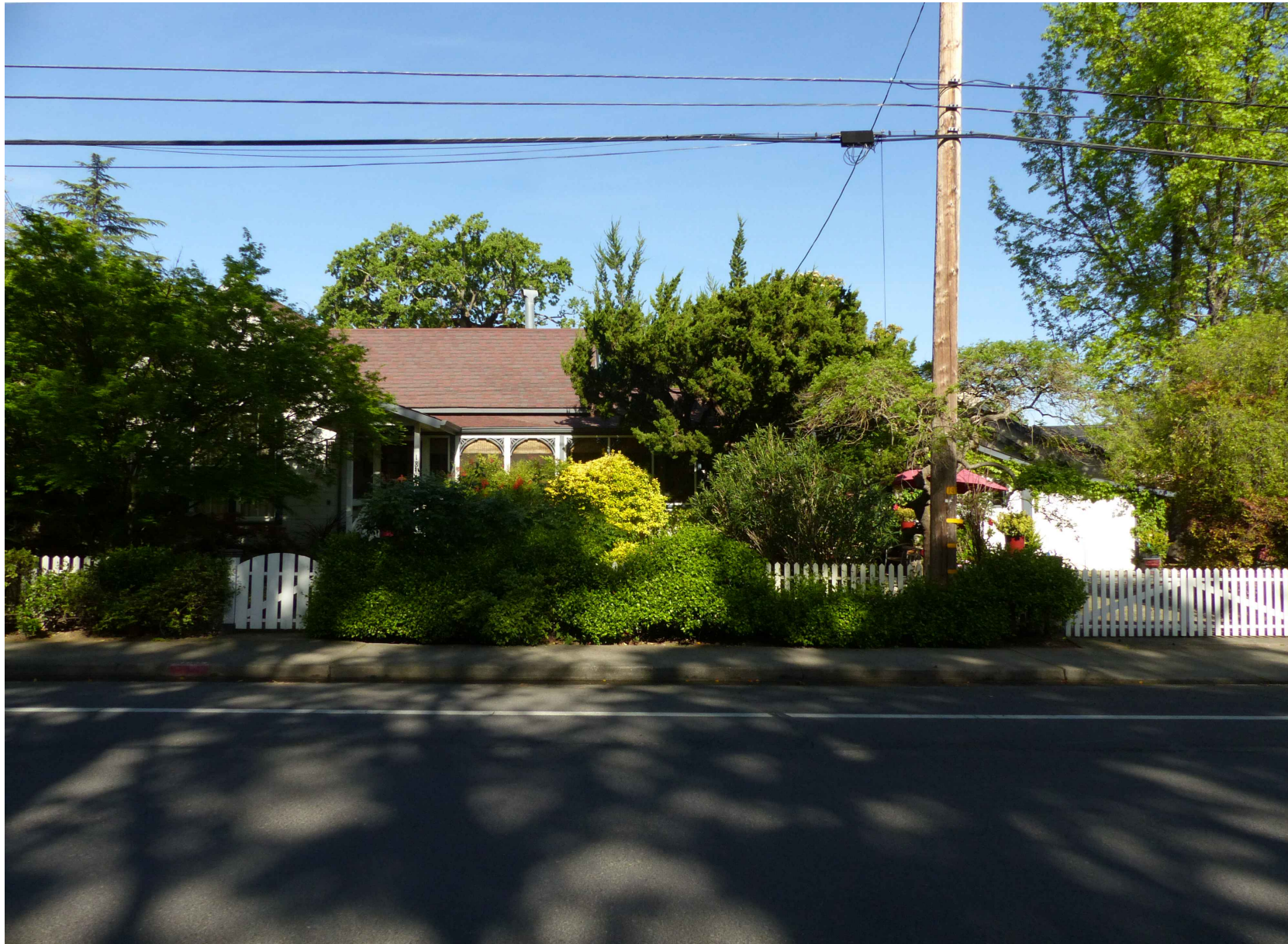
4 Existing Spring Street View
