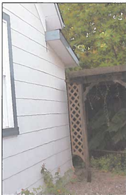
Figure 23: Addition off southwest corner of house
