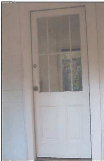
Figure 22: Original back door inside rear porch
