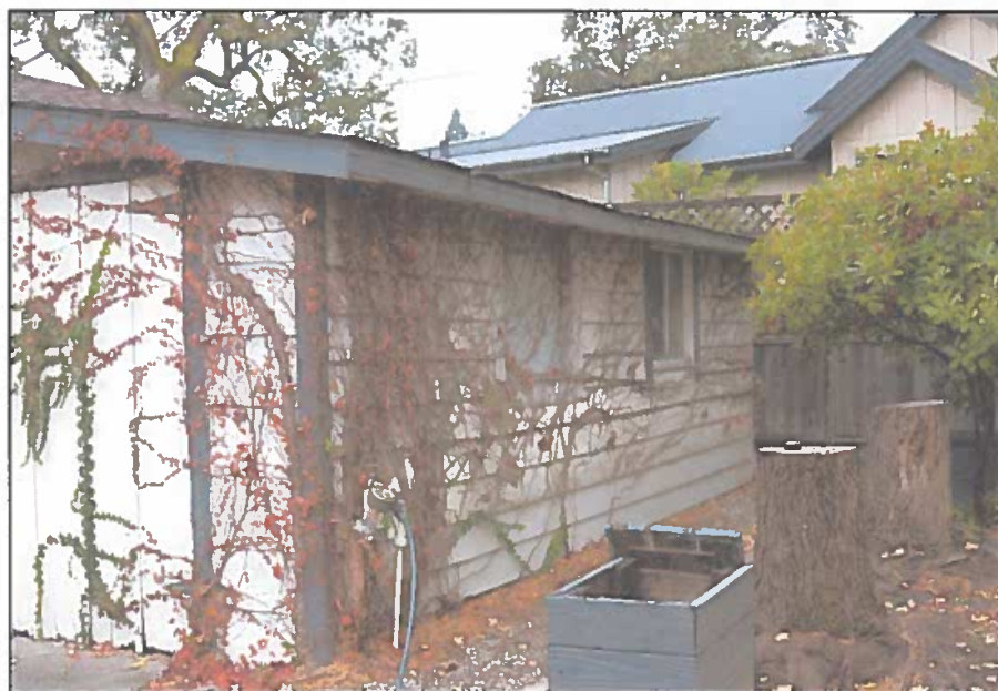
Figure 34: Garage, north elevation
