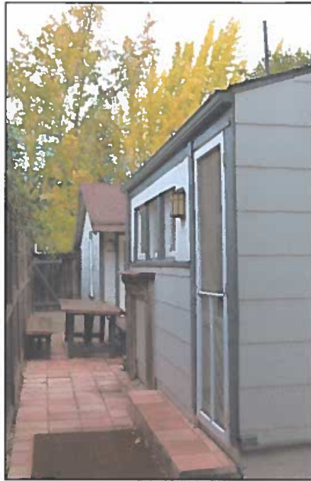
Figure 17: Back porch looking north
