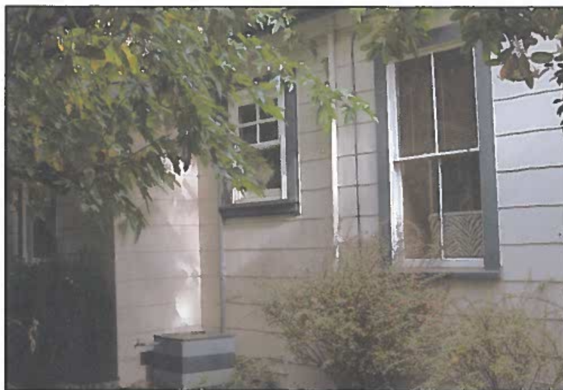
Figure 27: Modern window adjacent to original window, south elevation
