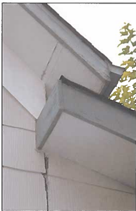
Figure 24: Junction of southwest addition at roof
