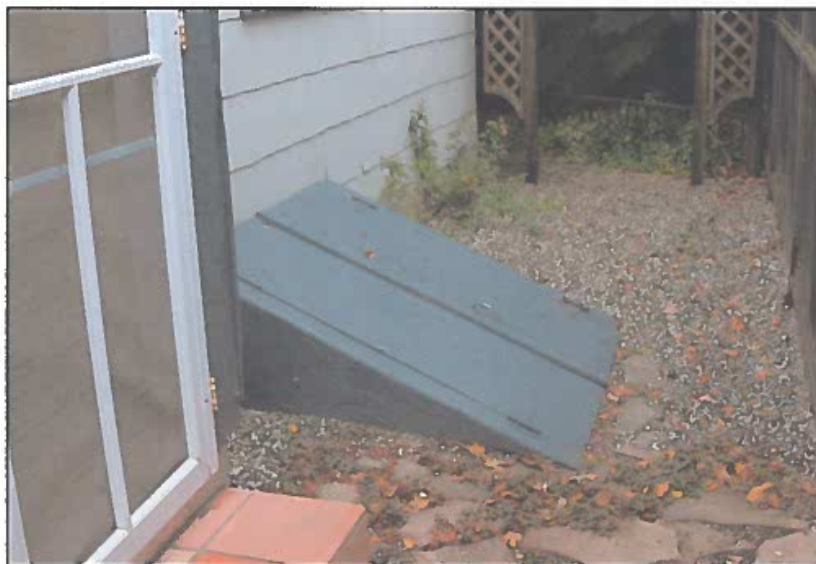
Figure 21: Cellar hatch, rear of house
