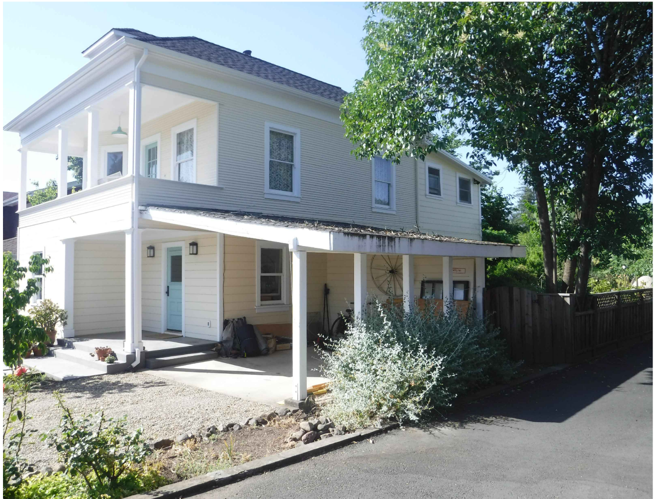
EXISTING WEST ELEVATION VIEW FROM SIDE YARD
