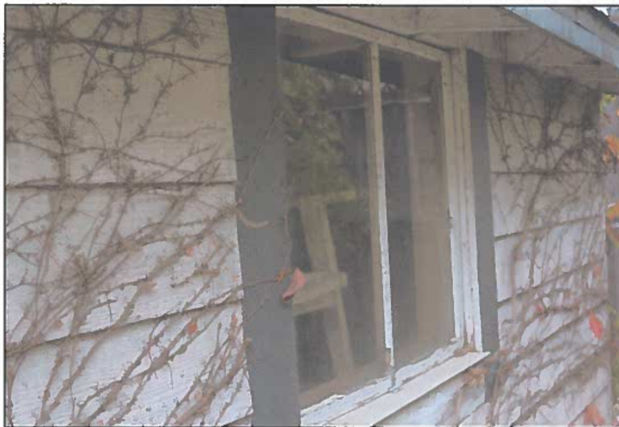
Figure 35: Garage, window on north elevation
