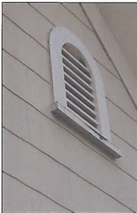
Figure 20: Wood, arched, louvered vent in gable of rear elevation
