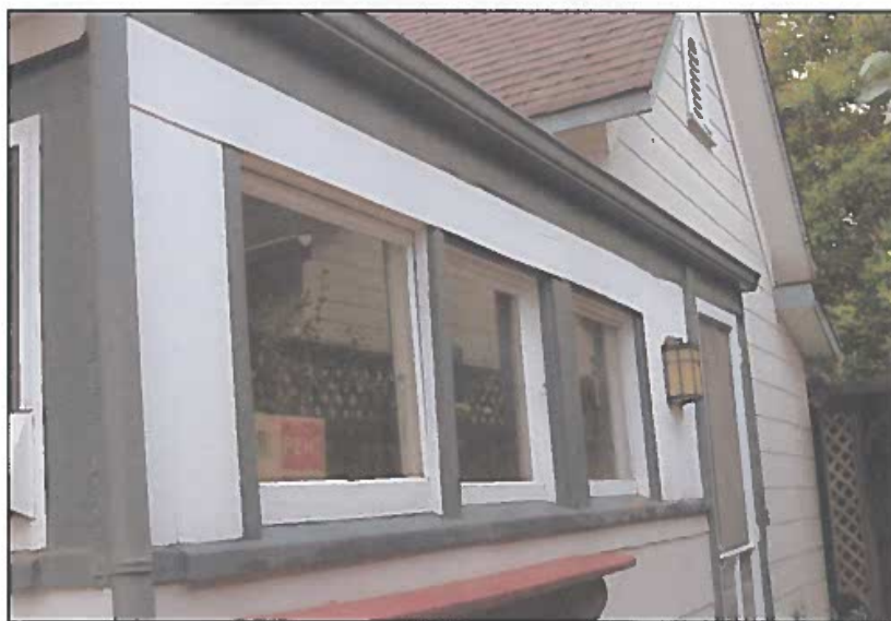
Figure 16: Infilled windows on back porch
