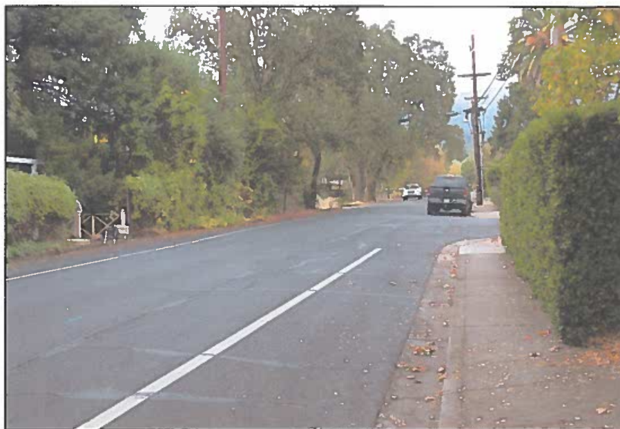
Figure 43: Streetscape, Spring Street looking south
