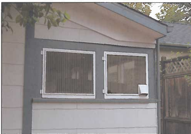
Figure 14: Infilled windows on back porch
