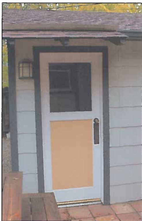
Figure 37: Garage, pedestrian door on west corner of south elevation
