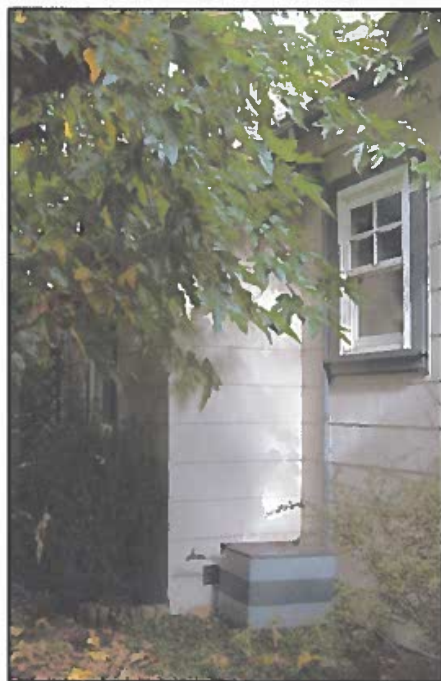
Figure 26: Southwest addition viewed from side yard (south)
