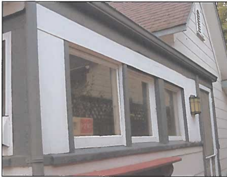
Modified back porch
