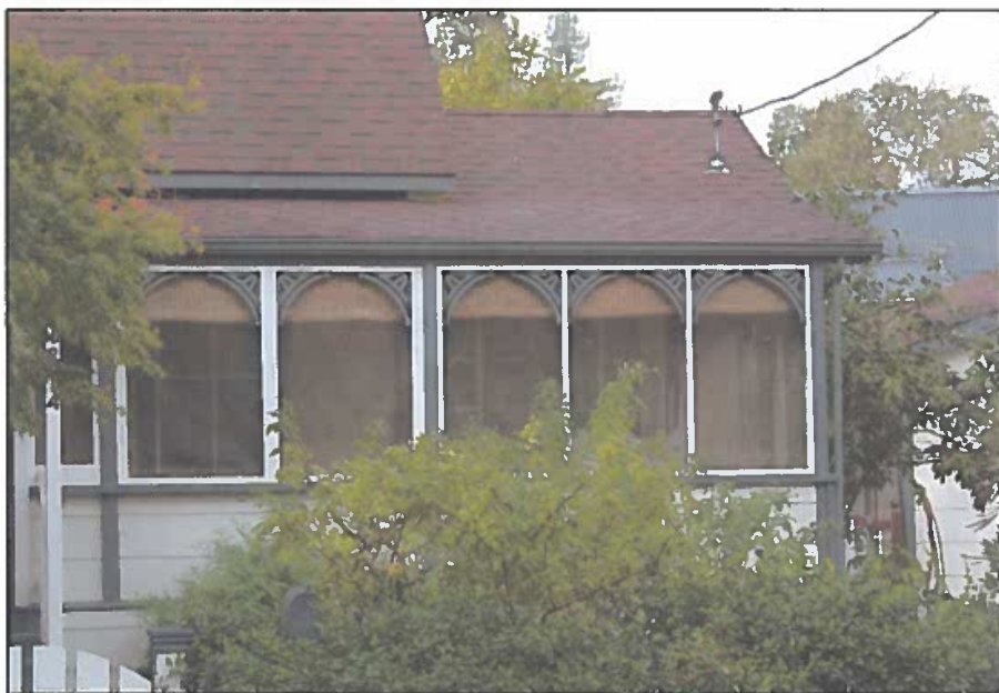
Figure 2: East elevation, screened porch
