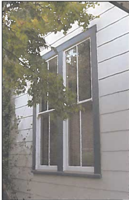
Figure 6: East elevation, pair of windows on gable end
