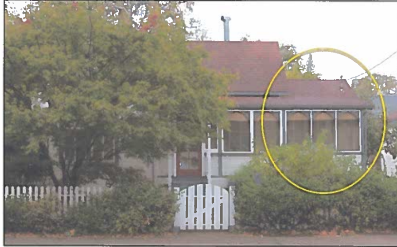
gable addition on north end and extended front porch
