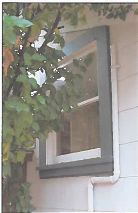
Figure 11: North facing window on original block of house
