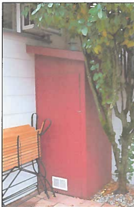
Figure 13: Mechanical closet at junction of north addition and original house
