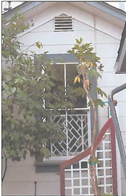
Figure 10: Window on gable end of north addition
