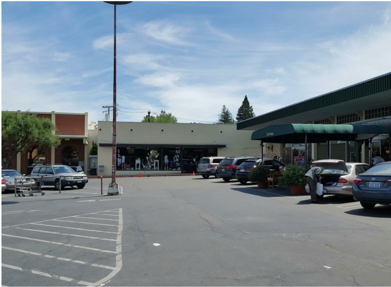
NORTH ELEVATION FROM SHOPPING CENTER PARKING LOT - LOOKING SOUTH
