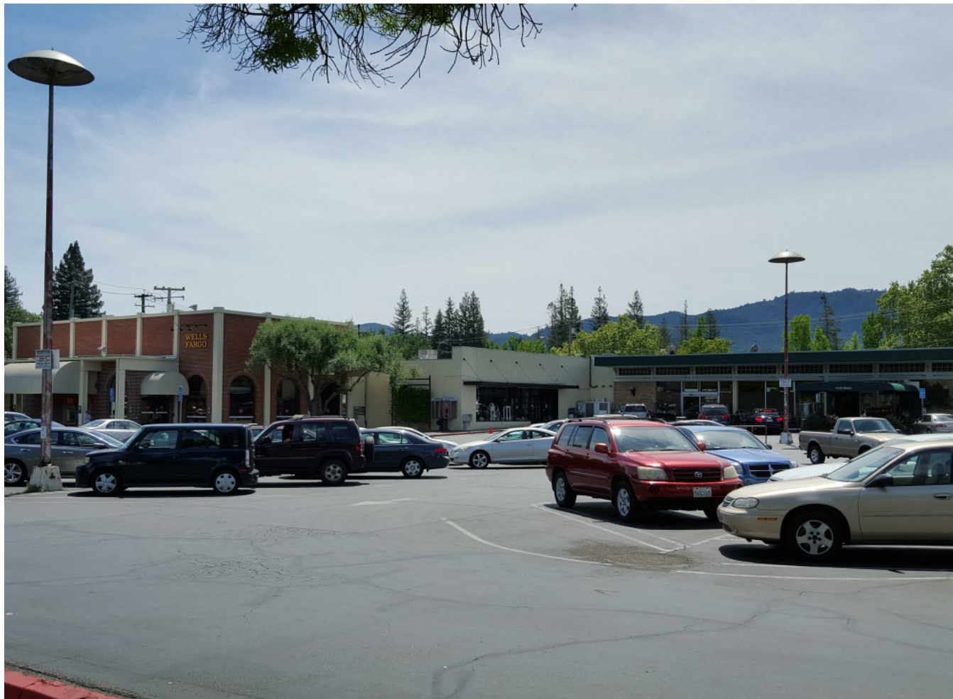
NORTH & EAST ELEVATIONS FROM MAIN STREET - LOOKING SOUTHWEST
