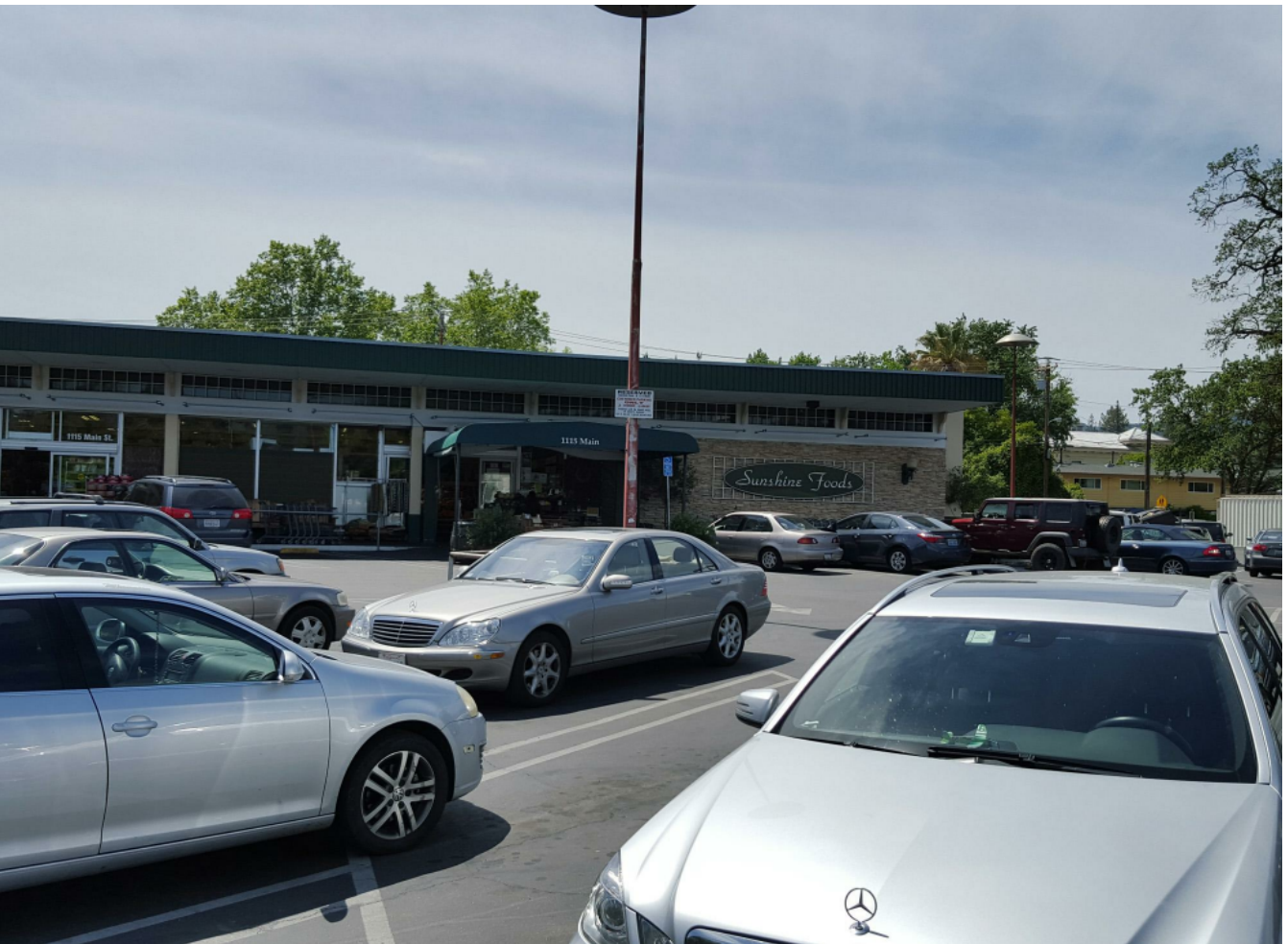
EAST ELEVATION OF ADJACENT SUNSHINE MARKET FROM PARKING LOT - LOOKING WEST
