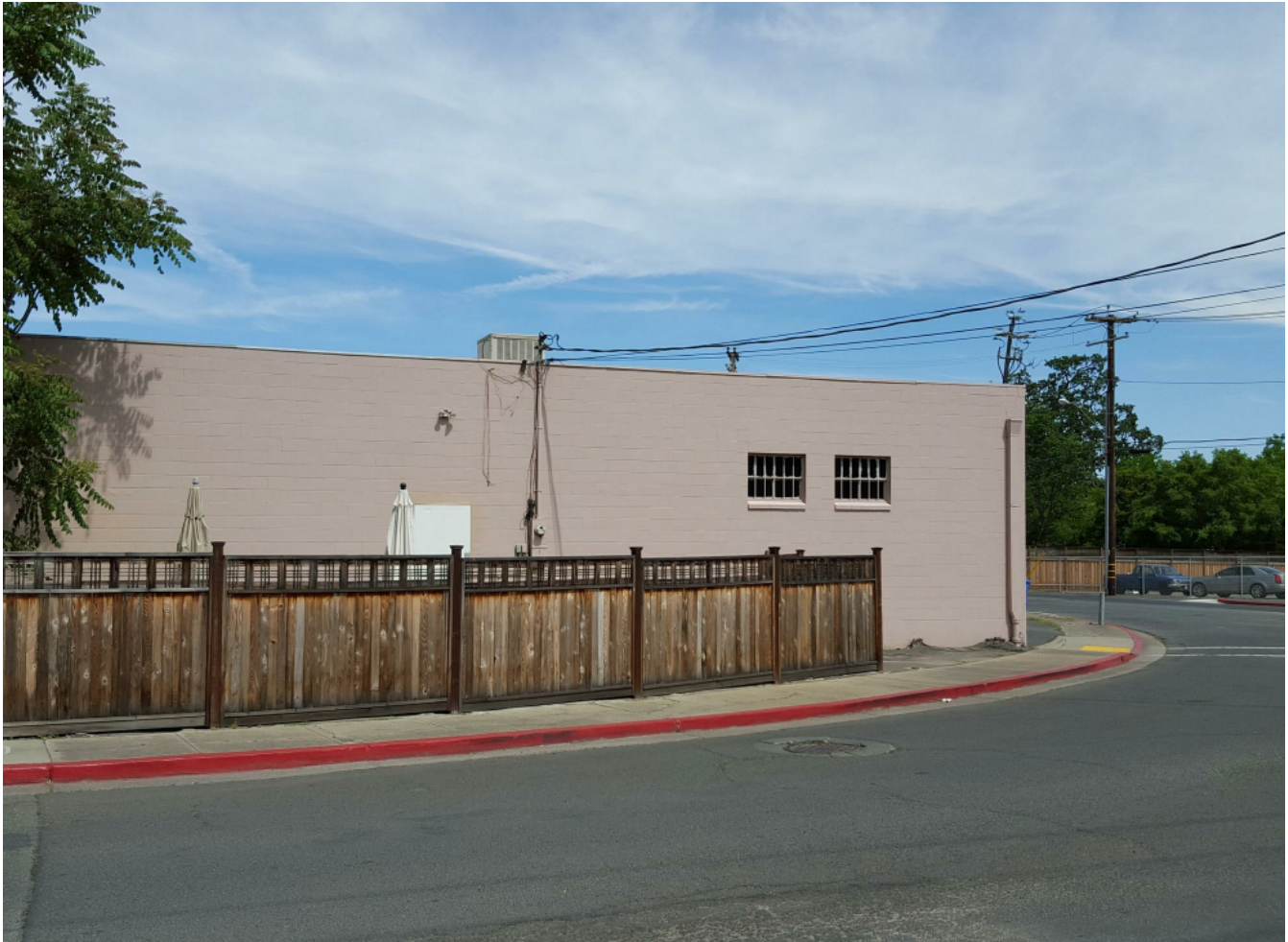
WEST ELEVATION FROM OAK AVENUE - LOOKING EAST
