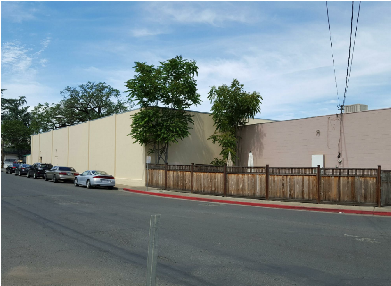
WEST ELEVATION FROM CORNER OF OAK AVENUE & MITCHELL DRIVE - LOOKING NORTHEAST
