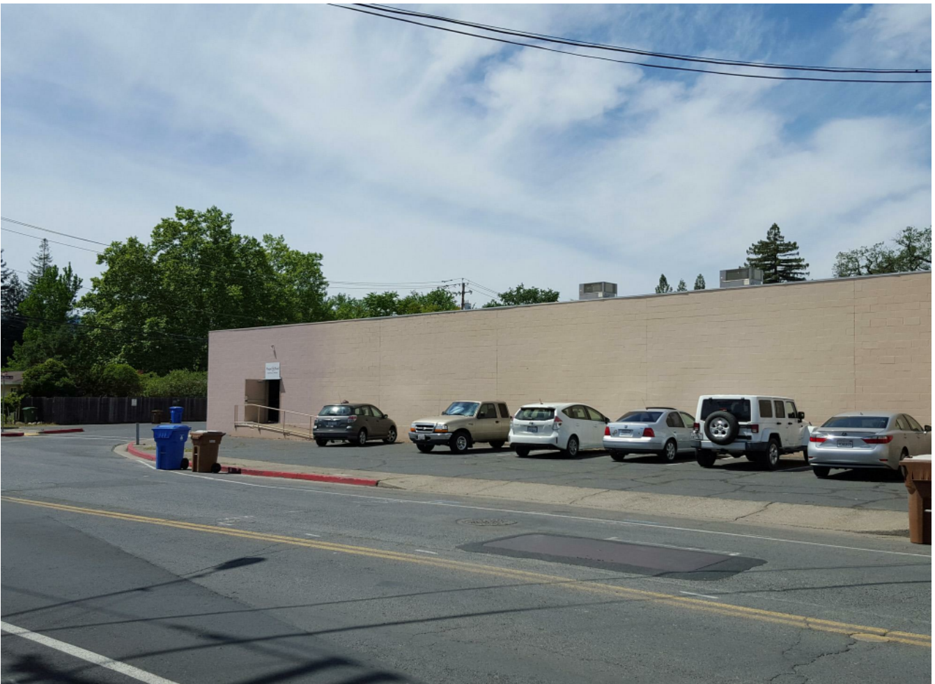
SOUTH ELEVATION FROM MITCHELL DRIVE - LOOKING NORTHWEST
