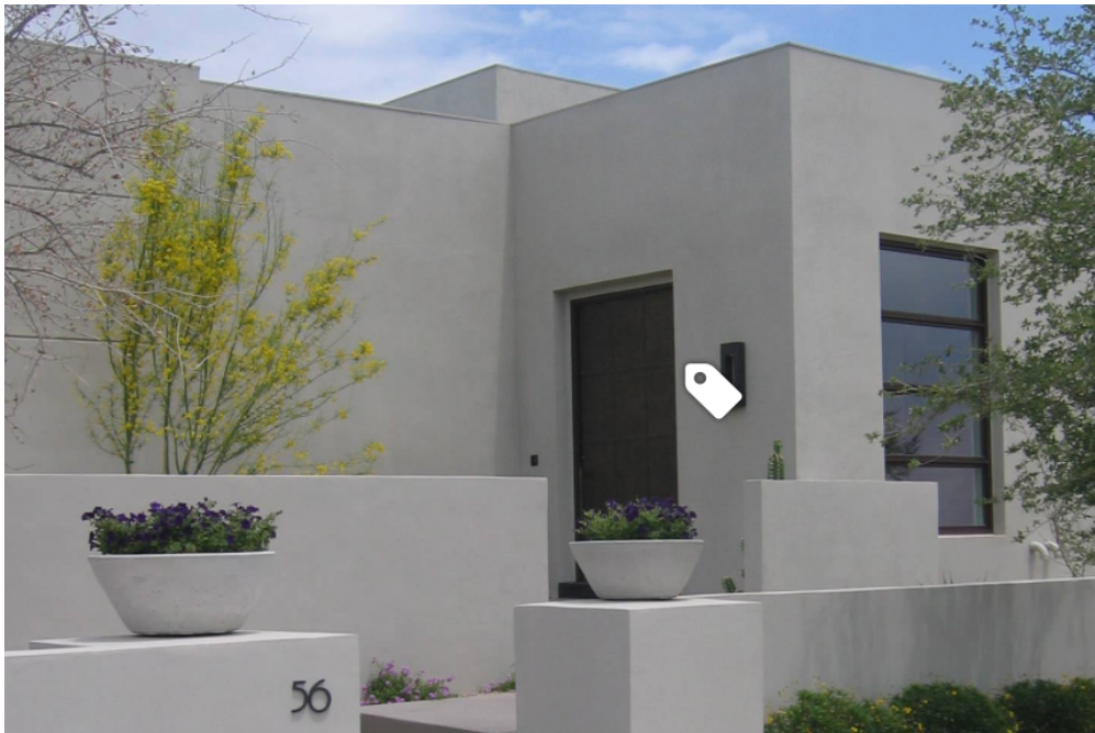
1 STUCCO WALLS PHOTO FROM HOUZZ
