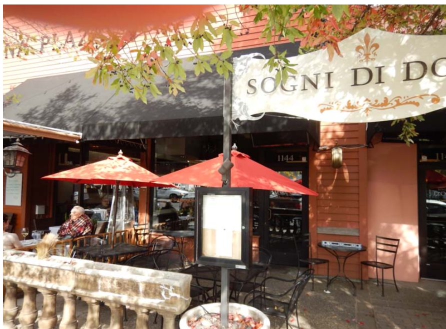
View of subject building
