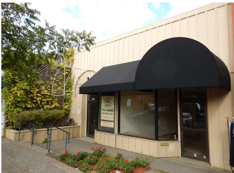
View of north end of subject building
