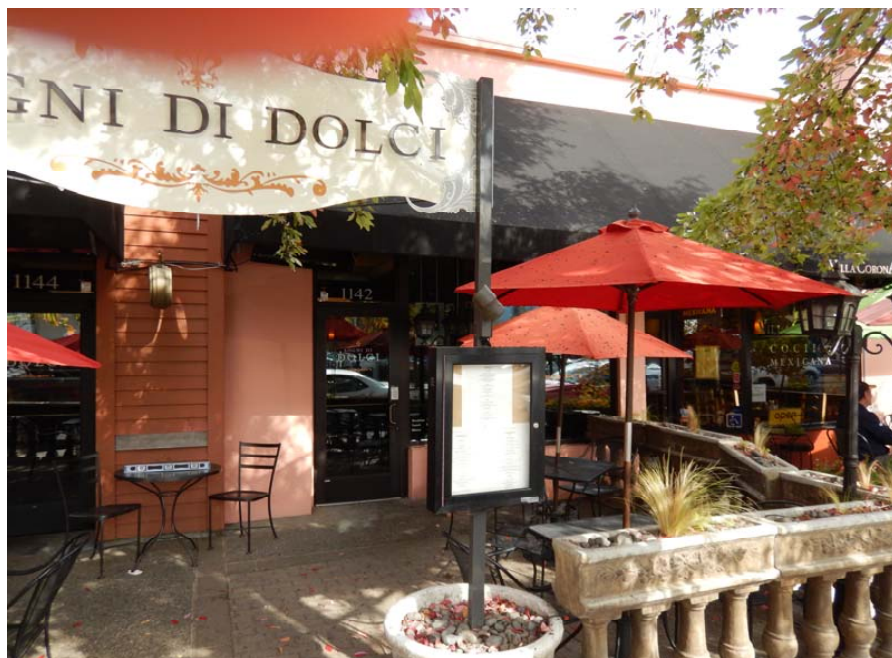
View of subject building
