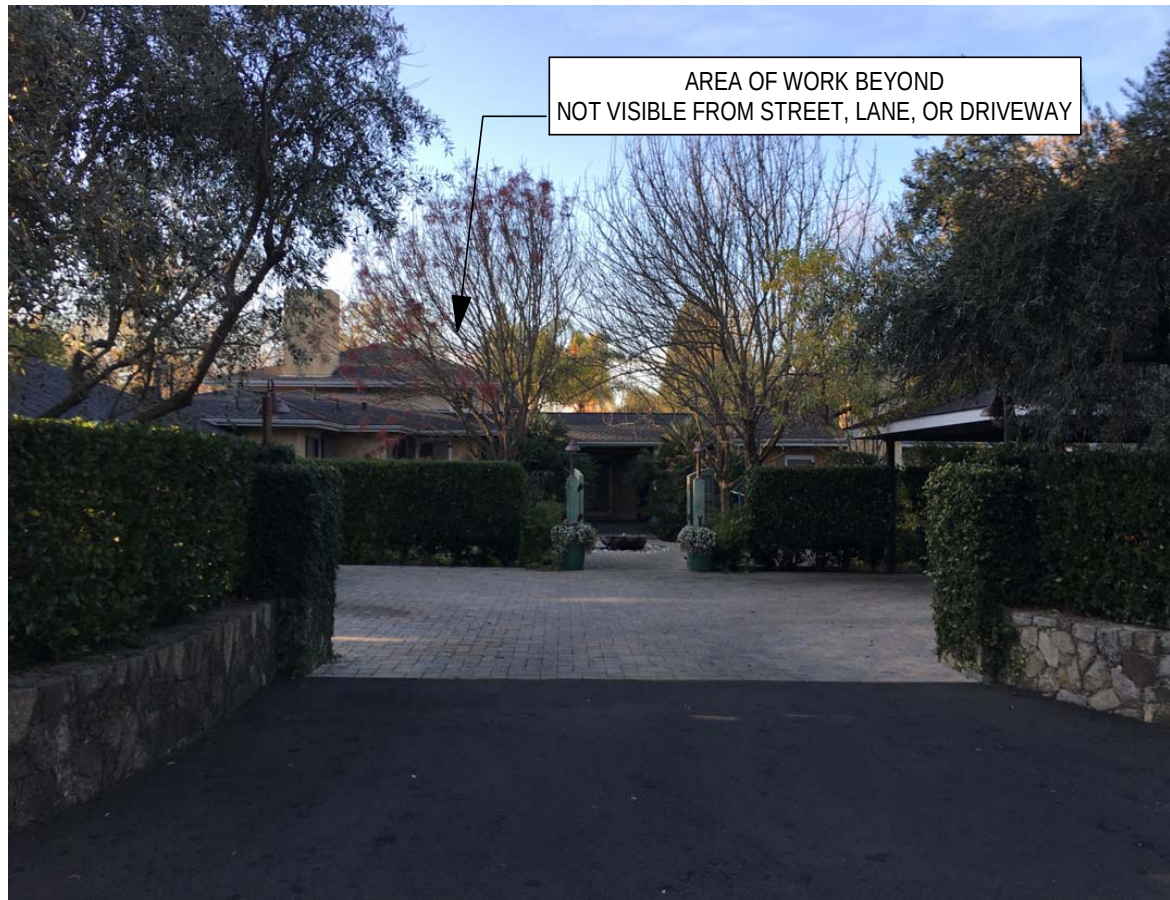
A VIEW FROM DRIVEWAY TOWARD CLOSET ADDITION BEYOND
