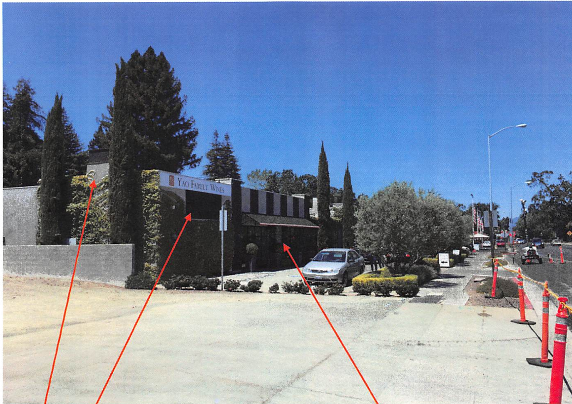
View of Building from South
