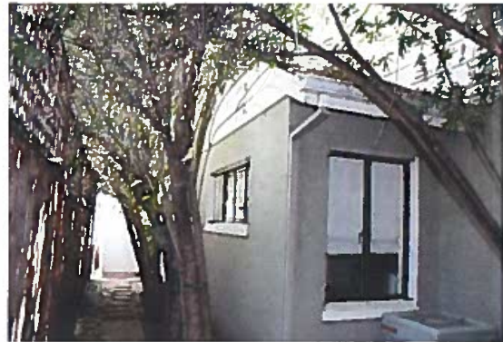
Photograph 9: Northwest elevation, camera facing east, May 11, 2018.
