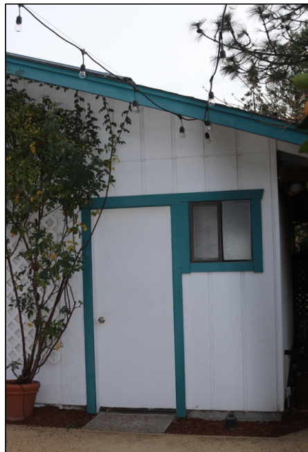
Figure 29: West elevation, pedestrian door at southwest corner
