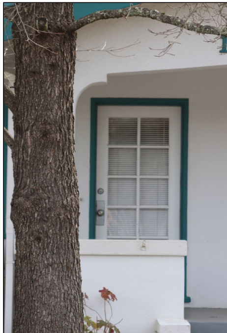
Figure 2: West elevation, front door
