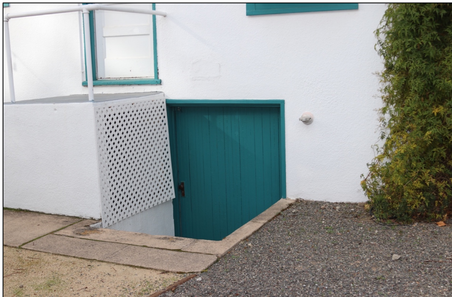
Figure 19: East elevation, door to basement
