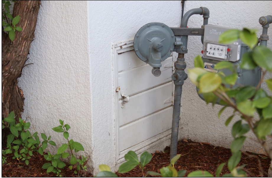
Figure 11: North elevation, hatch to crawl space
