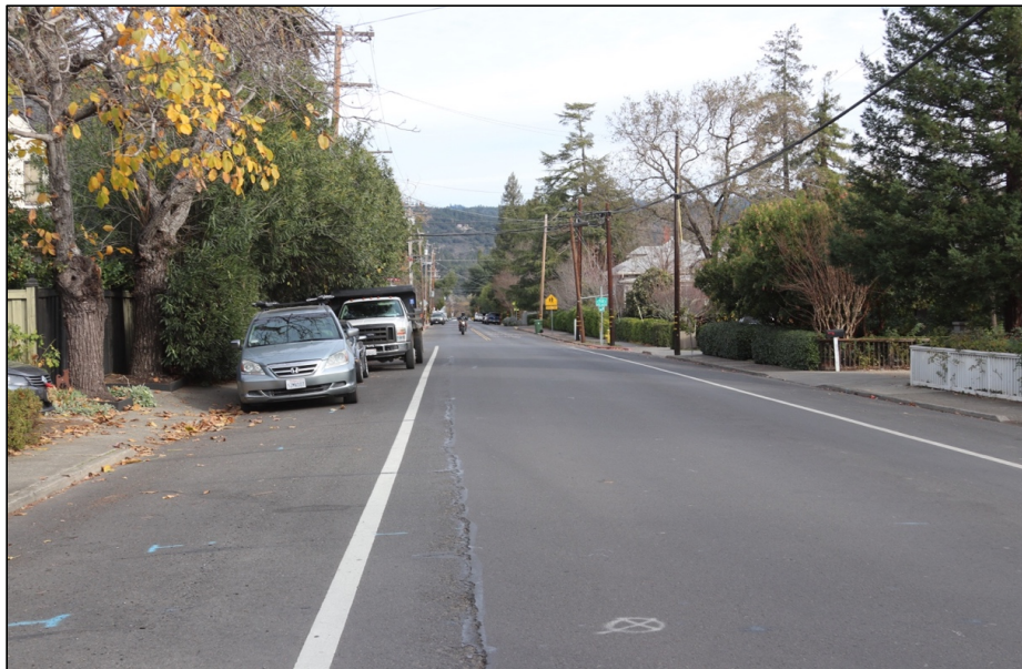
Figure 45: Madrona Avenue looking south
