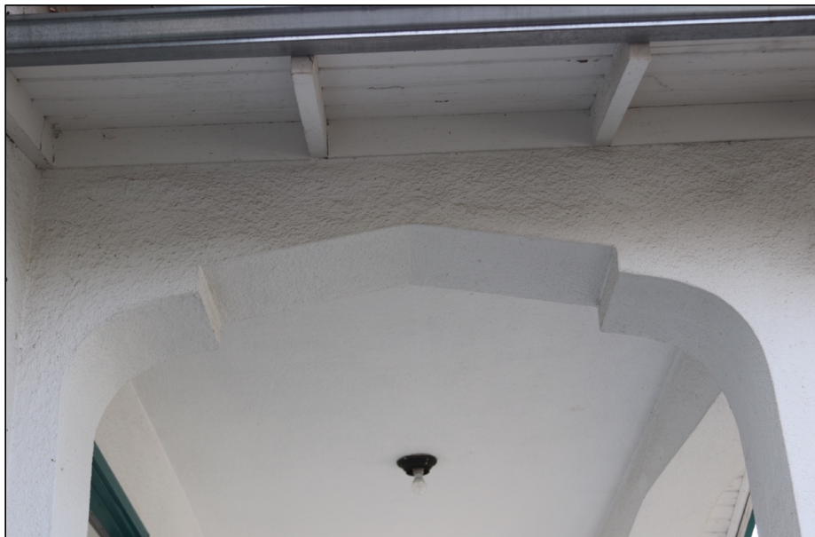
Figure 7: Detail of ogee arch on front porch
