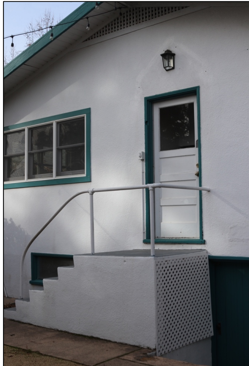
Figure 18: East elevation, back door and stoop
