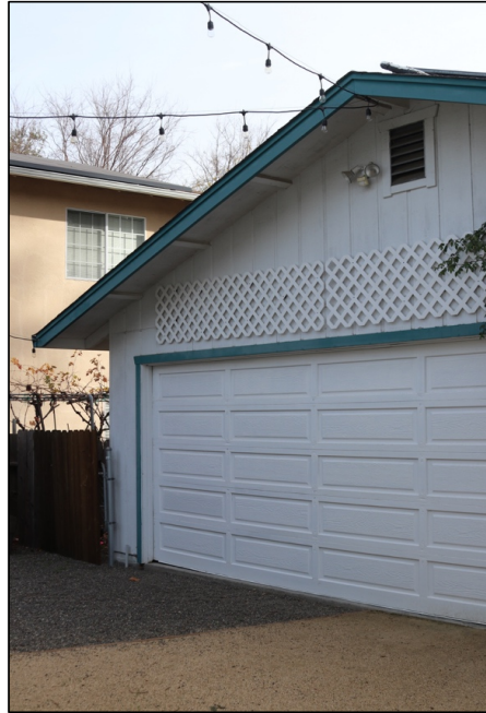
Figure 28: West elevation, northwest corner
