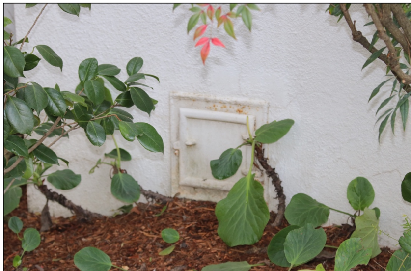
Figure 10: North elevation, ash trap at base of chimney
