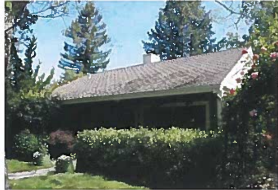
Photograph 3: Southwest (main) elevation, camera facing north, May 11, 2018.
