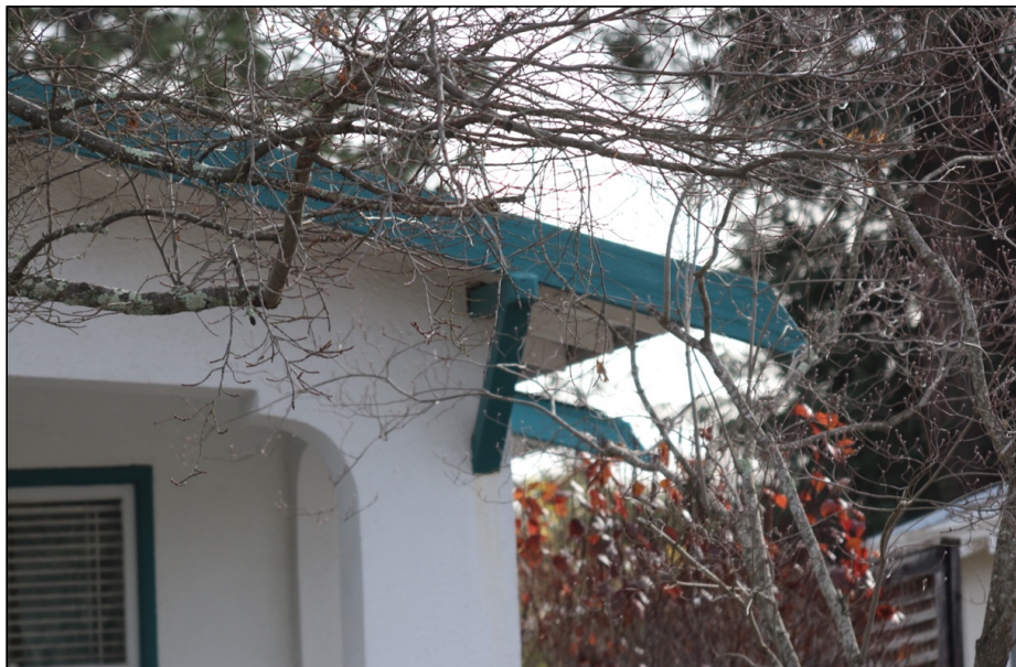
Figure 5: West elevation, eave and bracket at southwest corner
