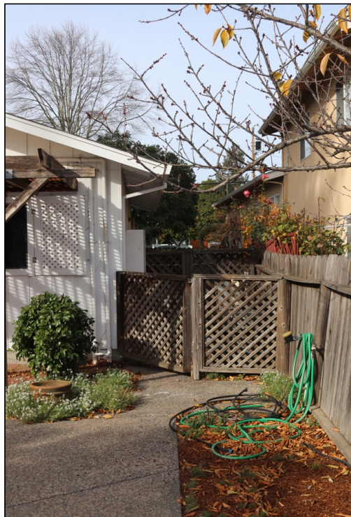
Figure 33: North elevation, pool equipment
