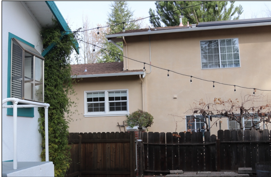
Figure 36: Wood board fence on north side of rear yard, looking north toward 1553 Madrona Ave.
