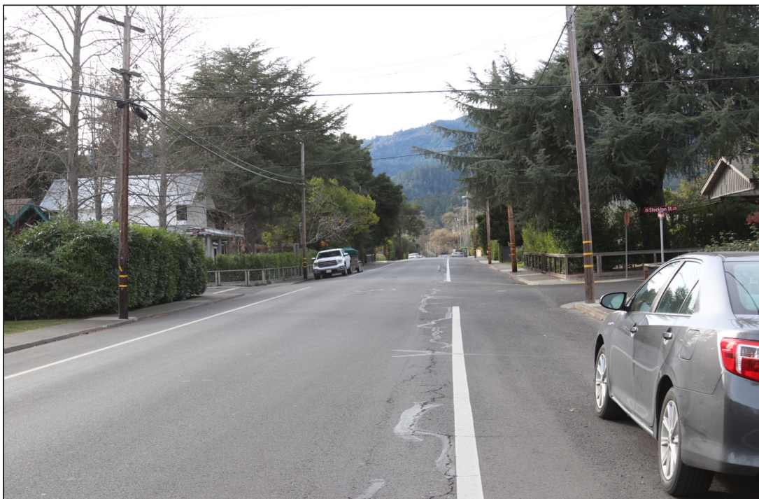
Figure 46: Madrona Avenue looking north
