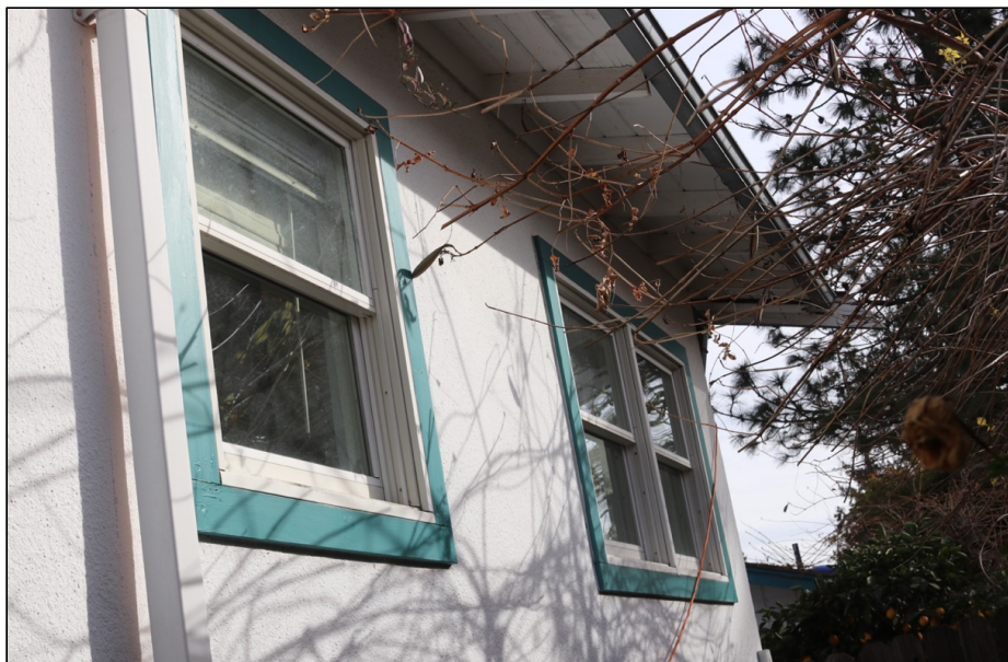
Figure 26: South elevation, windows at southeast corner
