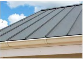
PROPOSED ROOFING: standing seam metal
