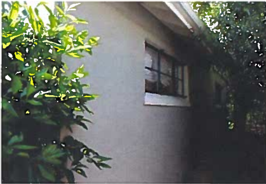
Photograph 8: Northwest elevation, camera facing south, May 11, 2018.
