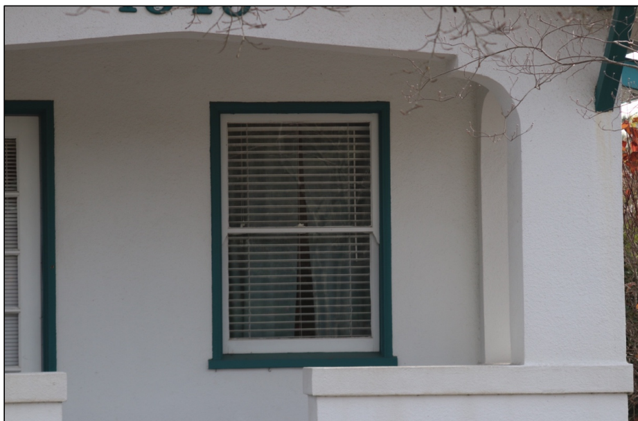
Figure 3: West elevation, window at southwest corner
