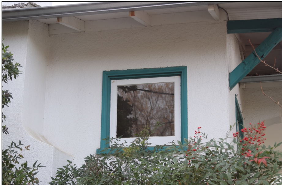
Figure 12: North elevation, square window at northwest corner
