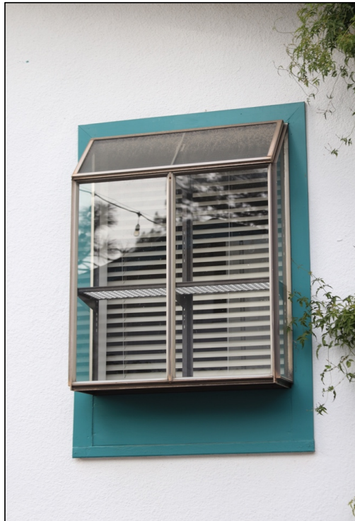
Figure 22: East elevation, northeast window
