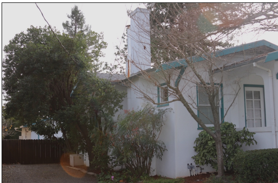
Figure 8: Northwest corner, chimney on north elevation
