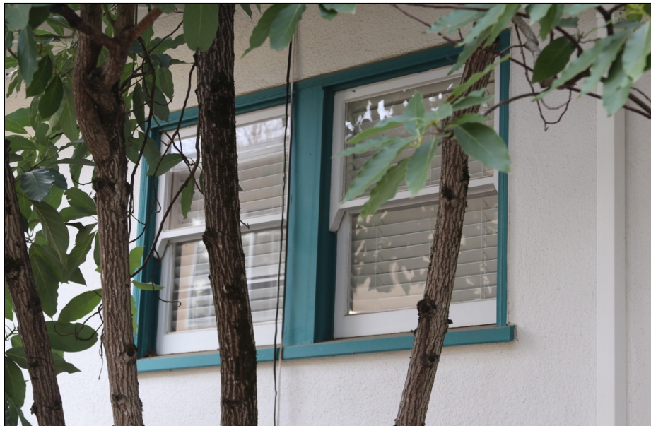
Figure 16: North elevation, windows at northeast corner
