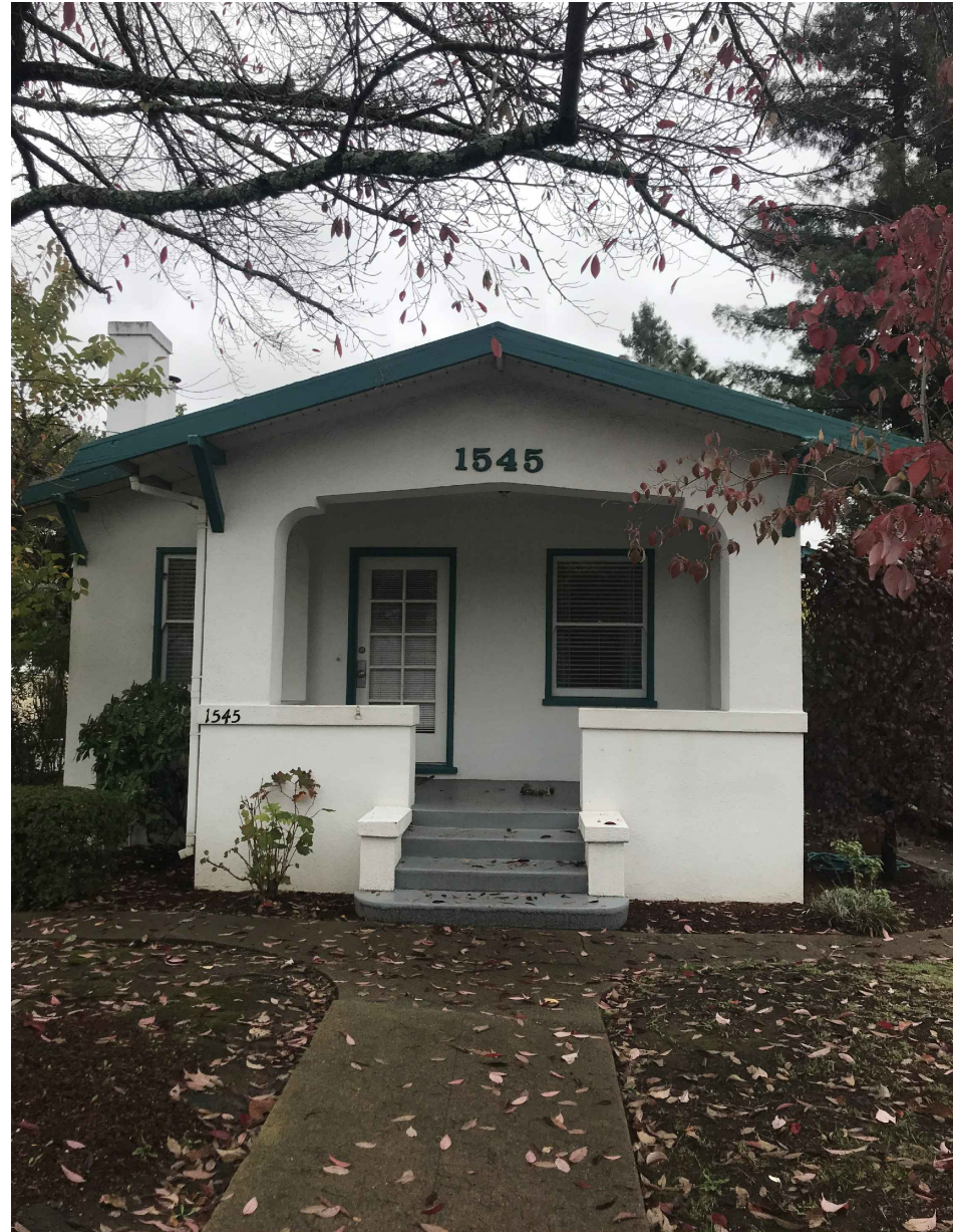
1 Existing Front View
