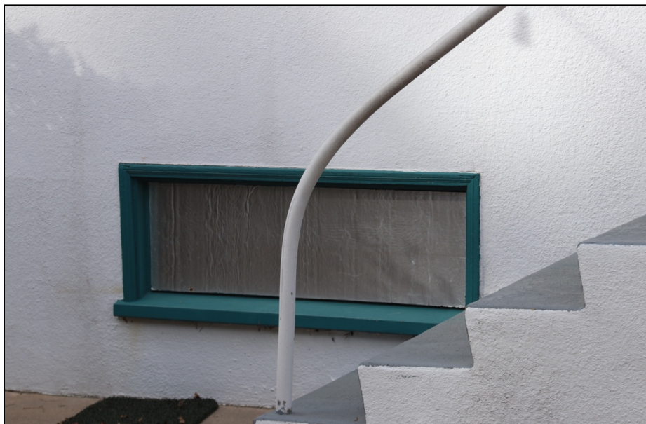
Figure 20: East elevation, basement window
