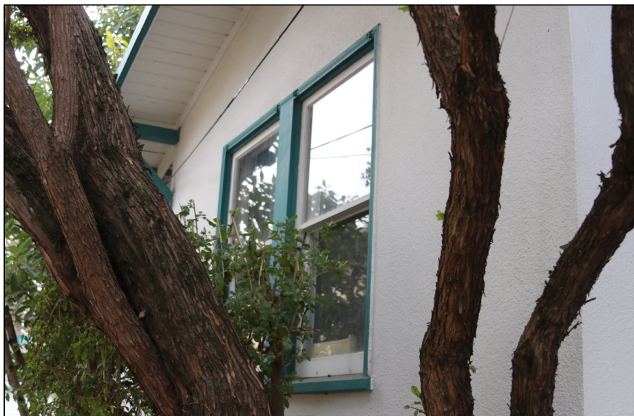
Figure 14: North elevation, pair of windows on cross gable
