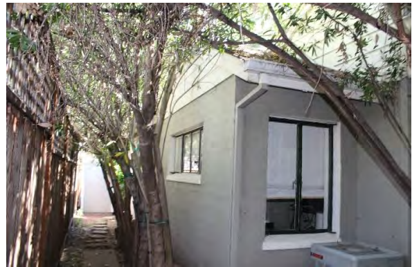
Photograph 9: Northwest elevation, camera facing east, May 11, 2018.
