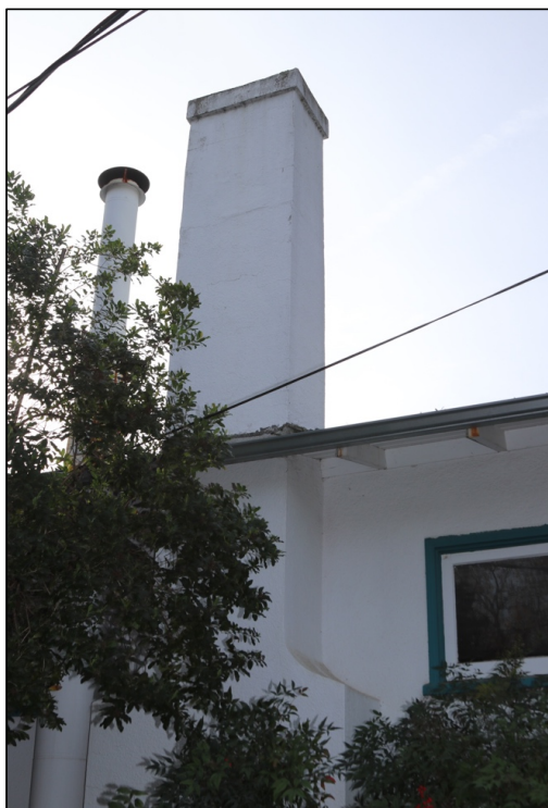
Figure 9: North elevation, chimney
