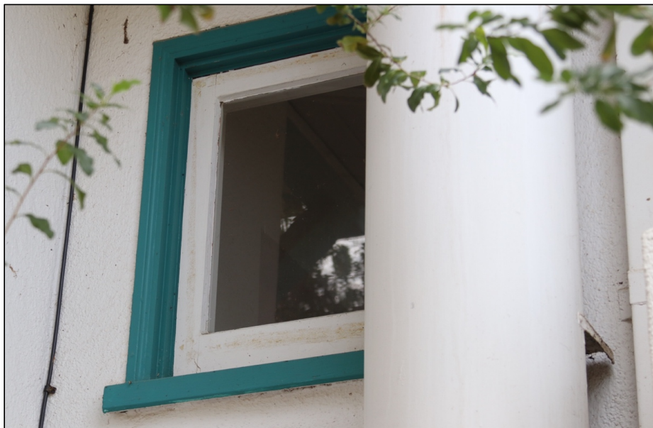
Figure 13: North elevation, square window east of chimney
