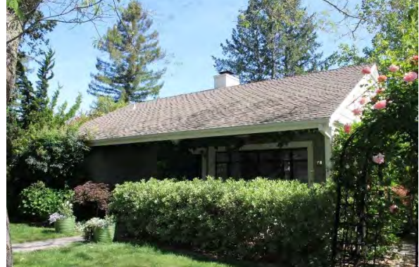
Photograph 3: Southwest (main) elevation, camera facing north, May 11, 2018.
