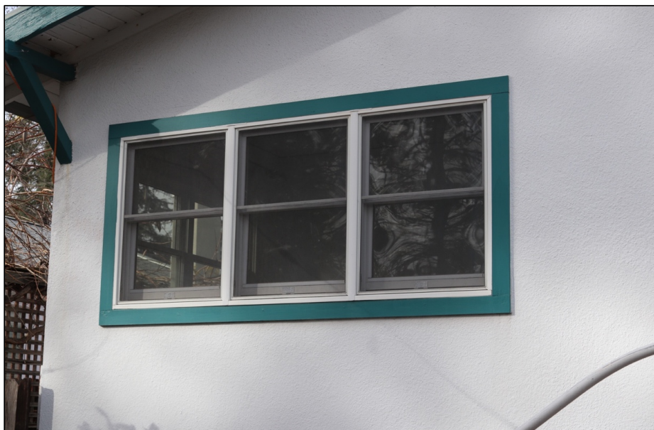
Figure 23: East elevation, southeast band of windows
