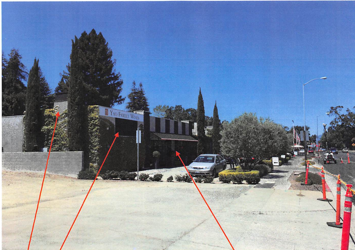
View of Building from South
