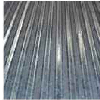
GALVANIZED CORRUGATED METAL ROOFING
