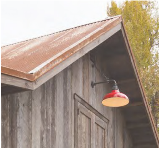
Corrugated Metal Roof
