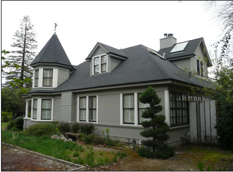
Photo showing the northwest elevation (center) and southwest elevation (right), facing east.
