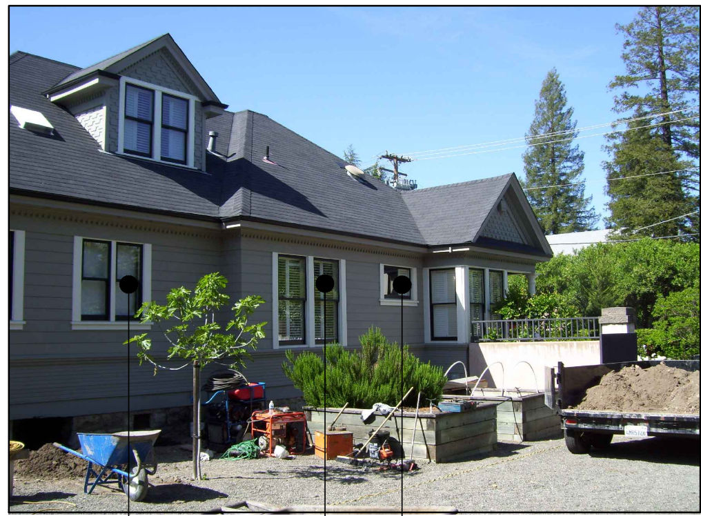
EXISTING WINDOWS TO BE REPLACED
