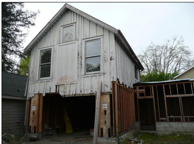
Figure 5. Photo showing the northeast elevation of the converted barn (center) with attached wing (far right).
