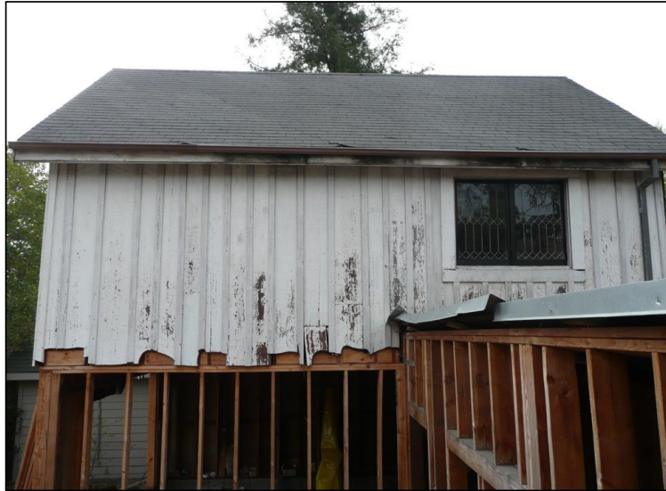
Figure 6. Photo showing the northwest elevation of the converted barn, with attached wing visible (bottom-left).
