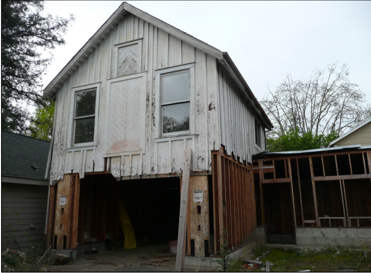
Photo showing the northeast elevation of the converted barn (center) with attached wing (far right).
