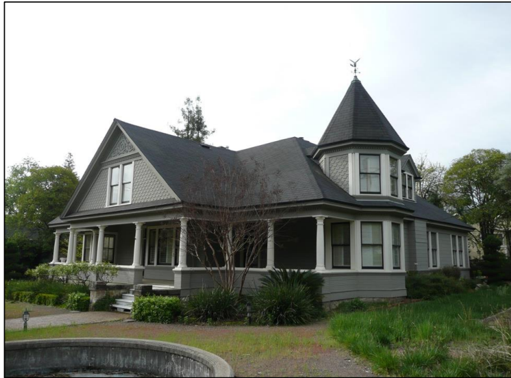
Figure 2. Photo showing the primary, northeast elevation (left) and secondary, northwest elevation, facing south.
