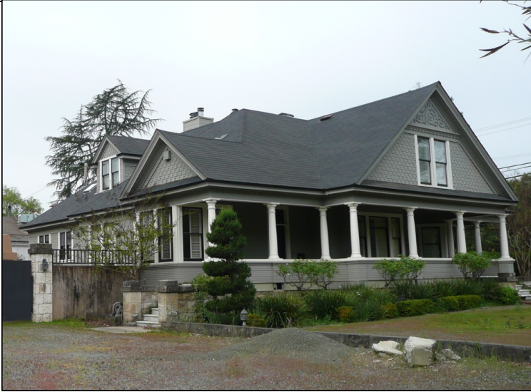
Photo showing the secondary, southeast elevation (left) and primary, northeast elevation (right), facing west.
