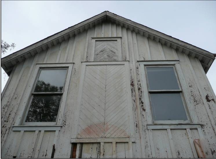
Photo showing detail of second-floor northeast elevation of converted barn.
