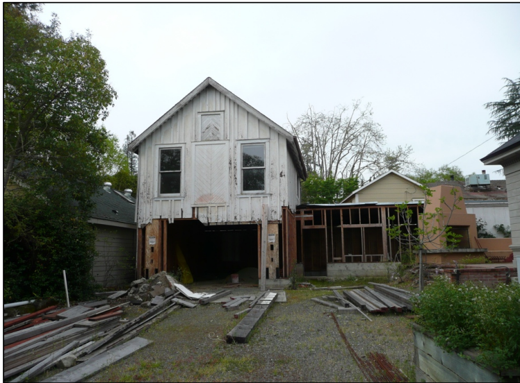
Photo showing the northeast elevation of the converted barn (center) with attached wing (right).
