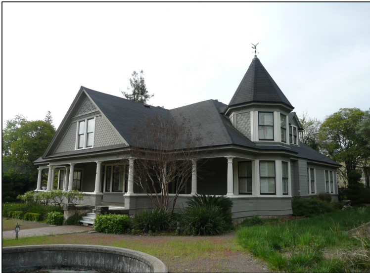
Photo showing the primary, northeast elevation (left) and secondary, northwest elevation, facing south.
