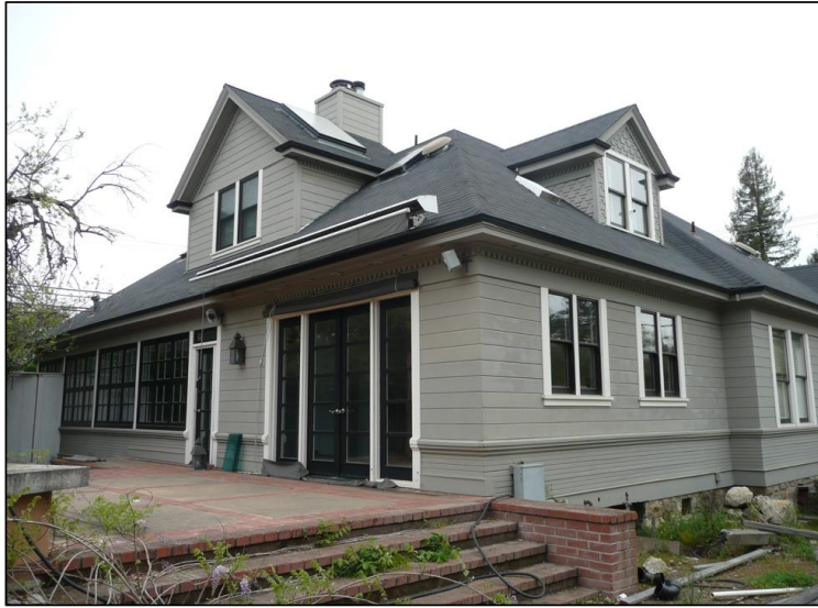
Figure 4. Photo showing the southwest elevation with contemporary gabled dormer and altered sunporch (left) and southeast elevation (right), facing north.
