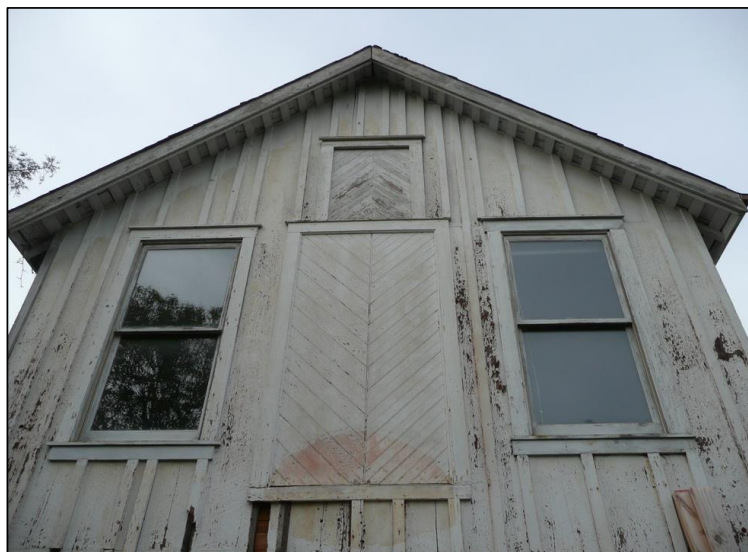
Figure 7. Photo showing detail of second-floor northeast elevation of converted barn.
