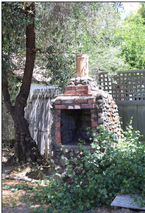
Figure 36: Brick and stone fireplace in north yard
