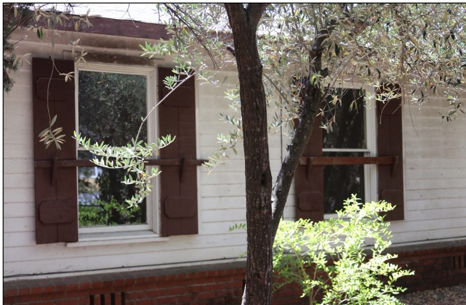
Figure 24: West (front) elevation, new house, windows south of door
