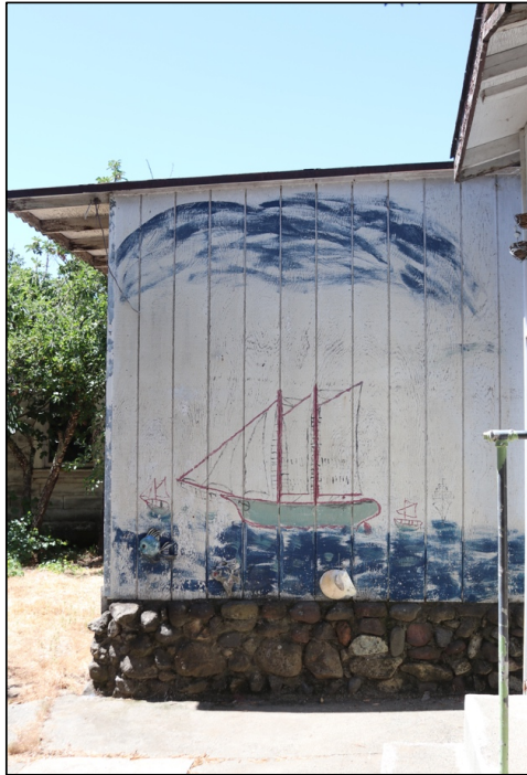
Figure 29: New house, north side of addition on rear
