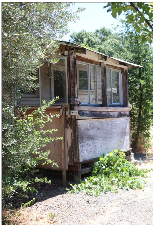
Figure 6: South elevation, original house, covered porch
