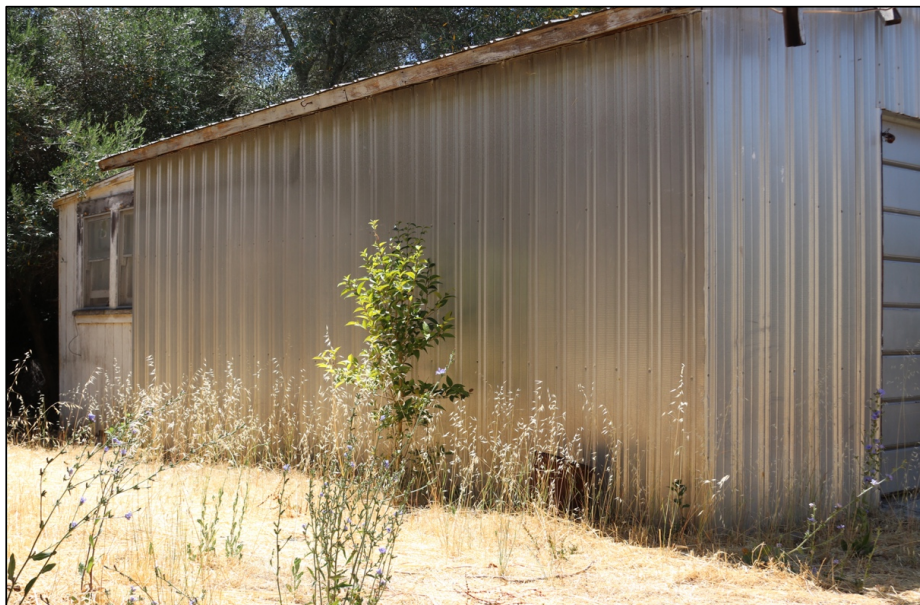
Figure 34: Garage, north side
