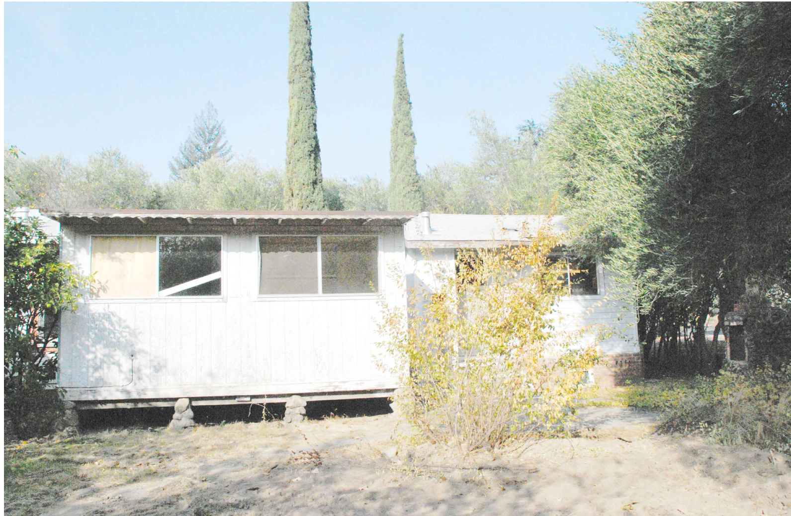
Rear of Residence 1 (east)
