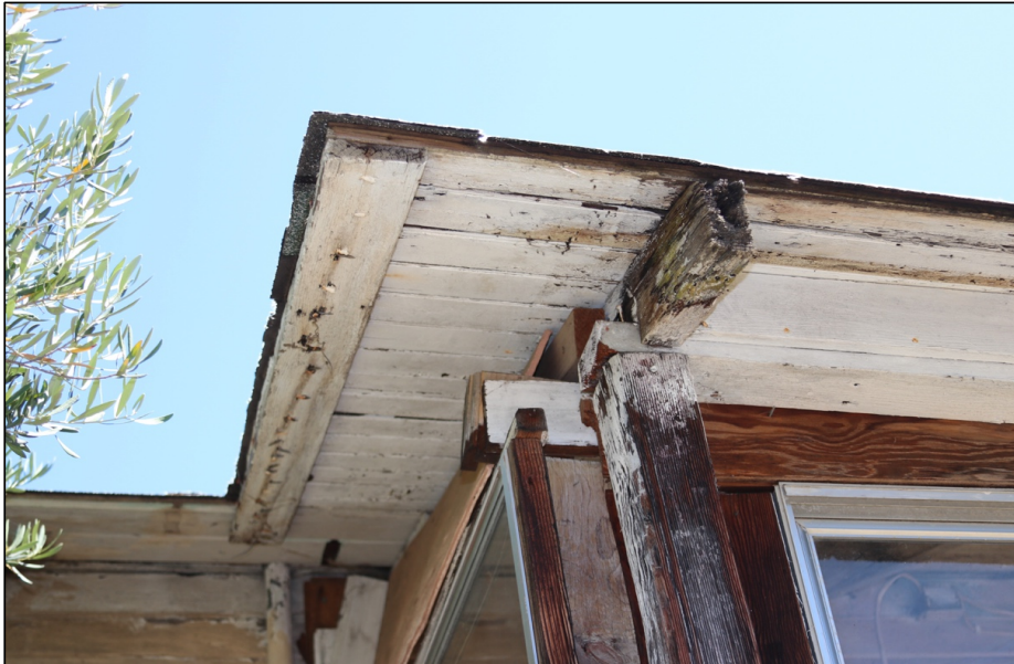
Figure 7: South elevation, original house, porch eaves
