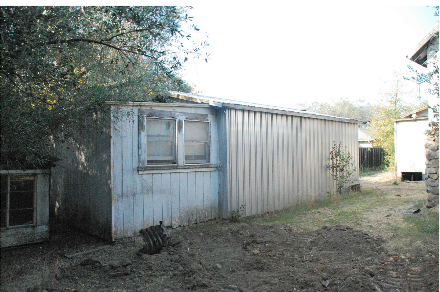
Side of of Garage (northeast)
