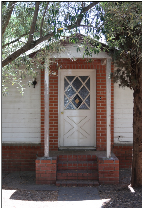
Figure 20: West elevation (front), new house, front door
