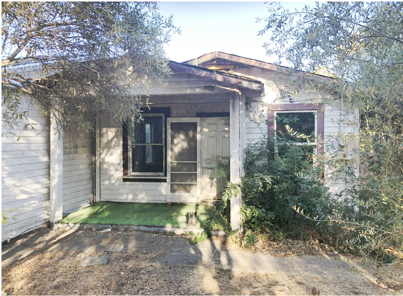
Front of Residence 2 (west)
