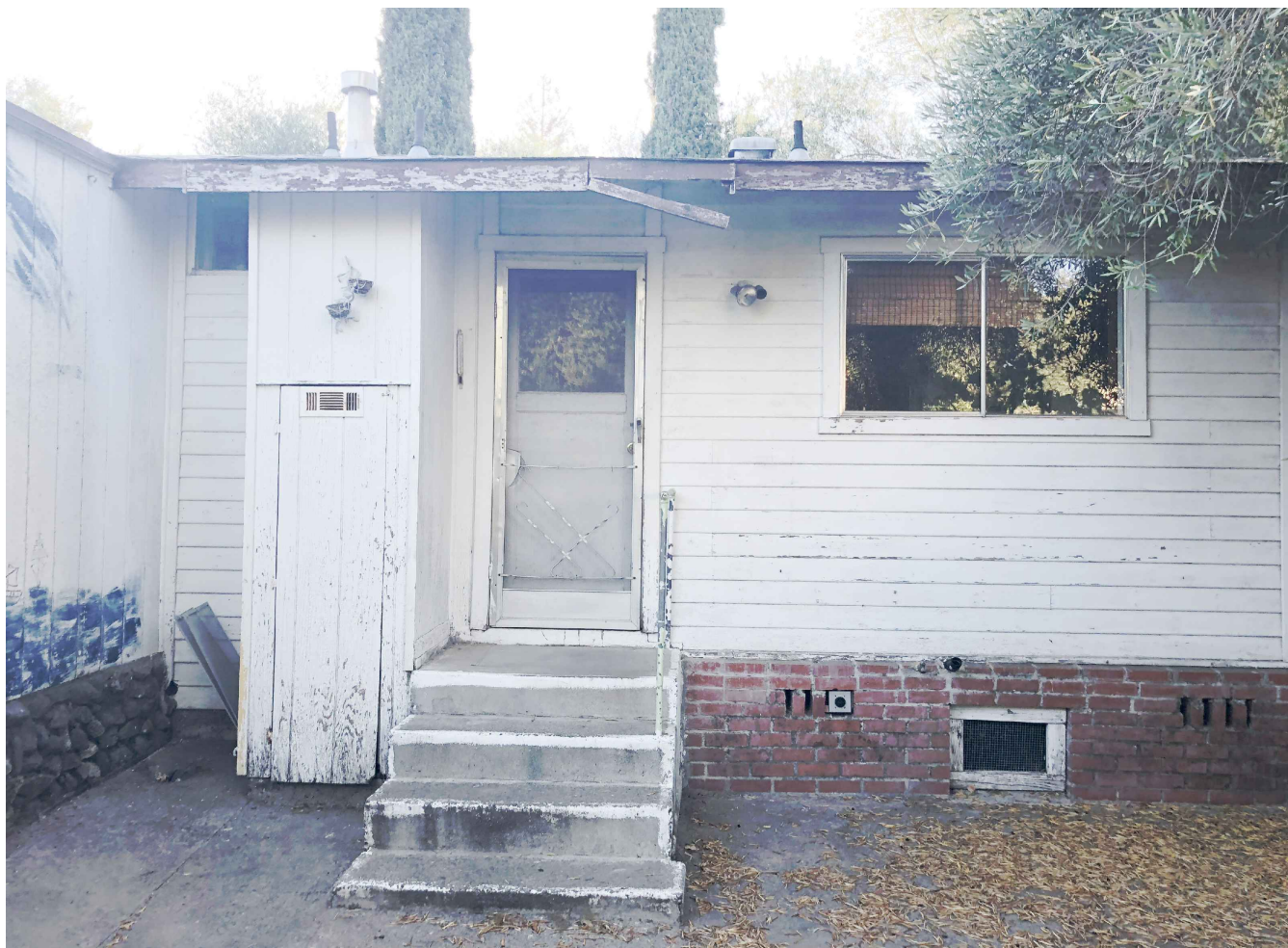
Rear of Residence 1 (east)
