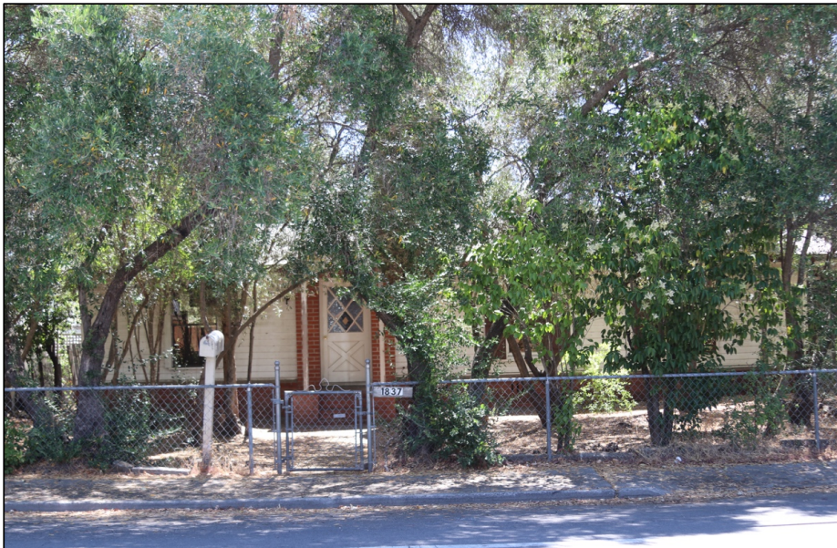
Figure 18: West (front) elevation, new house
