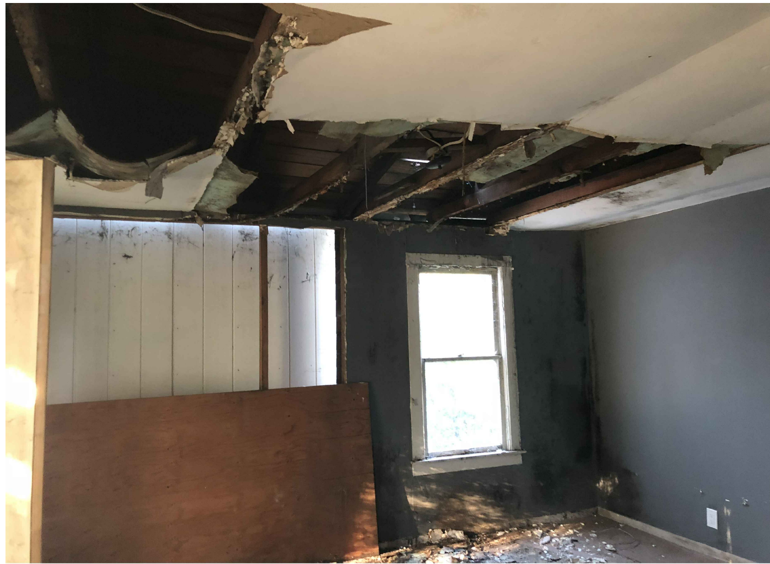
Condition of Structures
