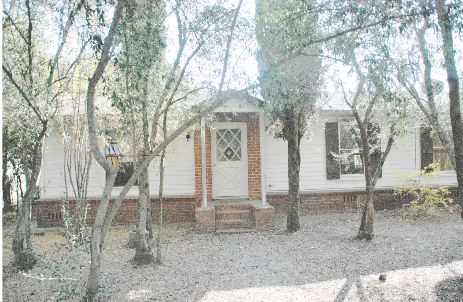
Front of Residence 1 (West)
