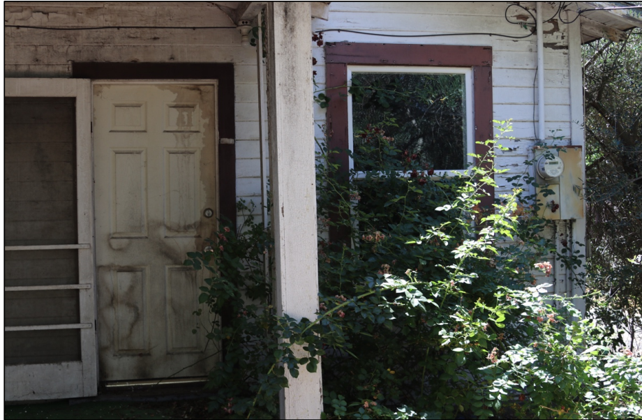
Figure 3: West elevation (front), original house, front door and window to the south
