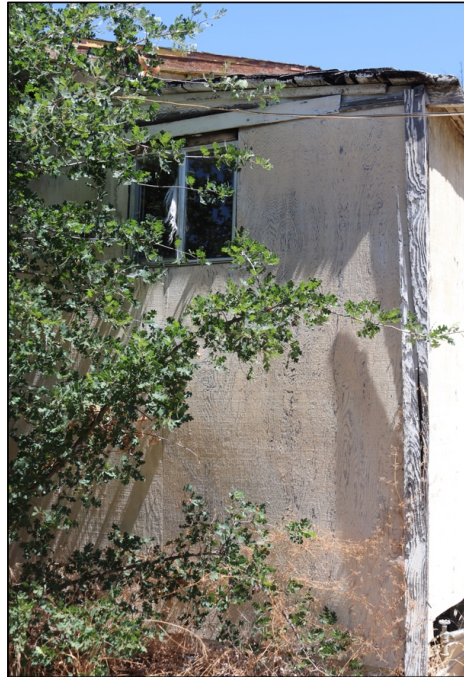
Figure 9: South elevation, original house, shed addition
