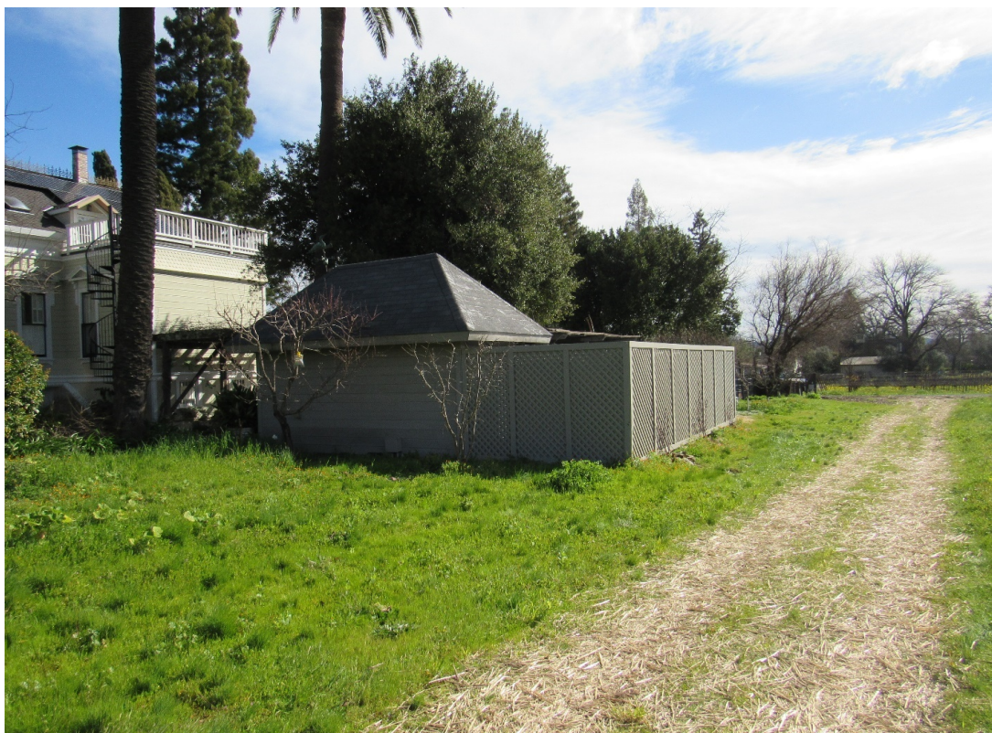
SOUTHWESTERN VIEW OF EXISTING SHED WITH LATTICE SCREENING AROUND WATER STORAGE TANKS
