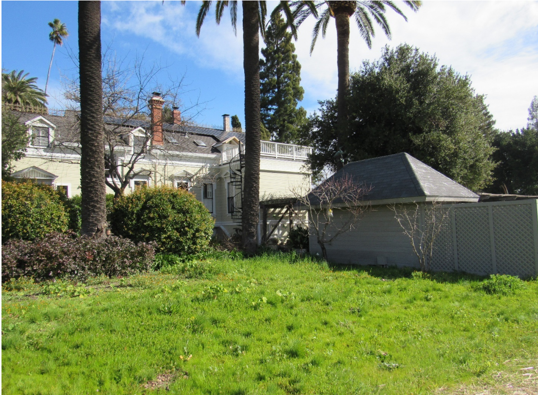
WESTERN VIEW OF EXISTING SHED WITH RESIDENCE BEYOND
