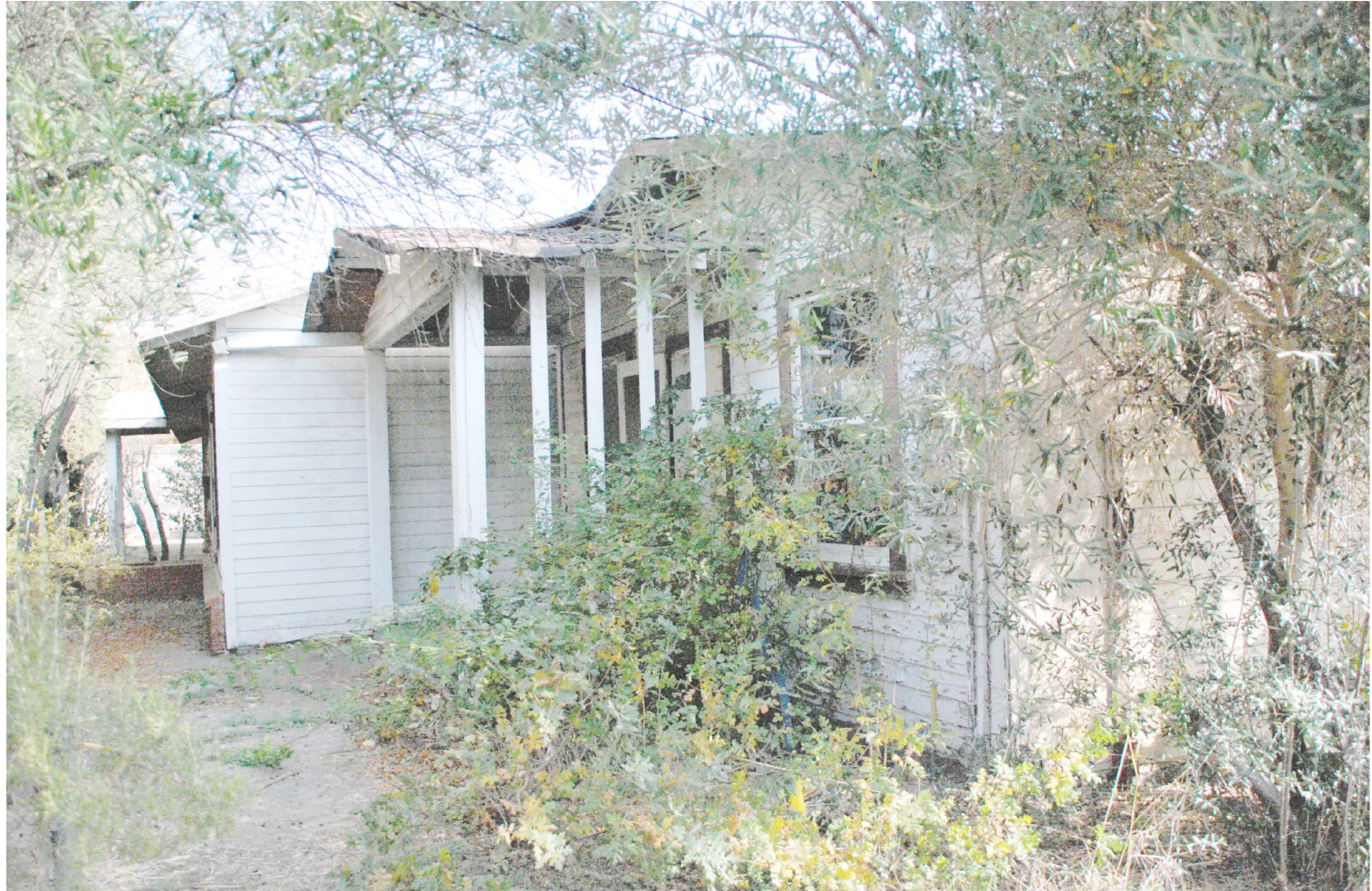
Side of Residence 2 (Southwest)
