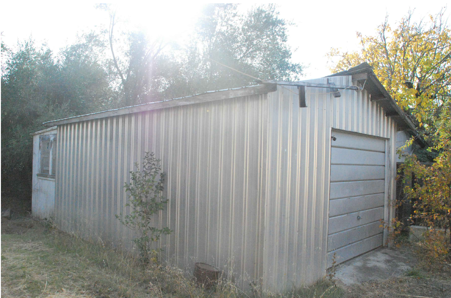
Side of Garage (northwest)
