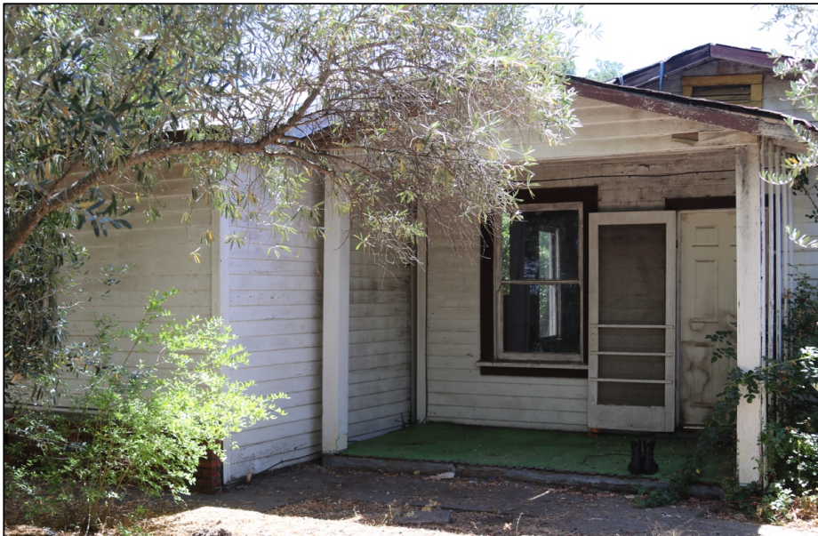
Figure 2: West elevation, junction of old house and new house
