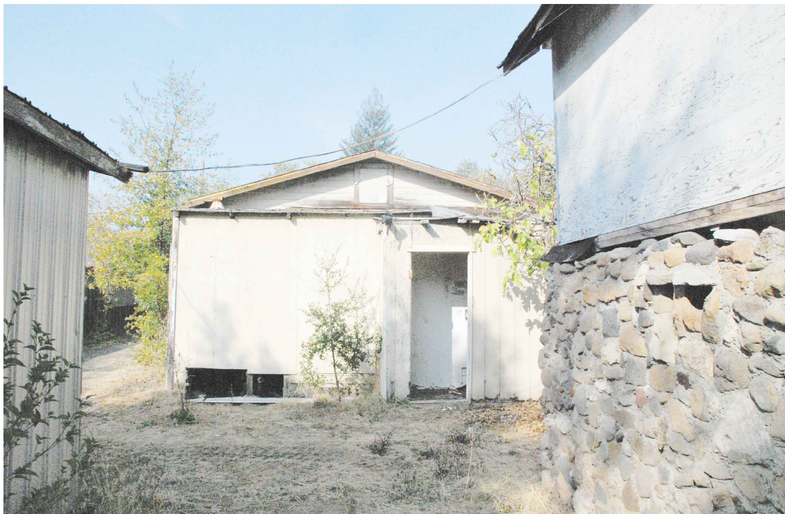
Rear of Residence 2 (east)
