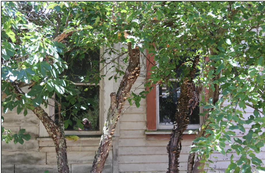
Figure 14: North elevation, original house, junction additional and main block, windows
