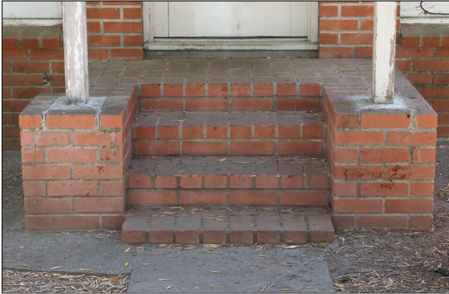
Figure 21: West (front) elevation, new house, front door stoop
