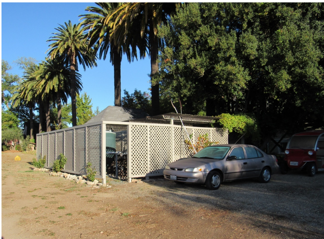
SOUTHEASTERN VIEW OF EXISTING SHED WITH LATTICE SCREENING AROUND WATER STORAGE TANKS
