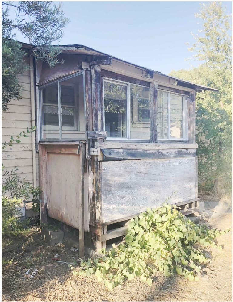
Side of Residence 2 (South)
