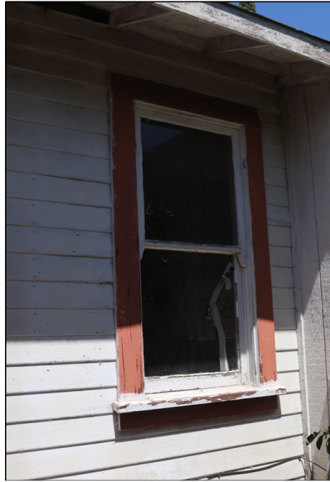
Figure 15: North elevation, original house, window
