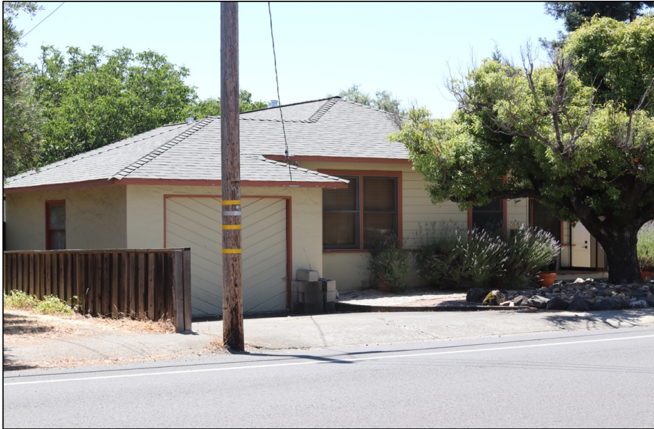
Figure 47: Neighbor to the south (1851 Madrona Ave.)
