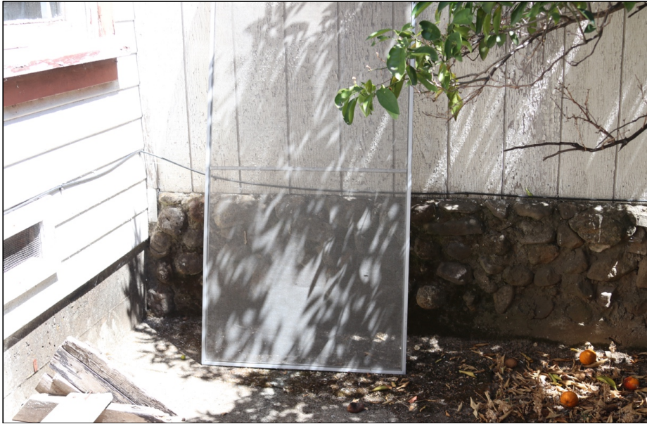
Figure 31: New house, south side of addition on rear, foundation
