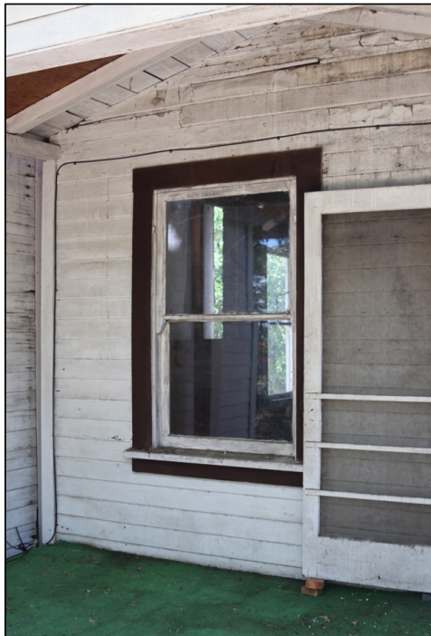
Figure 4: West elevation, original house, window north of front door
