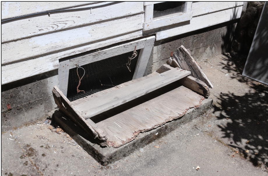
Figure 32: New house, north side, crawl space access
