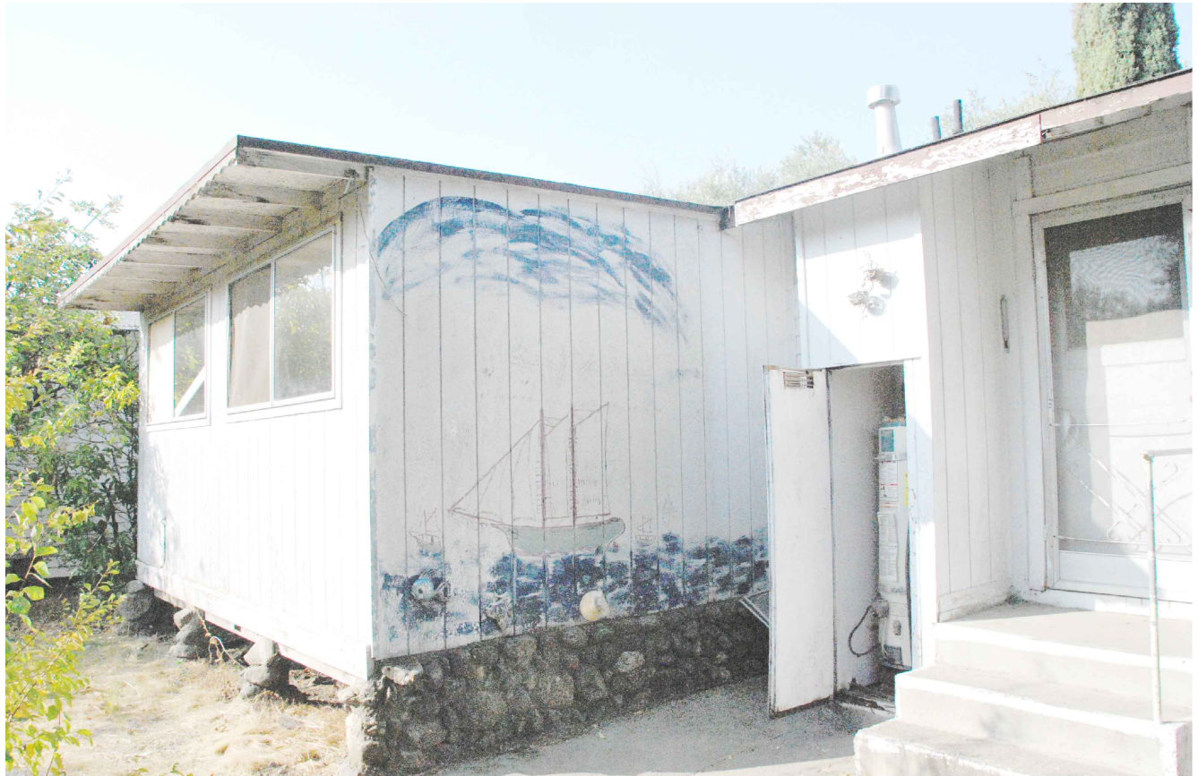
Rear of Residence 1 (northeast)
