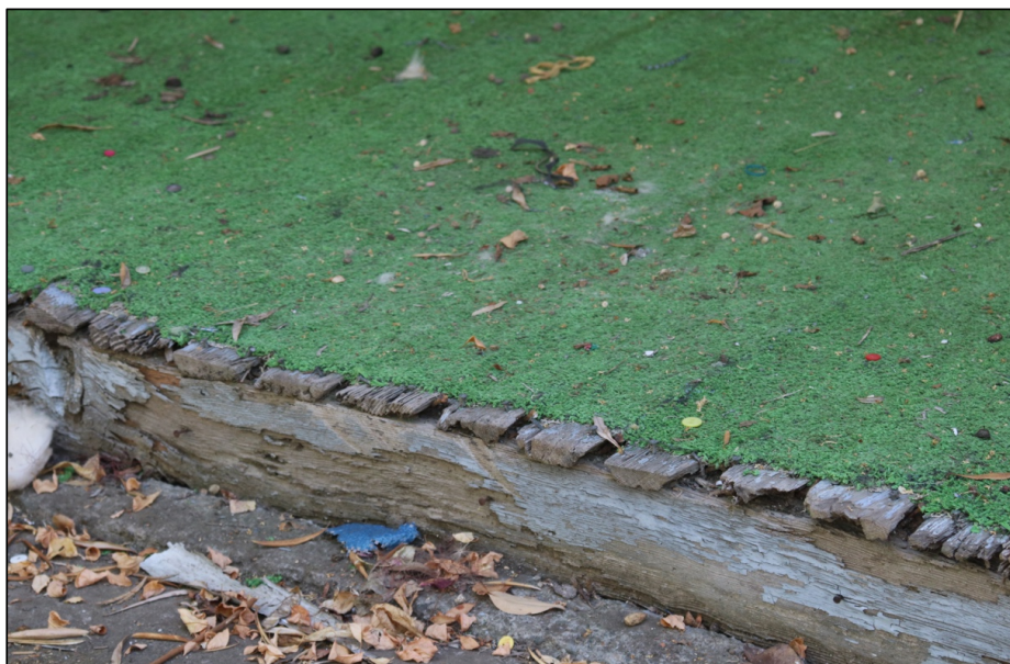
Figure 5: West elevation, original house, porch floor
