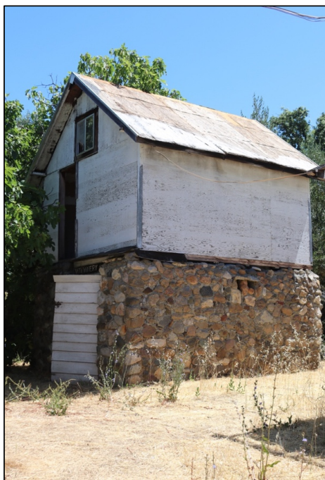
Figure 37: "Viti Winery" Building, west and south sides
