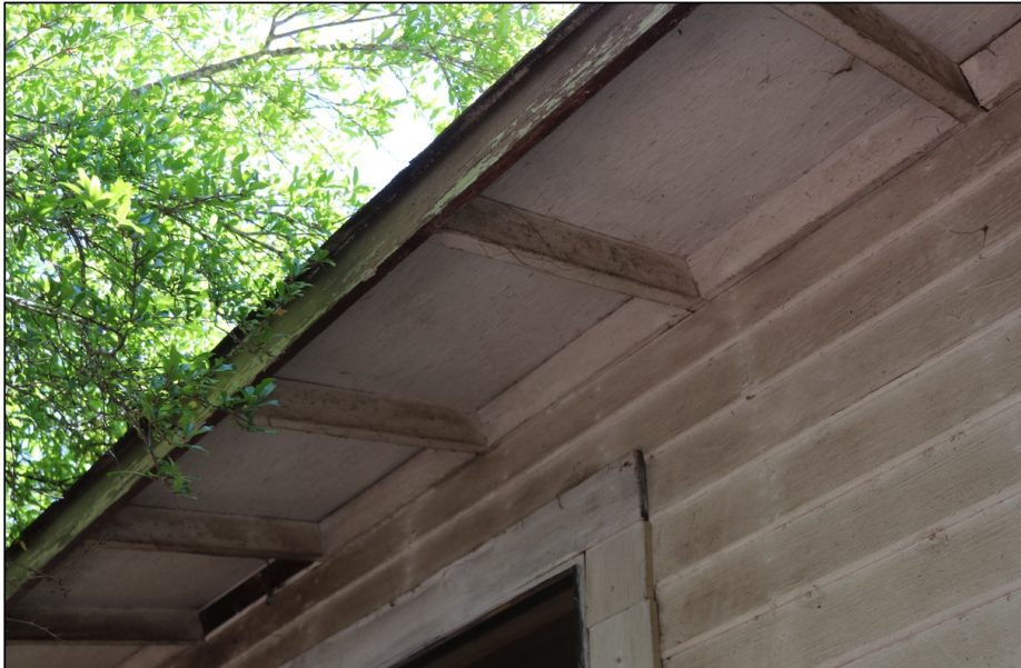
Figure 25: West (front) elevation, new house, eaves
