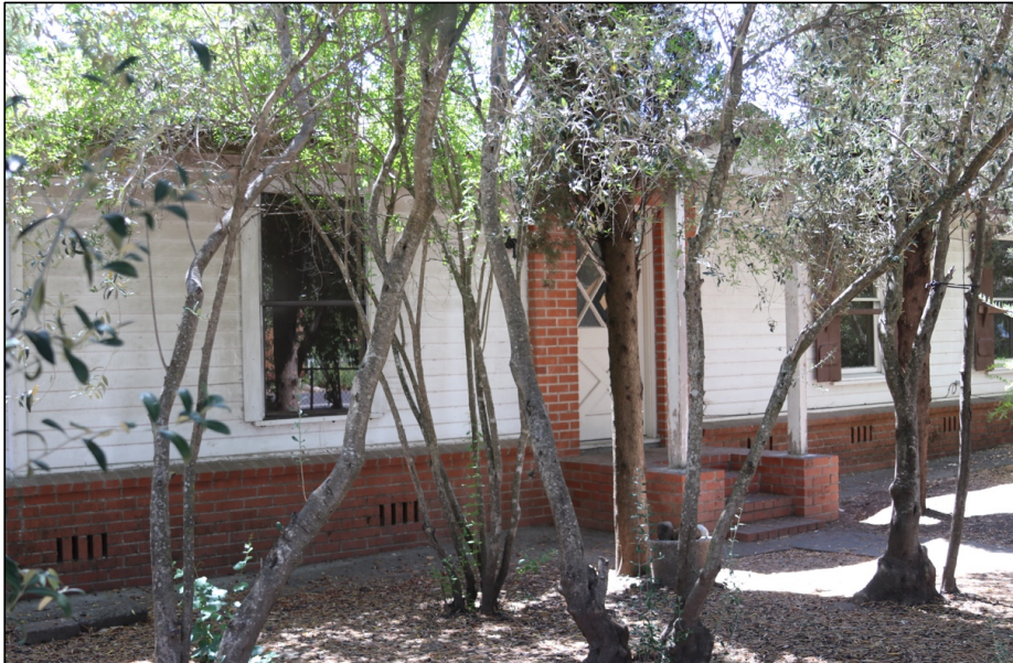
Figure 19: West (front) elevation, new house
