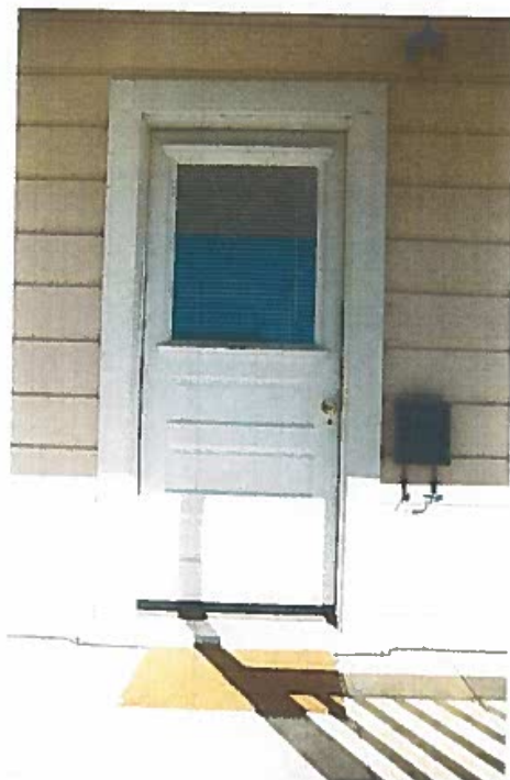
Primary Entry- South Elevation (Façade)
