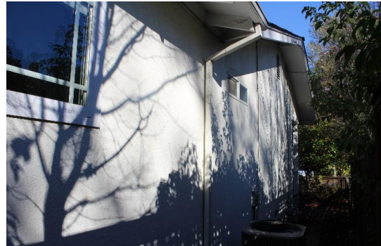
Photograph 5: East elevation, camera facing west, November 16, 2018.
