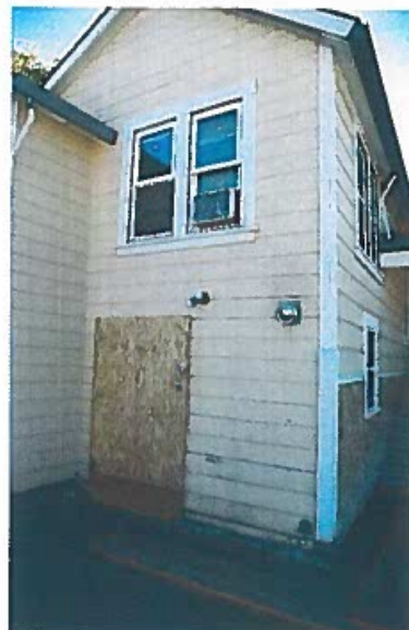
Partial Rear (north) Elevation
