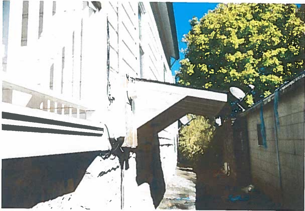
East Elevation- Looking North
