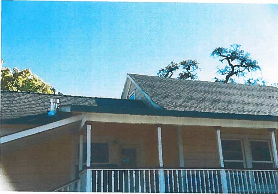
Detail of roofline- West (Side) Elevation
