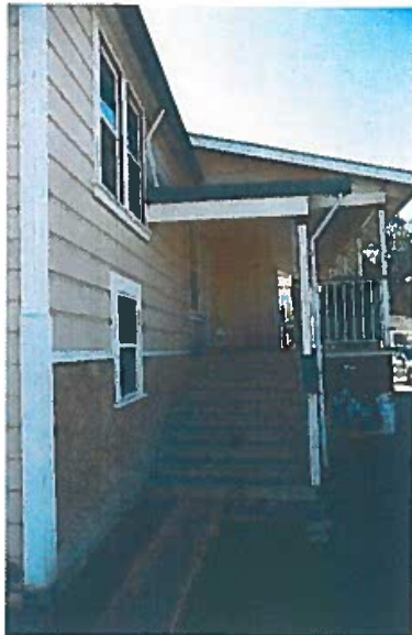
West Elevation- Looking south
