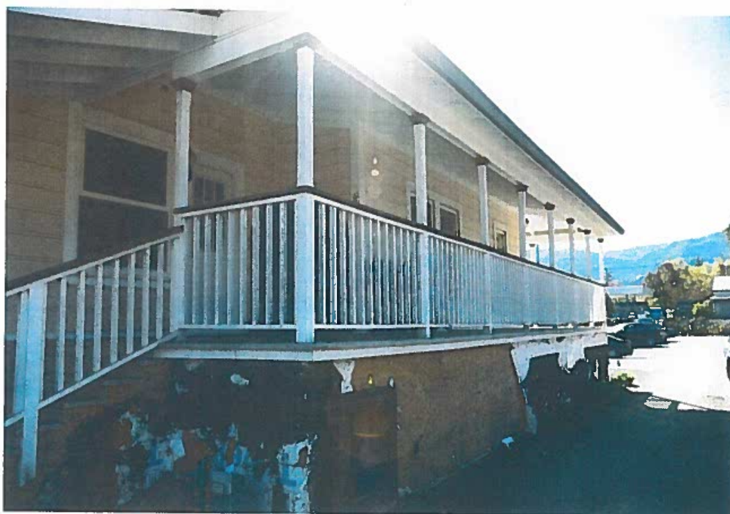
West Elevation- Looking Southeast
