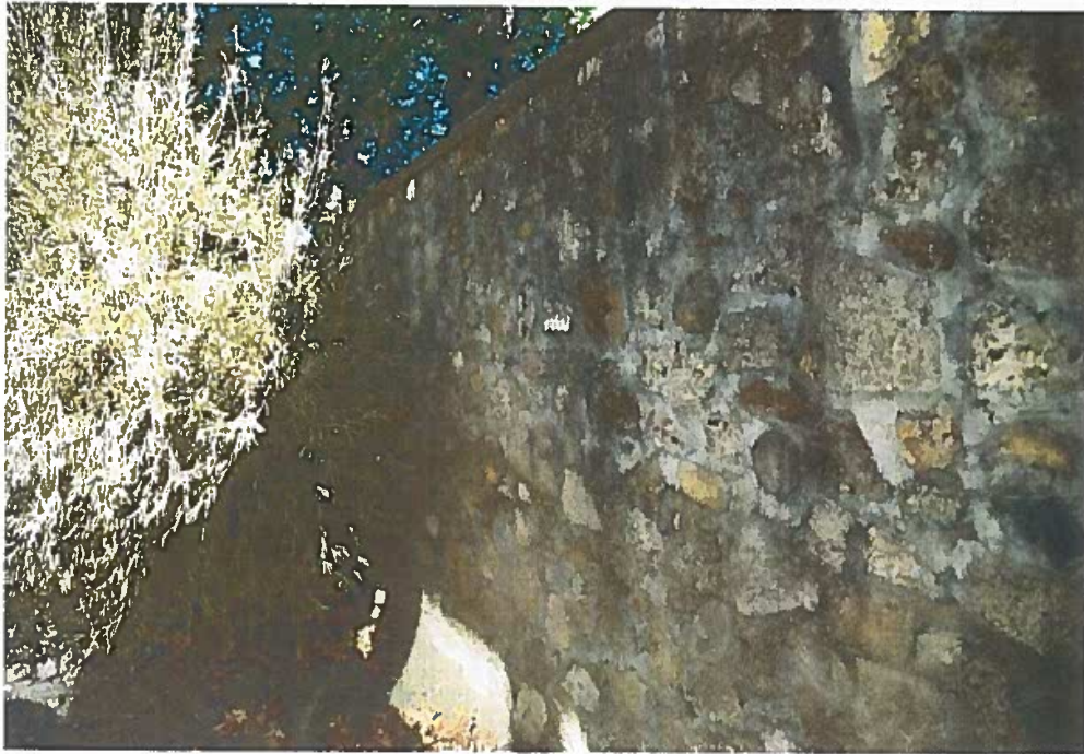
Detail of stone wall adjacent to eastern property line
