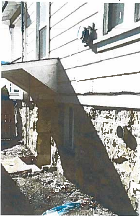
East Elevation- Looking South
