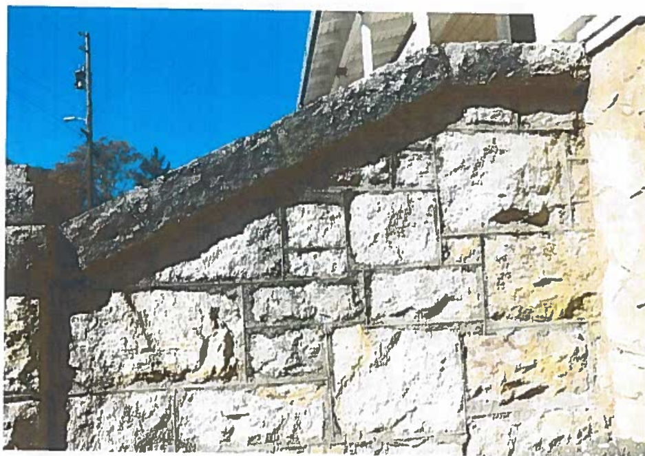
Detail of Stone Stem wall- South Elevation (Façade)
