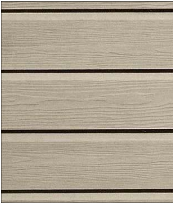
HORIZONTAL SHIP-LAP SIDING, HISTORIC PORTION, LIGHT BROWN/TAN
