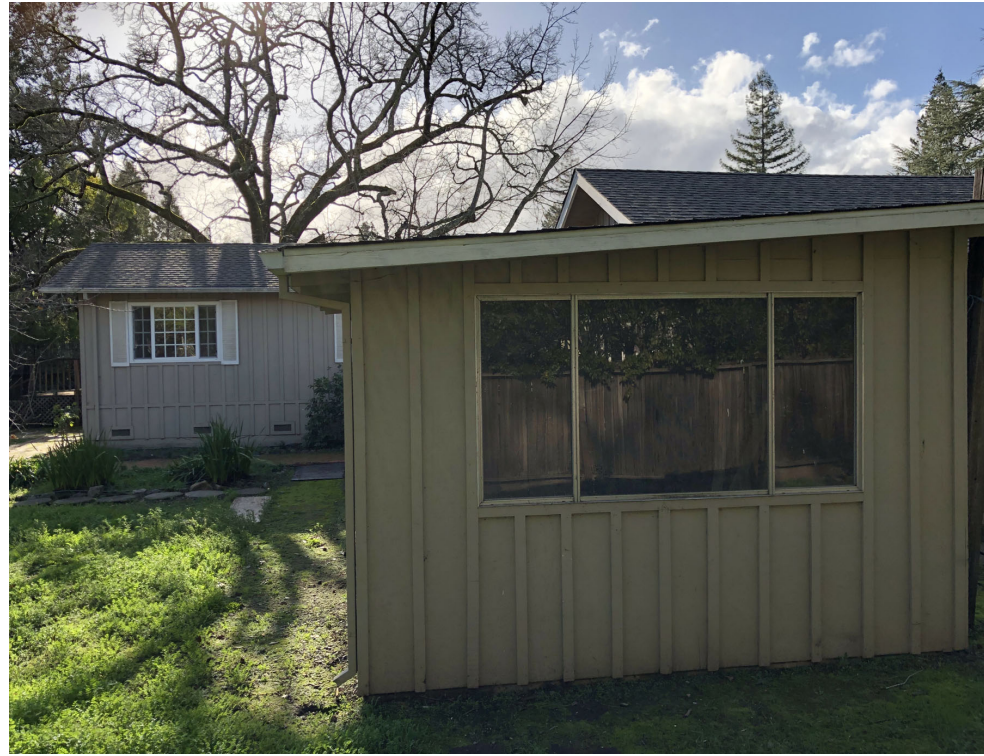
4. NORTH ELEVATION: GARAGE, MAIN RESIDENCE BEYOND (SEE PHOTO #5)
