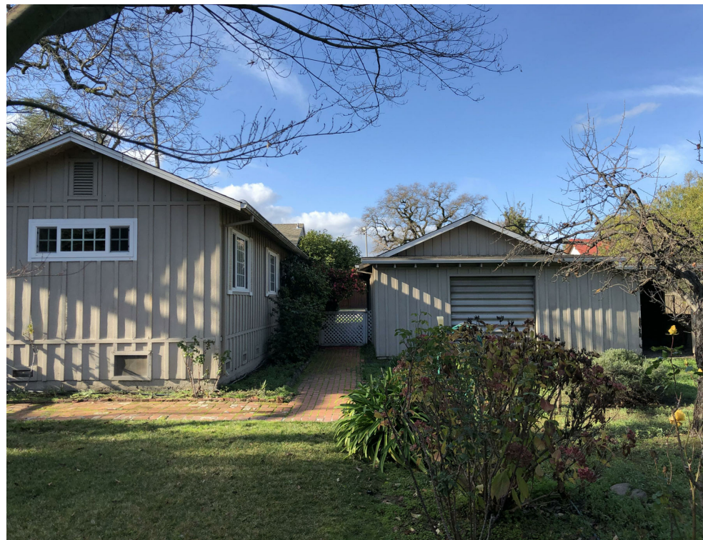
7. EAST ELEVATION: GARAGE, MAIN RESIDENCE (SEE PHOTO #8)
