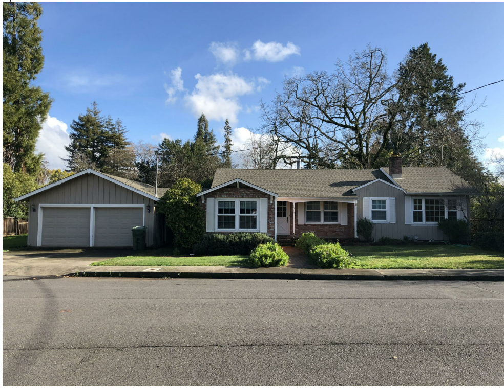
2. FRONT ELEVATION - EXISTING RESIDENCE ON PROJECT SITE 1515 PINE ST.
