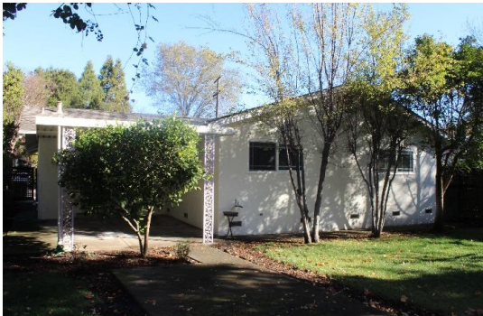
Photograph 6: South elevation, camera facing northeast, November 16, 2018.
