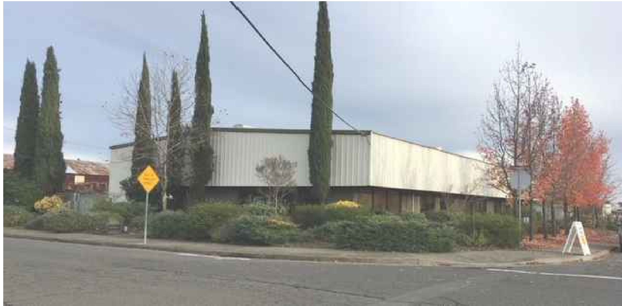
EXISTING SITE PHOTOS - WEST SCALE: NTS 4
