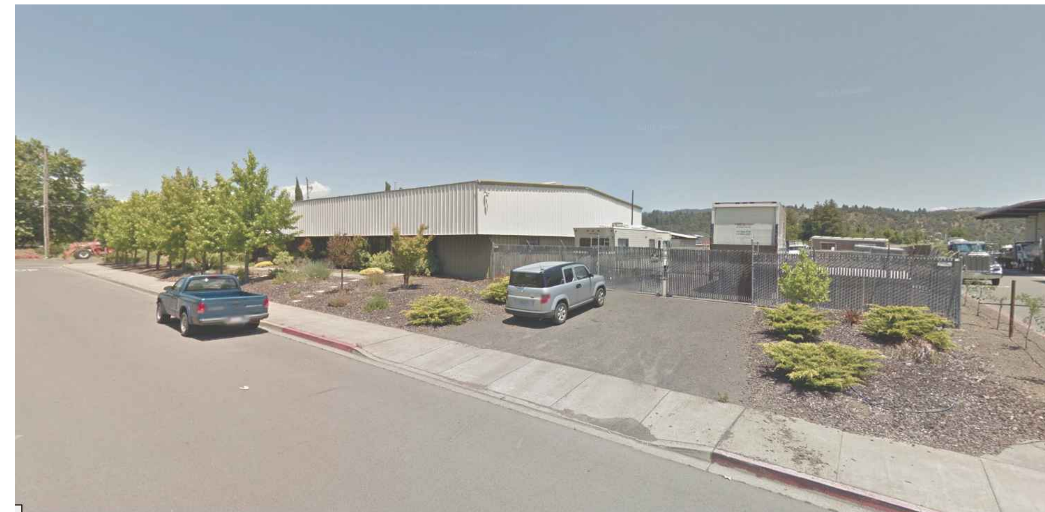
EXISTING SITE PHOTOS - SOUTH SCALE: NTS 1
