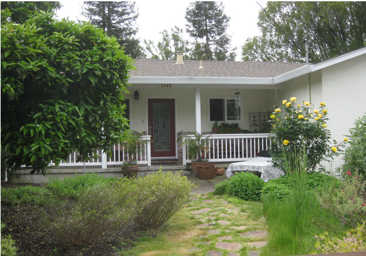
EXISTING RESIDENCE - FRONT/PORCH ELEVATION
