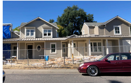
1401 Allyn Ave. – In Progress
