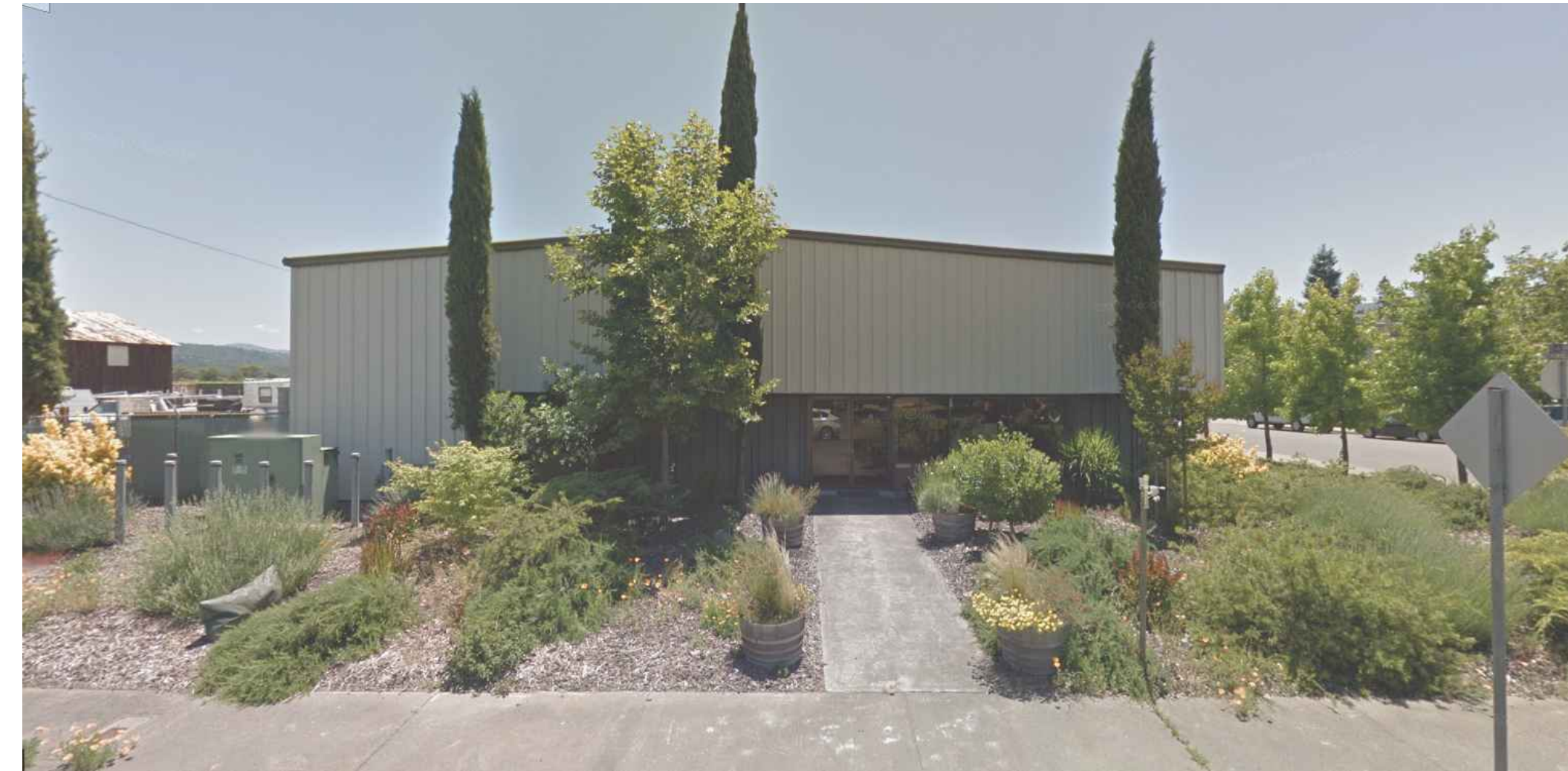
EXISTING SITE PHOTOS - NORTH WEST
