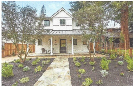
1645 Vineyard Ave – Completed 2018
