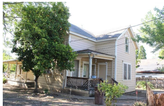
Photograph 7: Northeast and northwest elevations, camera facing south, May 4, 2018.
