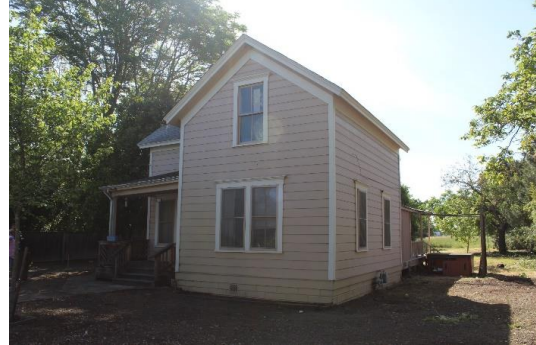
Photograph 3: Northwest and southwest elevations, camera facing east, May 4, 2018.
