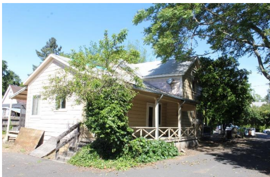
Photograph 6: Southeast and northeast elevations, camera facing west, May 4, 2018.
