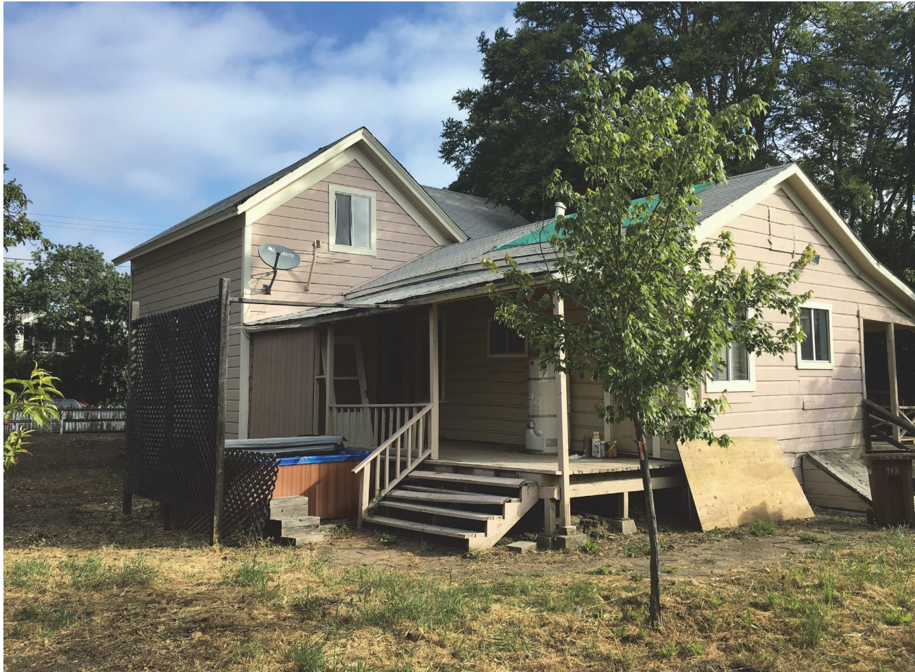
7. VIEW FROM SOUTHWEST
