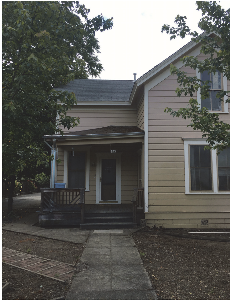
2. VIEW FROM NORTH - STREET ELEVATION
