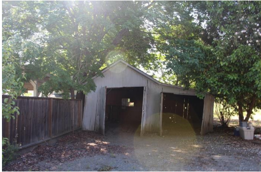
Photograph 8: Garage, northwest elevation, camera facing southeast, May 4, 2018.
