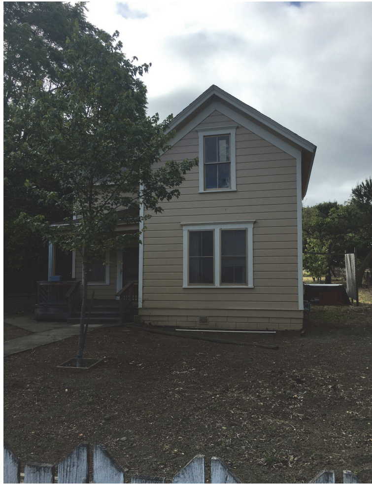
3. VIEW FROM NORTH - STREET ELEVATION
