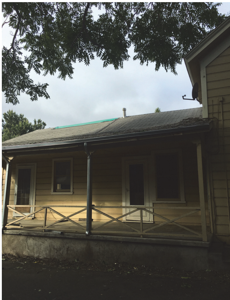
11. VIEW FROM EAST - SIDE PORCH
