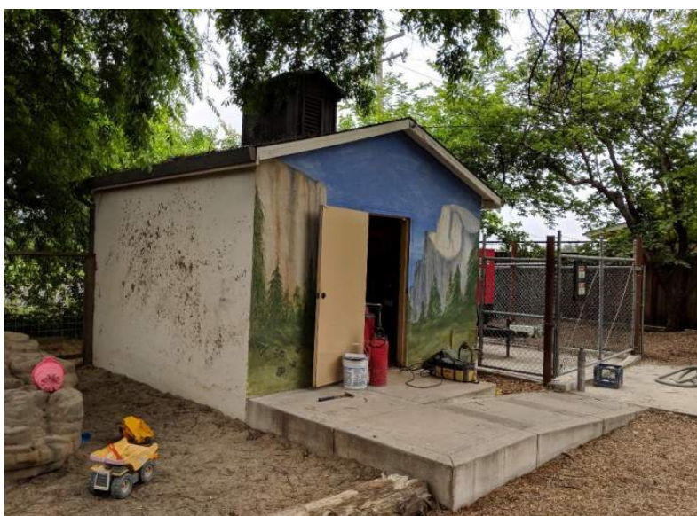
Photo 1: Crinella Pump House Building
