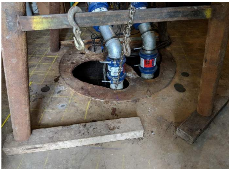
Photo 3: Existing Wet Well Opening
