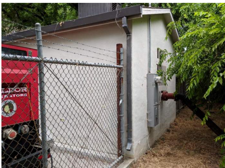
Photo 2: Pump House Building Rear
