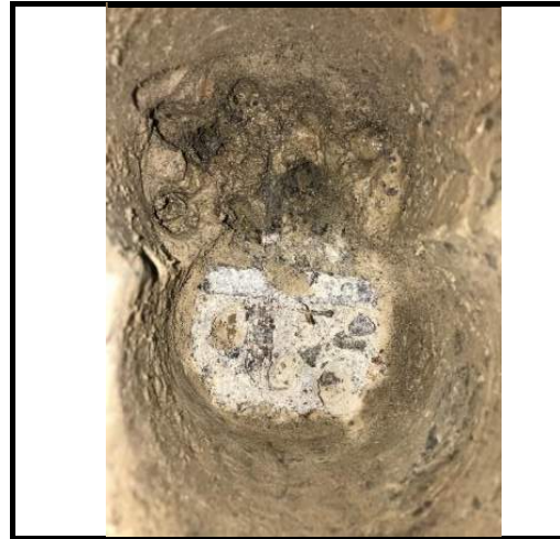
# 4 Reinforcing Steel (Each Way)
