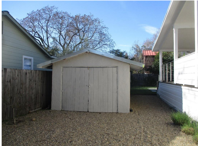
Figure 15. Southeast elevation, facing northwest.
