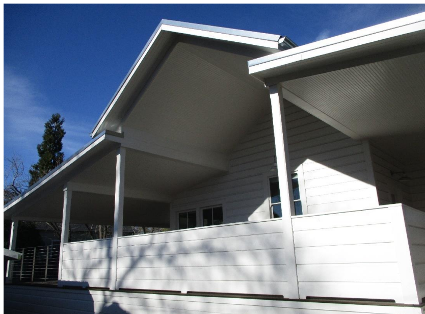
Figure 9. Southwest elevation, facing north.
