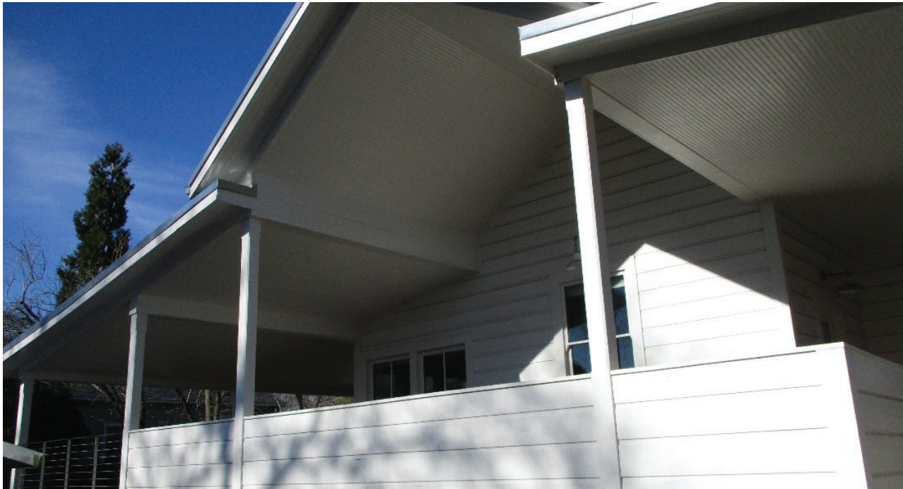
Roof Covered South Deck
