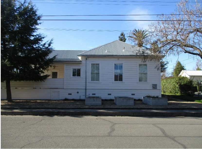
Southeast elevation, facing northwest.
