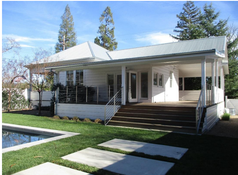
Figure 10. Northwest elevation facing east.
