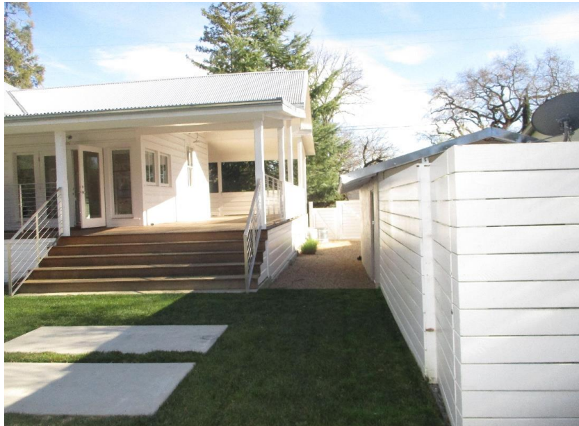
Figure 16. Photo showing the wood fence that extends from the rear of the ca. 1925 garage.
