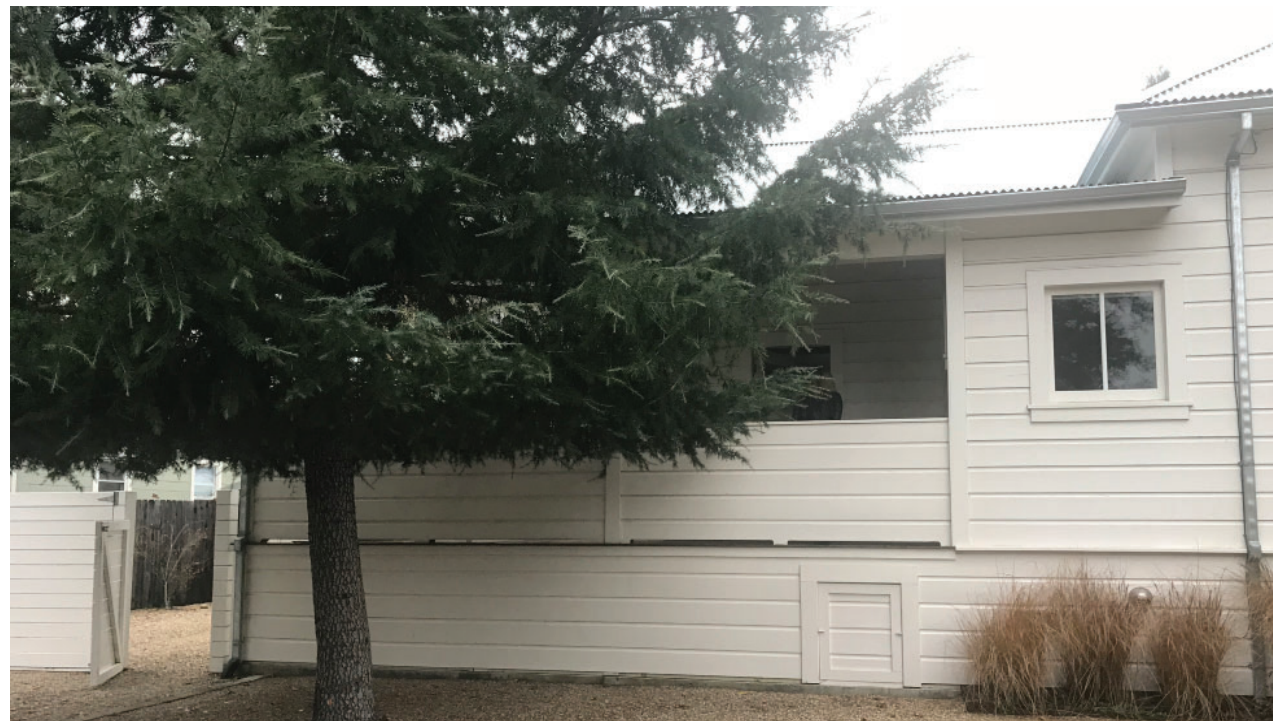
Covered South Deck from Tainter Street
