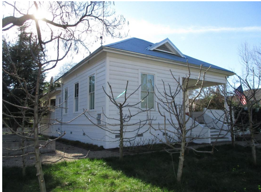
Figure 7. Northeast elevation, facing west.
