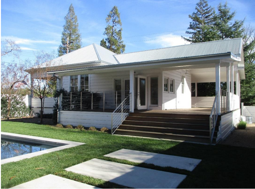
Northwest elevation facing east.
