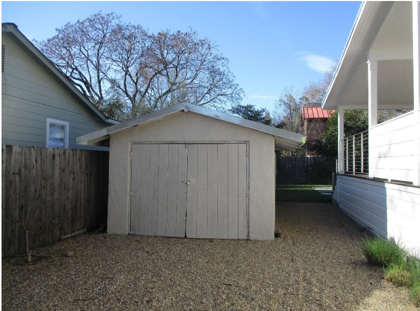
Southeast elevation, facing northwest.
