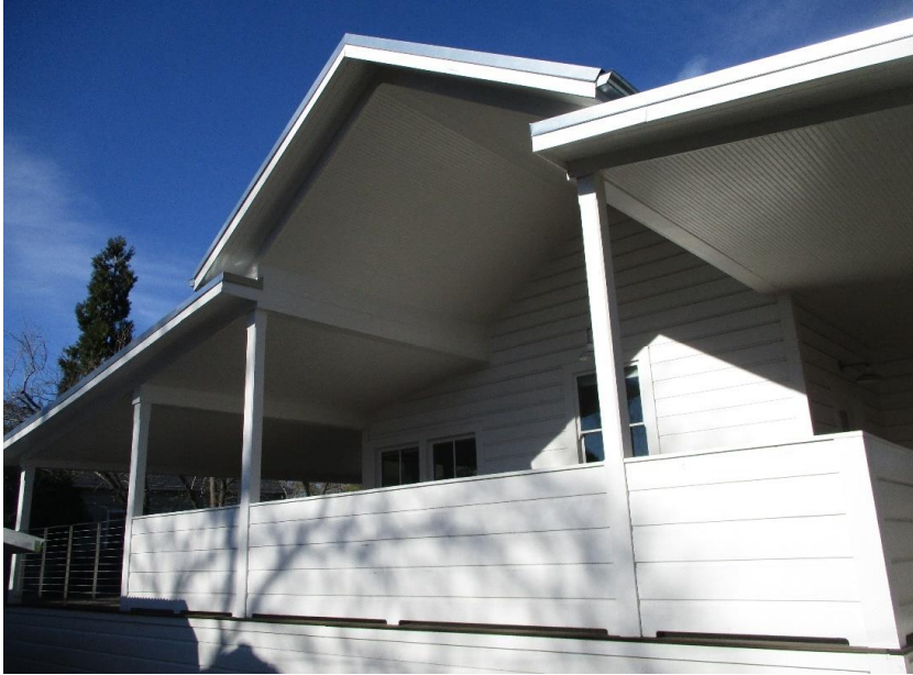
Southwest elevation, facing north.
