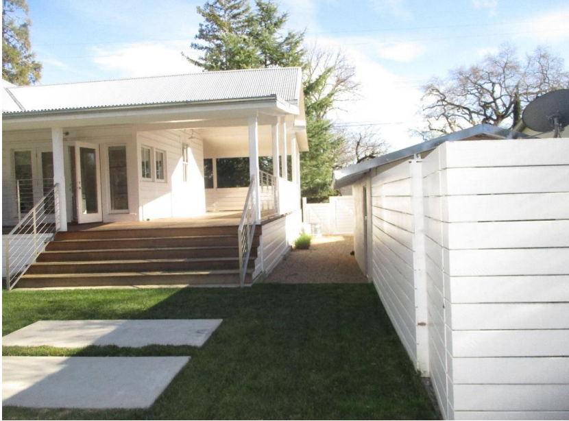
Photo showing the wood fence that extends from the rear of the ca. 1925 garage.
