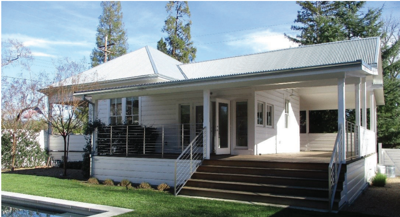
West Back Yard - Looking at roof covered south deck
