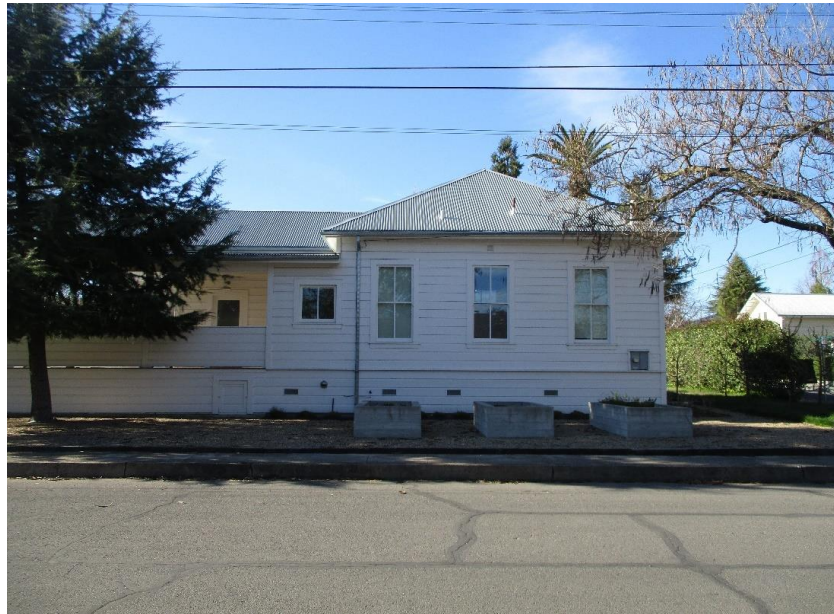
Figure 8. Southeast elevation, facing northwest.
