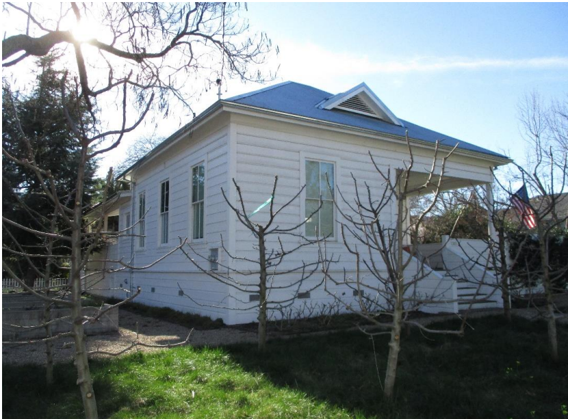
Northeast elevation, facing west.
