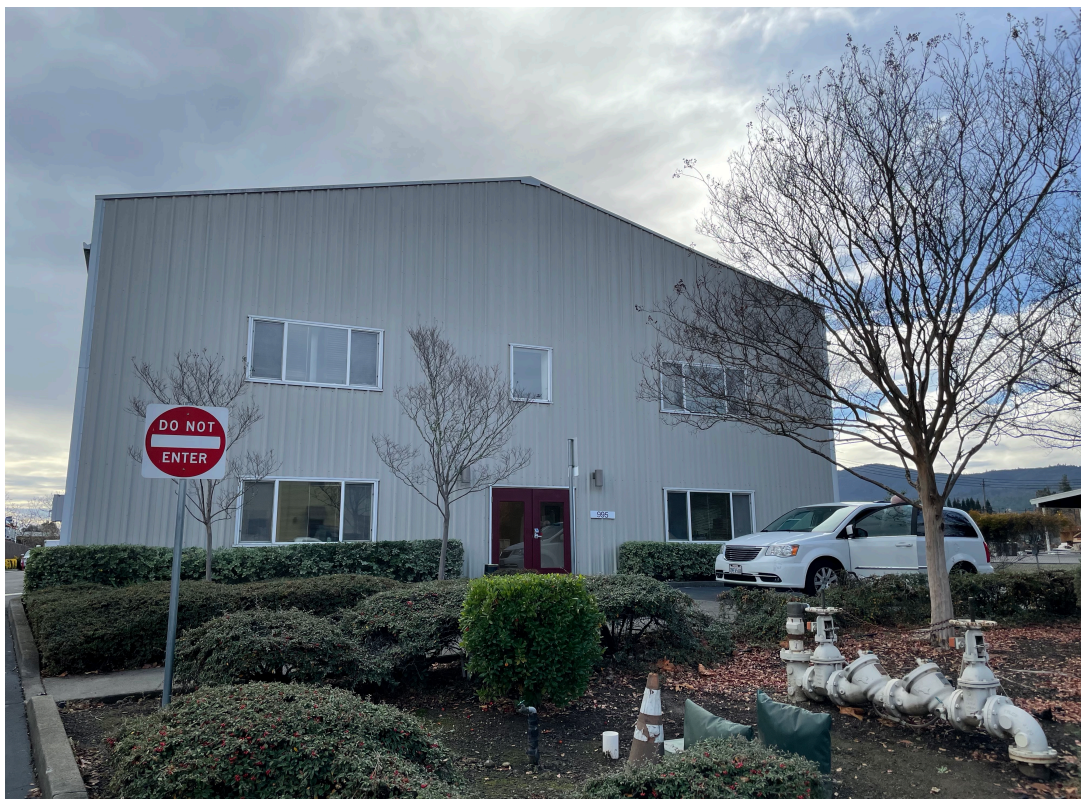
Front of Building - Western Side
