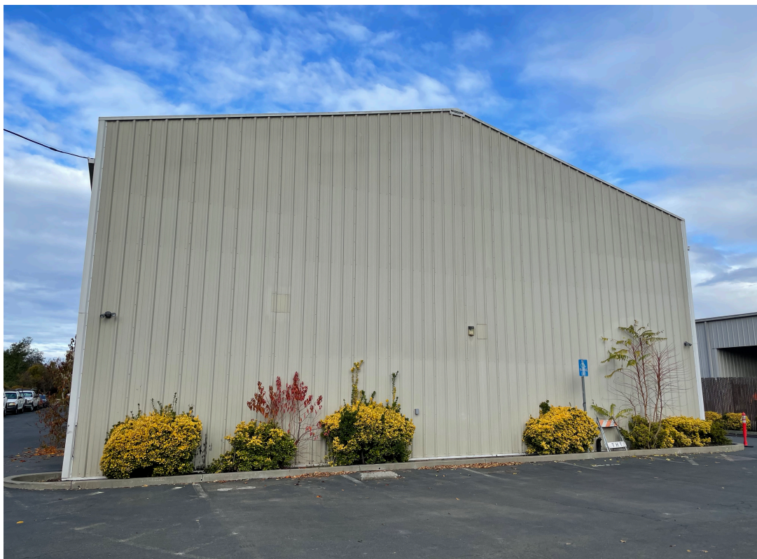
Back of Building - Eastern Side
