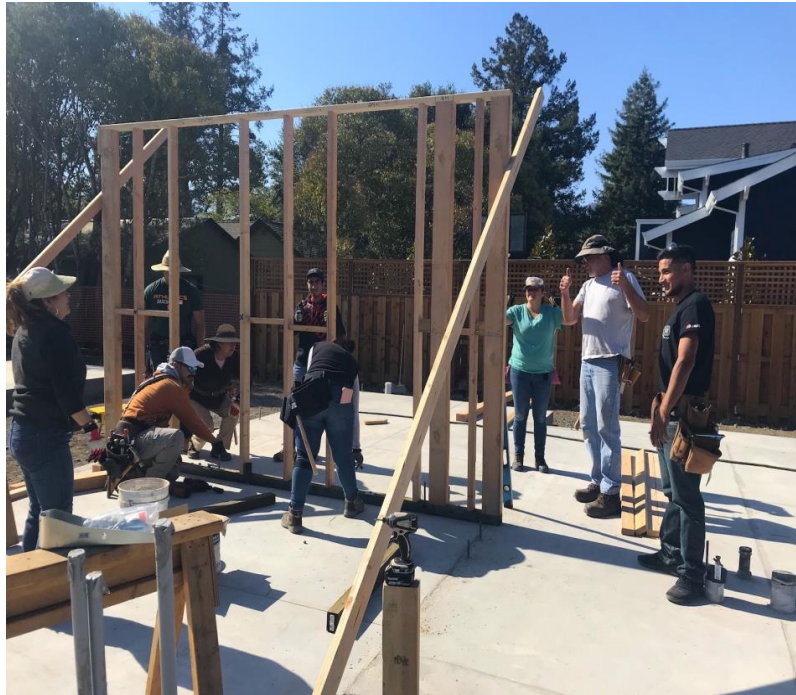
Brenkle Court Self-Help Housing Project 8 townhomes, ownership Completion: August 2021
