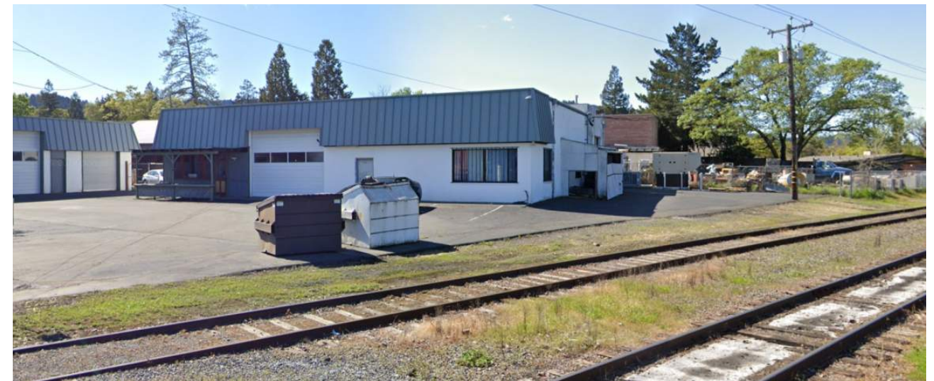
Photo 4 - view of front and eastern elevations of 1020 Fulton Lane. Wine Train tracks are visible in foreground.
