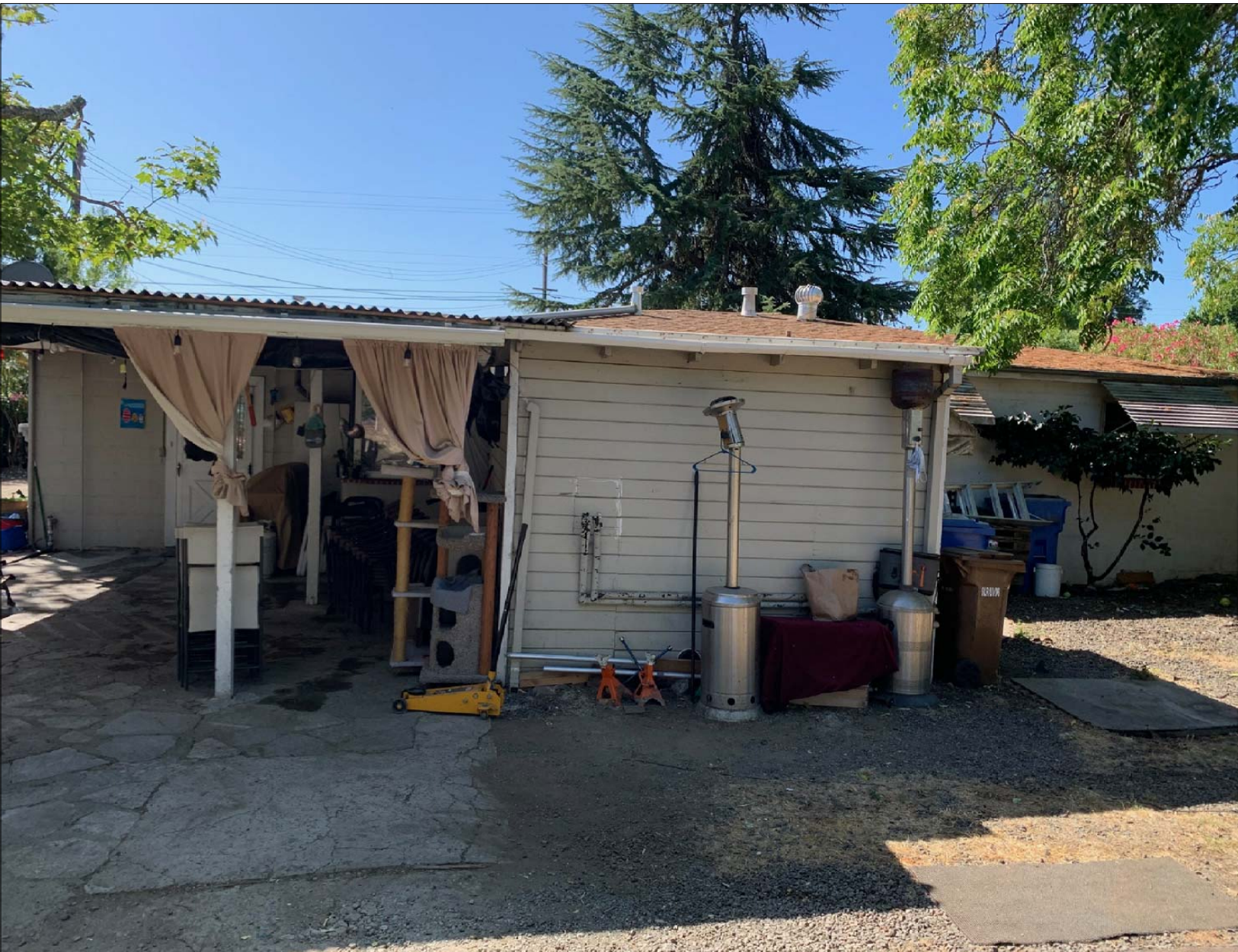
MAIN HOUSE PATIO
