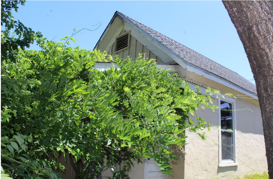
Photograph 4: 1420 Allyn Avenue, northwest elevation, camera facing east, May 10, 2021.
