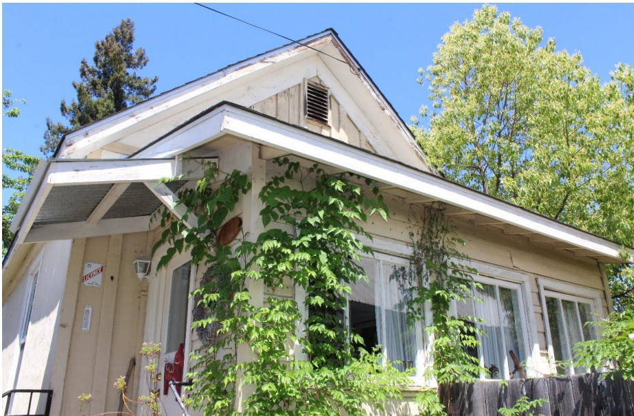
Photograph 7: 1420 Allyn Avenue, southeast elevation, camera facing north, May 10, 2021.
