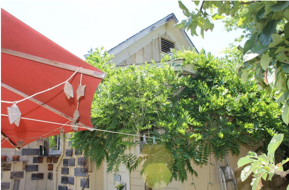
Photograph 5: 1420 Allyn Avenue, northwest elevation, camera facing south, May 10, 2021.
