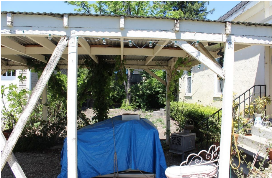
Photograph 9: 1420 Allyn Avenue, southwest elevation carport, camera facing northwest, May 10, 2021.
