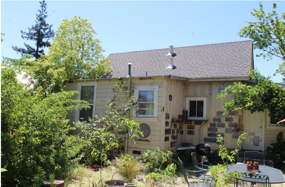
Photograph 6: 1420 Allyn Avenue, northeast elevation, camera facing southwest, May 10, 2021.
