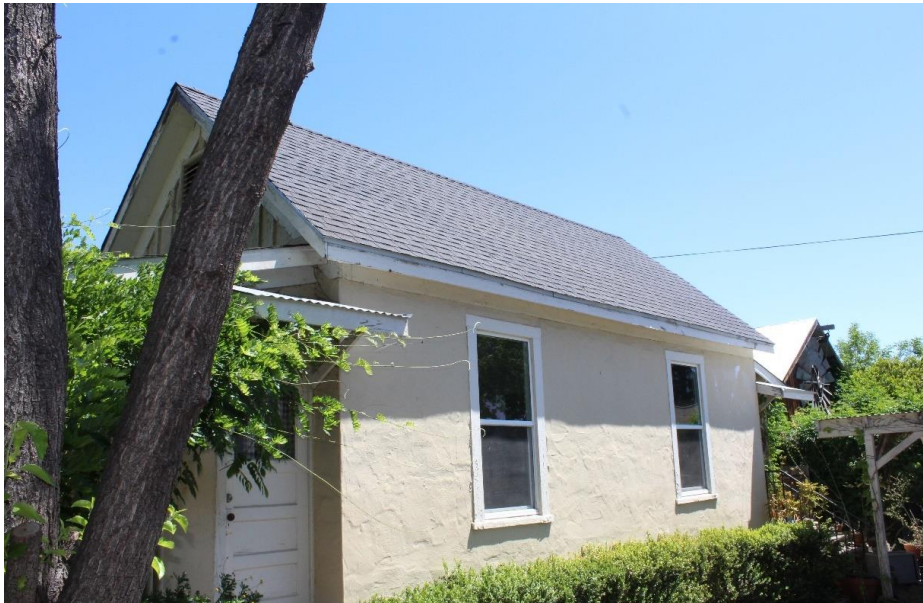
Photograph 3: 1420 Allyn Avenue, southwest elevation, camera facing east, May 10, 2021.
