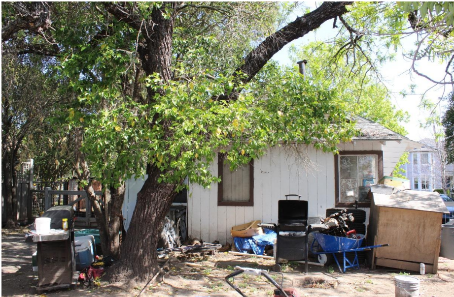
Photograph 7: 1547 Allyn Avenue, southwest elevation, camera facing northeast, April 9, 2021.
