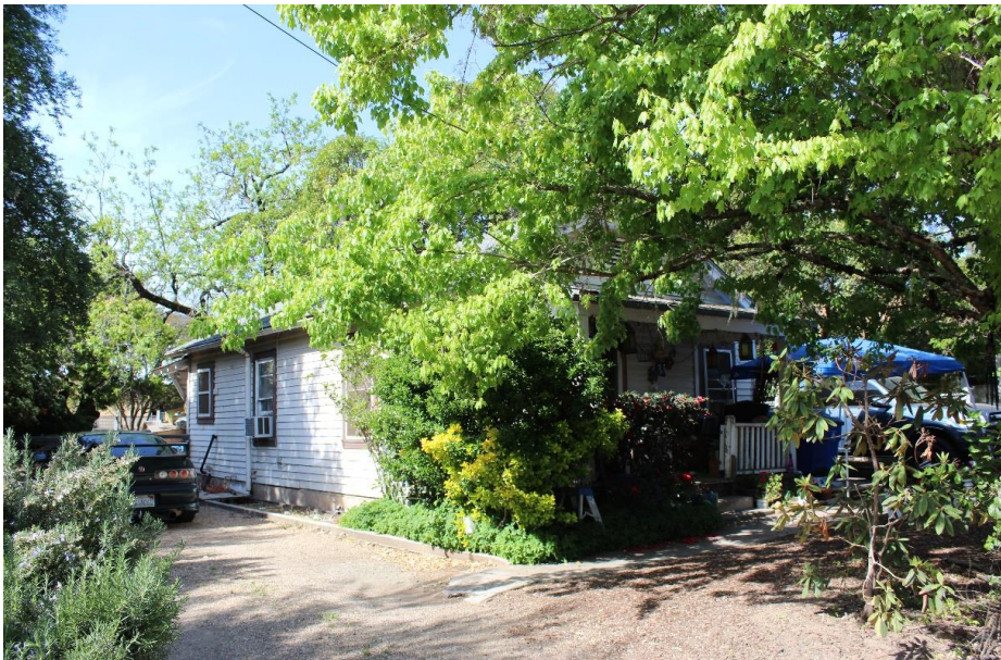
Photograph 5: 1547 Allyn Avenue, southeast and northeast elevations, camera facing southwest, April 9, 2021.
