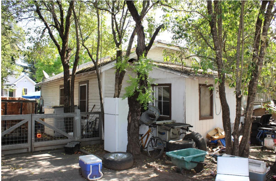
Photograph 8: 1547 Allyn Avenue, northwest and southwest elevations, camera facing northeast, April 9, 2021.
