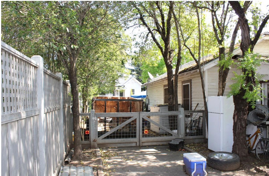
Photograph 9: 1547 Allyn Avenue, northwest elevation, camera facing north, April 9, 2021.
