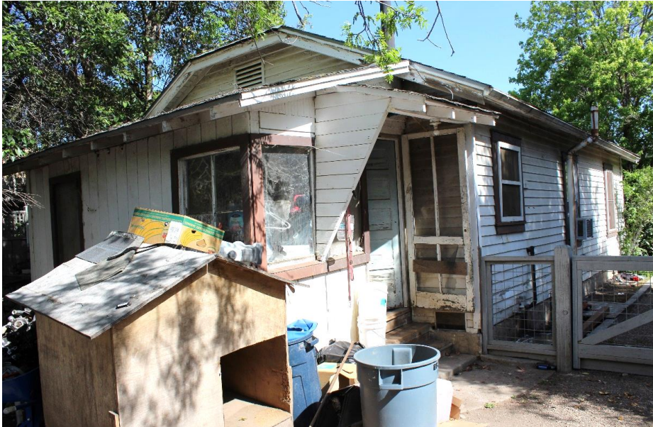
Photograph 6: 1547 Allyn Avenue, southeast and southwest elevations, camera facing northwest, April 9, 2021.
