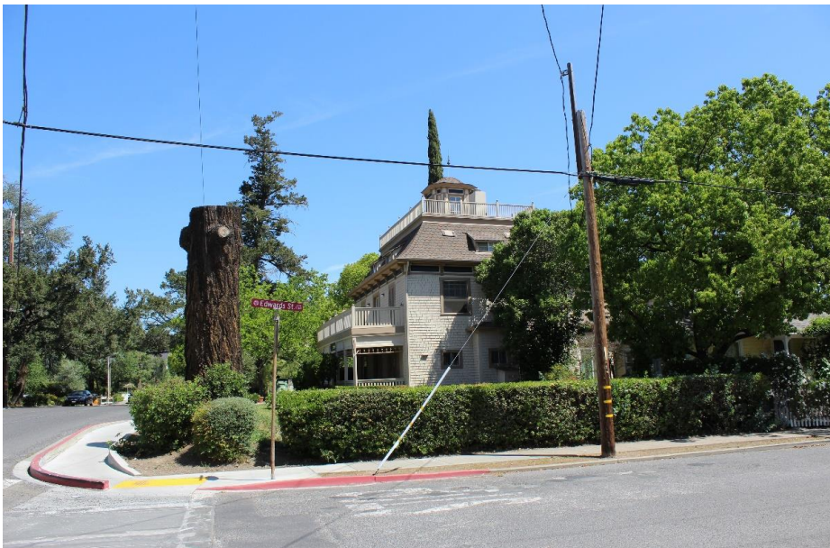
Photograph 6: View from 1227 Edwards St. looking towards Hunt Avenue, camera facing north, April 19, 2021.
