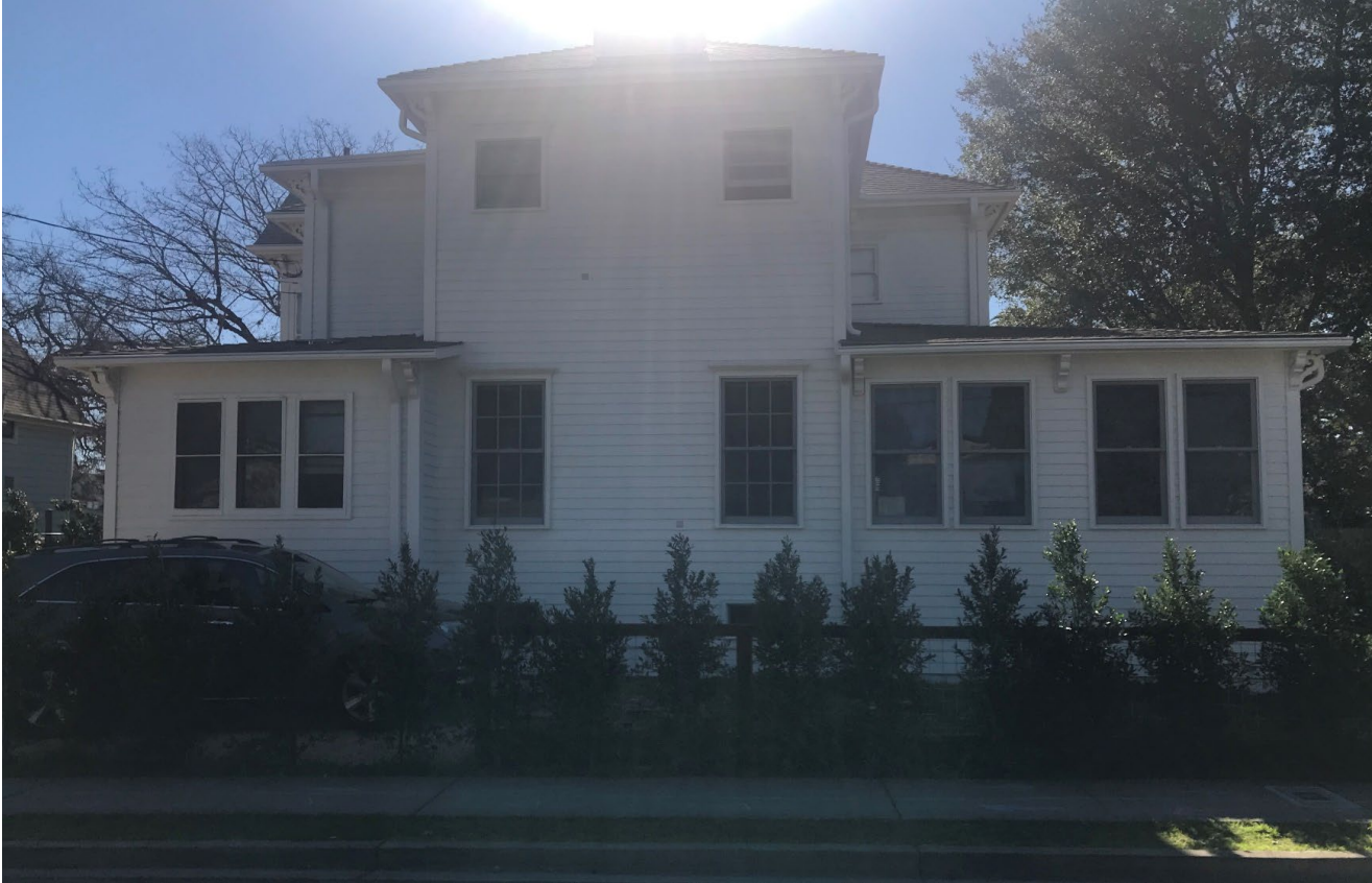
1227 Edwards Street | North Elevation | Side of House, viewed from Edwards Street
