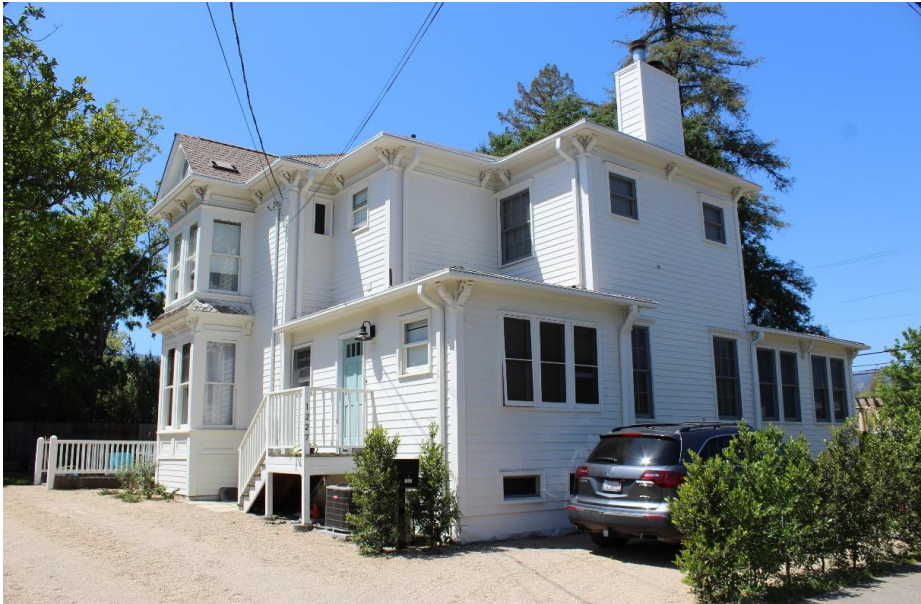
Photograph 2: 1227 Edwards St., southeast and northeast elevations, camera facing west, April 19, 2021.
