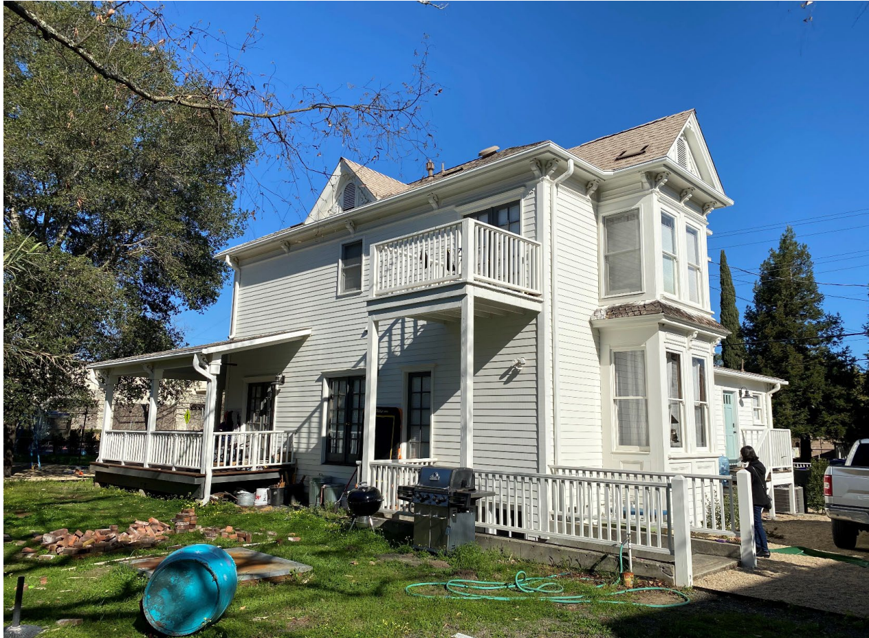
1227 Edwards Street | Southeast Corner | Side of house, viewed from backyard
