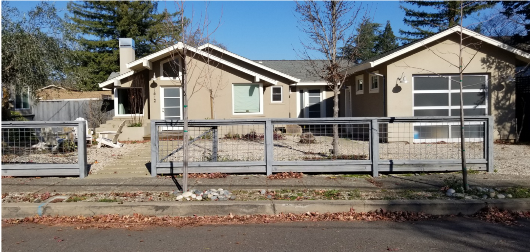
Picture #1 - Front View
