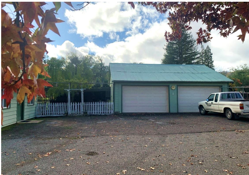
Photograph 7: 2126 Madrona Avenue garage, northeast elevation, camera facing south, November 10, 2021.
