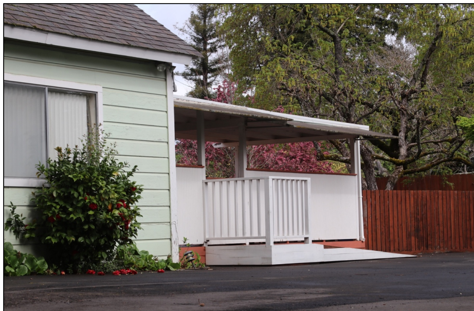
Figure 10: East elevation, porch and handicap ramp
