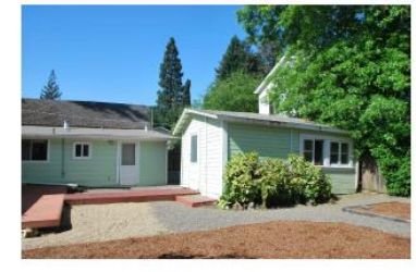
Existing Back Unit
