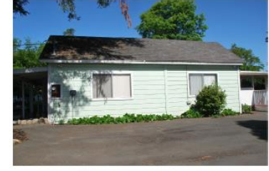
Existing Side Right View
