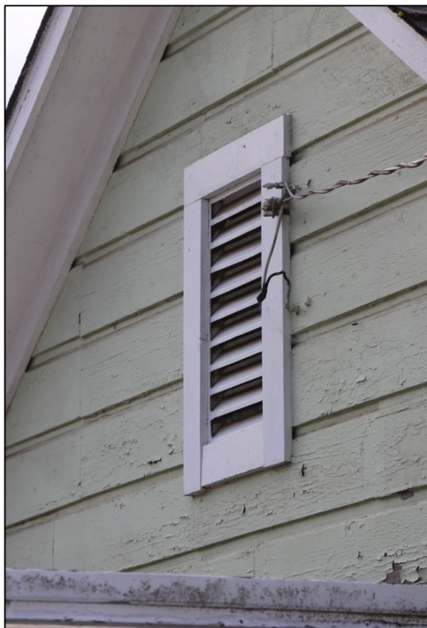
Figure 16: North elevation, gable vent
