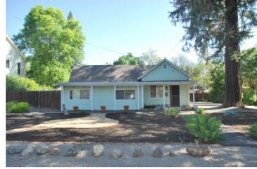
Existing Front View
