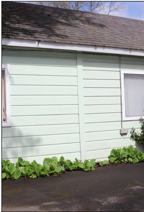
Figure 11: East elevation, siding detail
