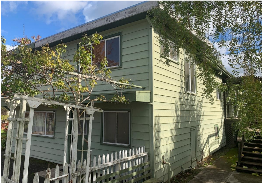
Photograph 5: 2126 Madrona Avenue, northwest and southwest elevations, camera facing northeast, November 10, 2021.
