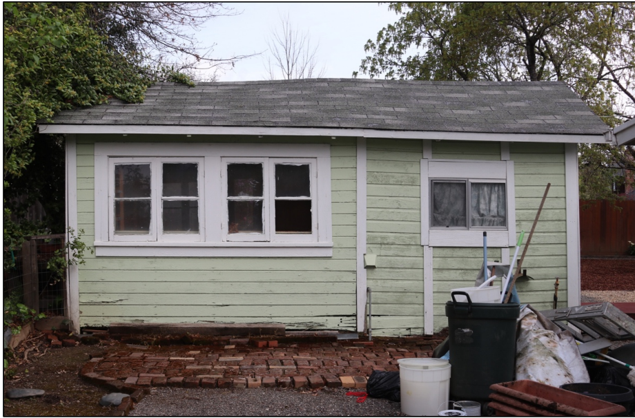
Figure 23: Auxiliary building, south elevation
