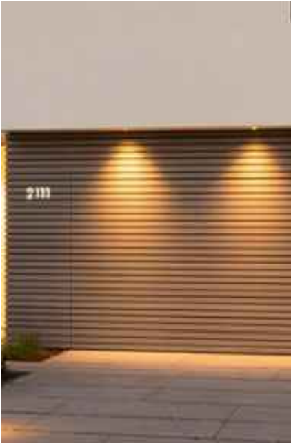
CEMENT PLASTER & WOOD WALLS
