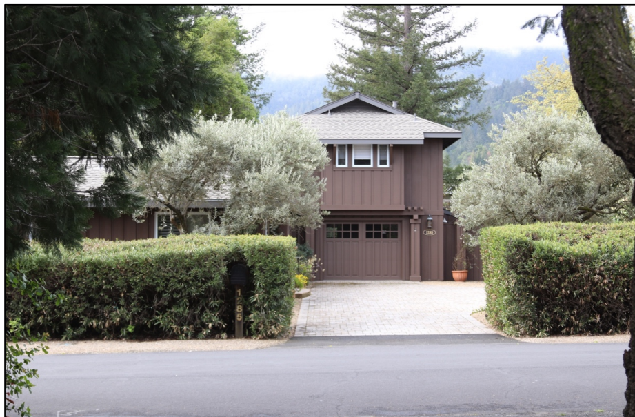
Figure 31: Neighbor across the street (1285 Hudson Ave.)
