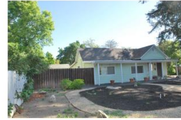
Existing Side Left View
