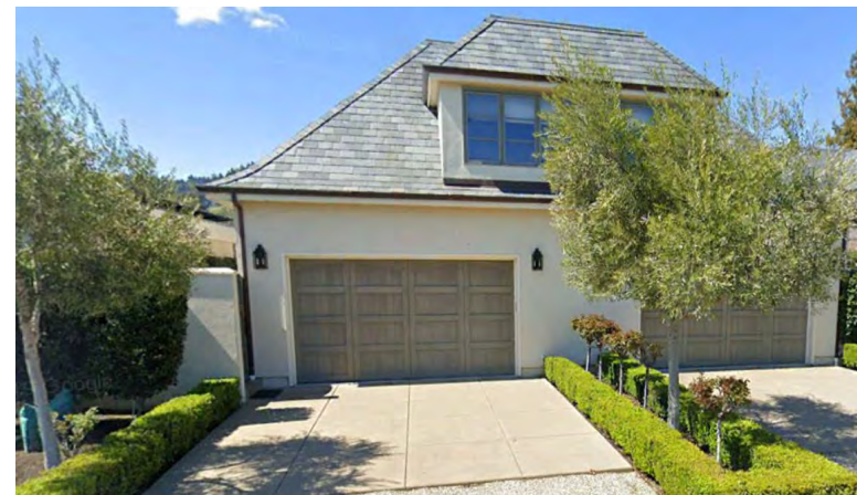
2056 Madrona Avenue, adjacent to project on Madrona Avenue
