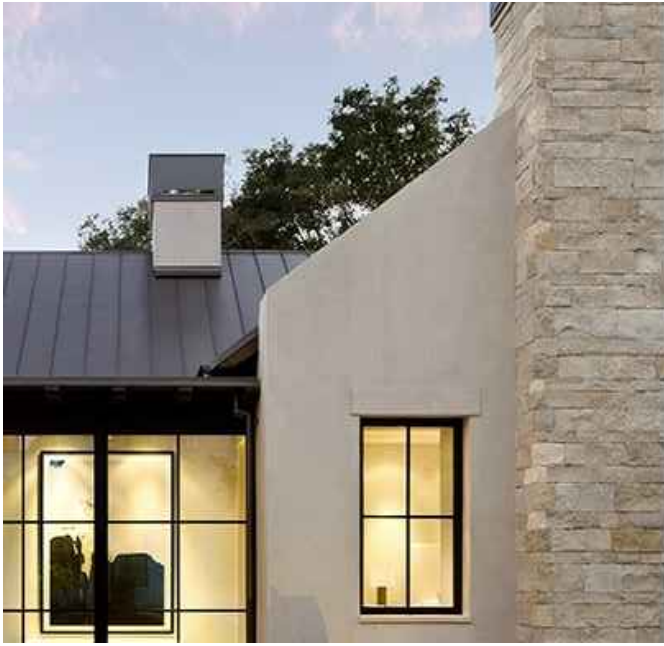
STONE VENEER & CEMENT PLASTER WALLS WITH DARK METAL WINDOW FRAMES
