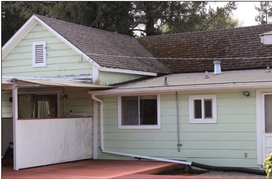
Figure 12: North elevation, rooflines
