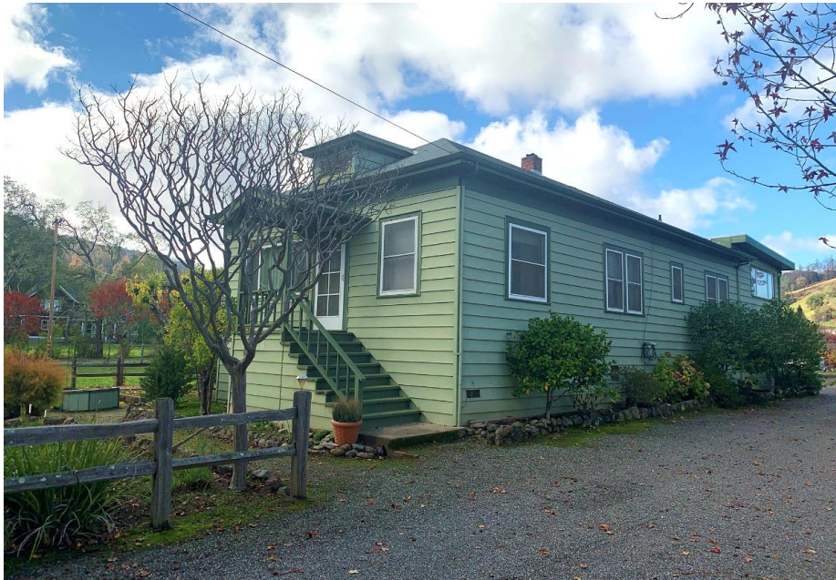
Photograph 2: 2126 Madrona Avenue, southeast and northeast elevations, camera facing southwest, November 10, 2021.
