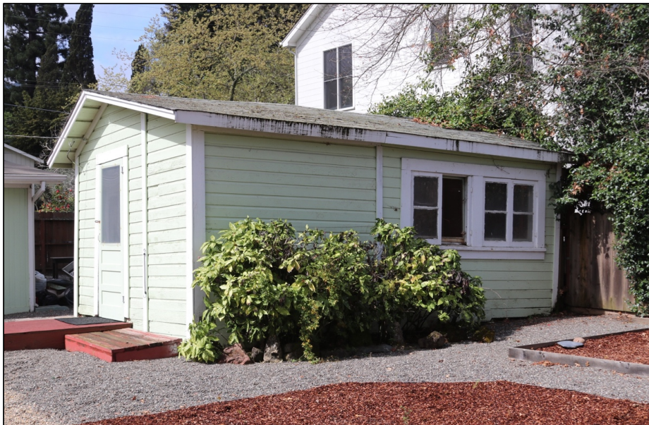
Figure 24: Auxiliary building, north elevation
