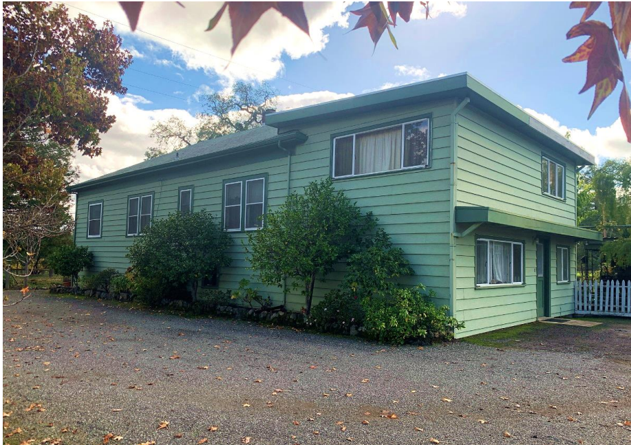
Photograph 3: 2126 Madrona Avenue, northeast and northwest elevations, camera facing southeast, November 10, 2021.
