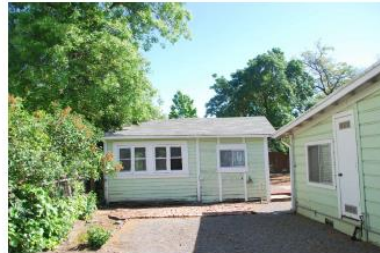
Existing Side Left View
