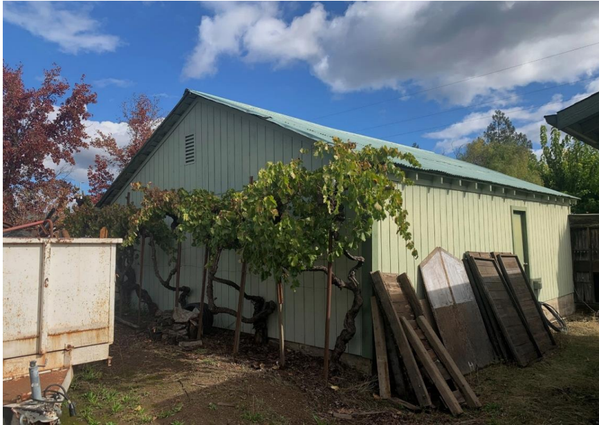
Photograph 8: 2126 Madrona Avenue garage, southwest and southeast elevations, camera facing northwest, November 10, 2021.
