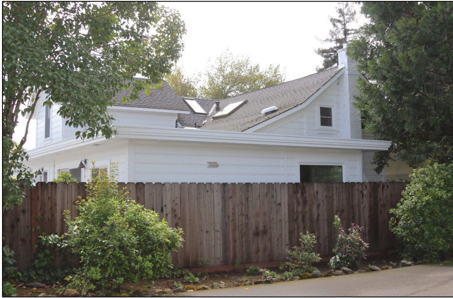
Figure 29: Neighbor to the east (1296 Hudson Ave.)
