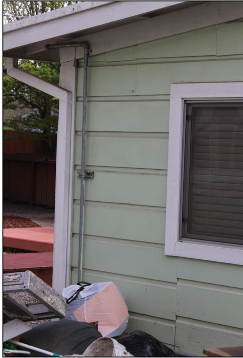
Figure 21: West elevation, siding detail at northwest corner
