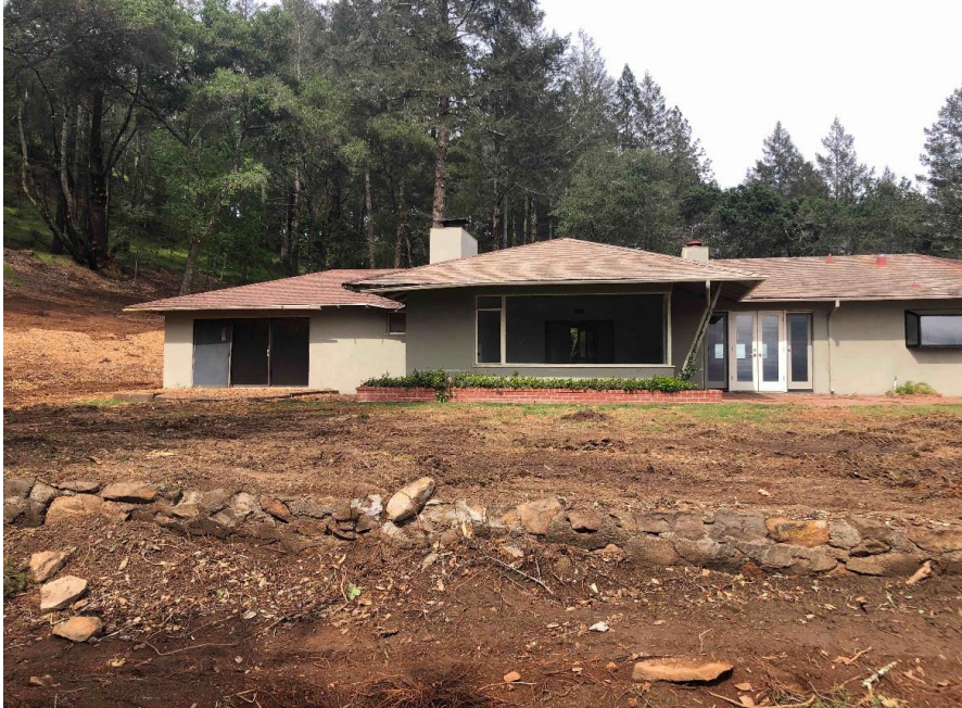
Photograph 4: 2484 Spring Mountain Road, east elevation, camera facing west, March 3, 2022.
