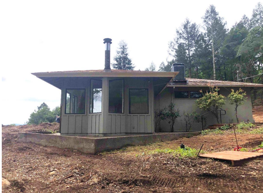
Photograph 6: 2484 Spring Mountain Road, north elevation, camera facing south, March 3, 2022.
