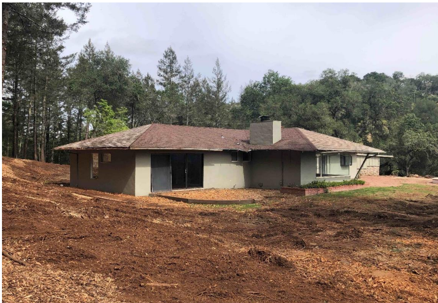
Photograph 3: 2484 Spring Mountain Road, southwest and east elevations, camera facing north, March 3, 2022.
