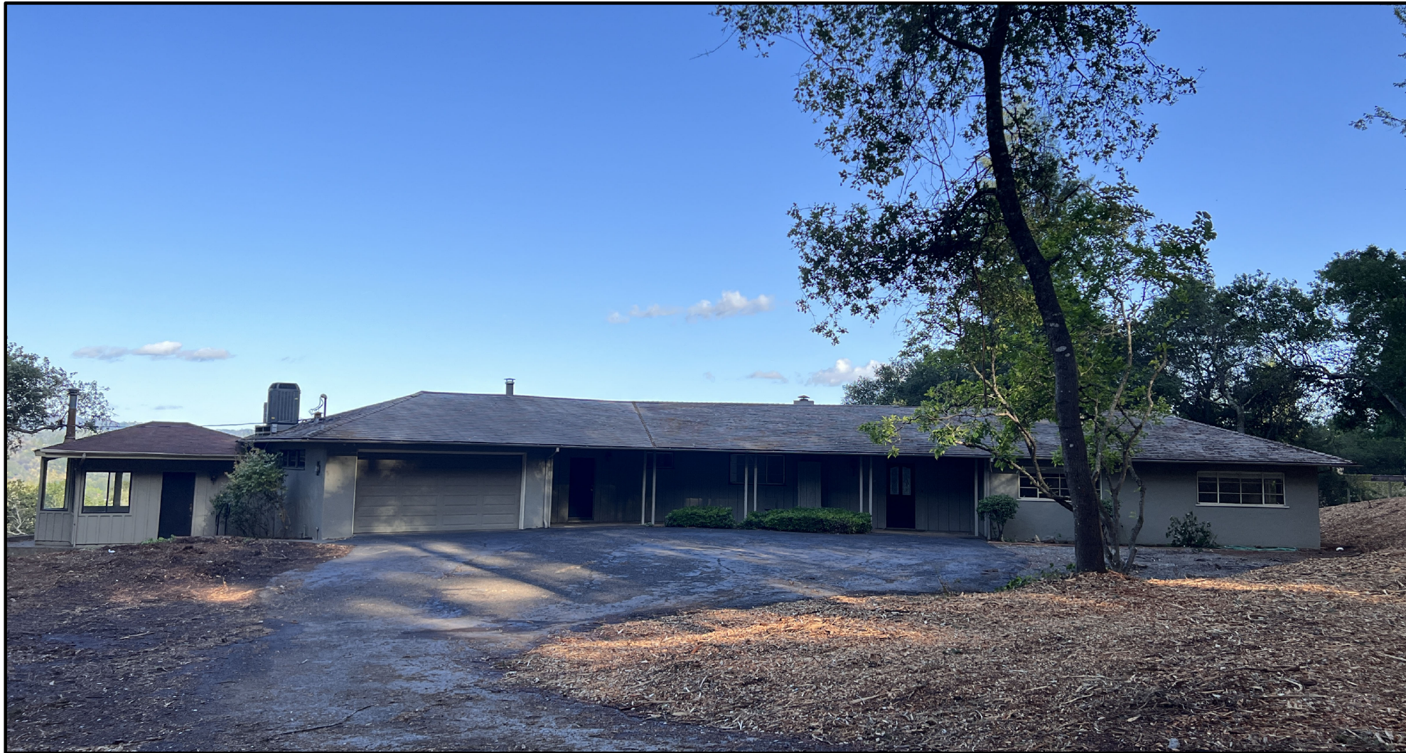
EXISTING PHOTO - FRONT
