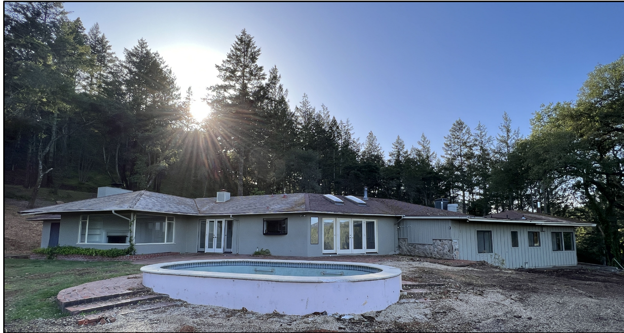
EXISTING PHOTO - REAR
