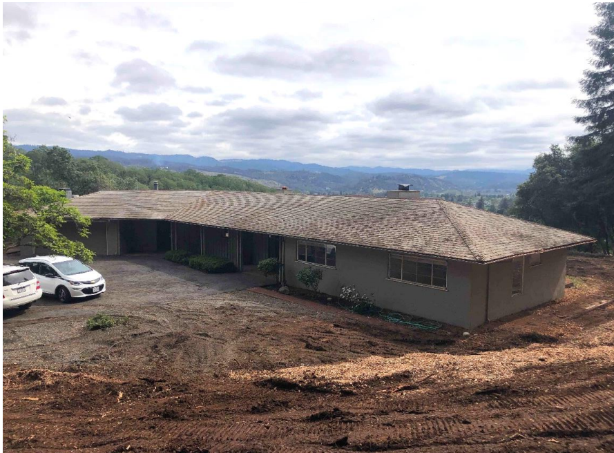
Photograph 2: 2484 Spring Mountain Road, northwest and southwest elevations, camera facing northeast, March 3, 2022.
