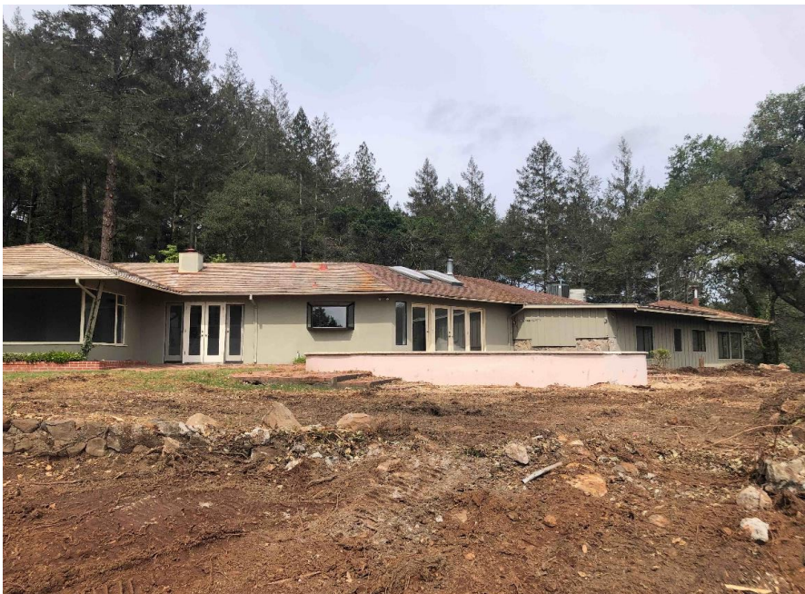
Photograph 5: 2484 Spring Mountain Road, east elevation, camera facing west, March 3, 2022.
