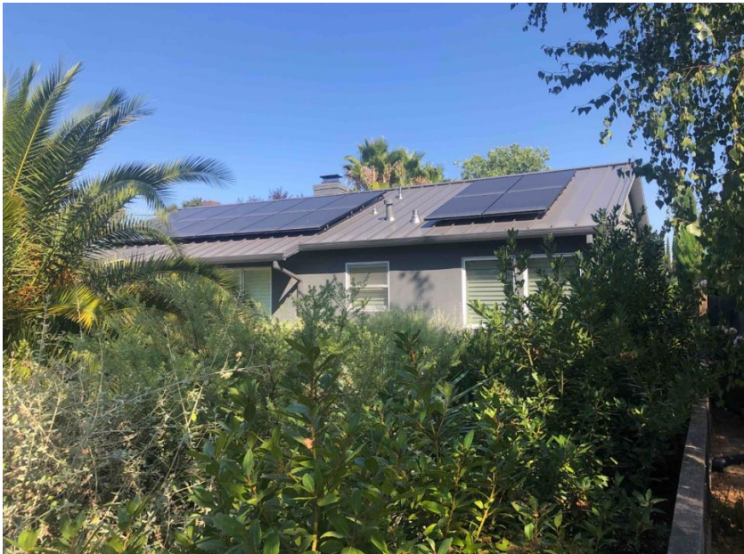
Photograph 3: 1663 Adams St, northwest elevation, camera facing southeast, August 16, 2022.
