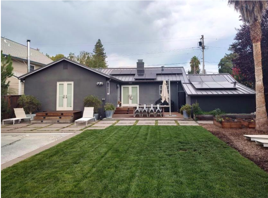
Photograph 6: 1663 Adams St, southeast elevation, camera facing northwest, August 16, 2022.
