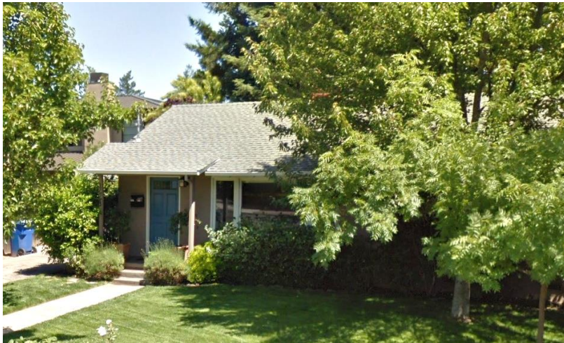
Figure 1: 1663 Adams Street, northwest elevation, camera facing southeast, 2011.
