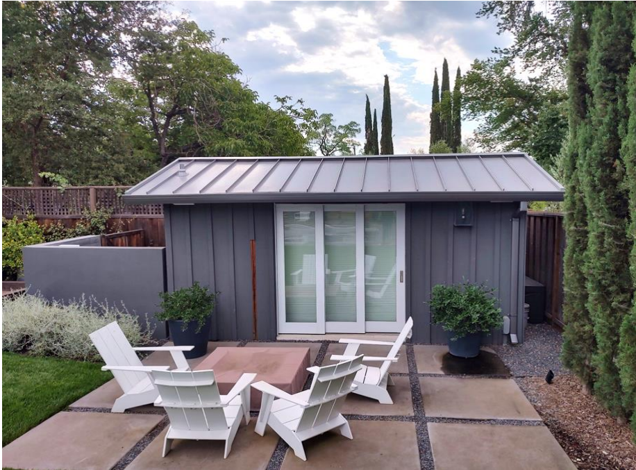
Photograph 8: 1663 Adams St pool house, northwest elevation, camera facing southeast, August 16, 2022.
