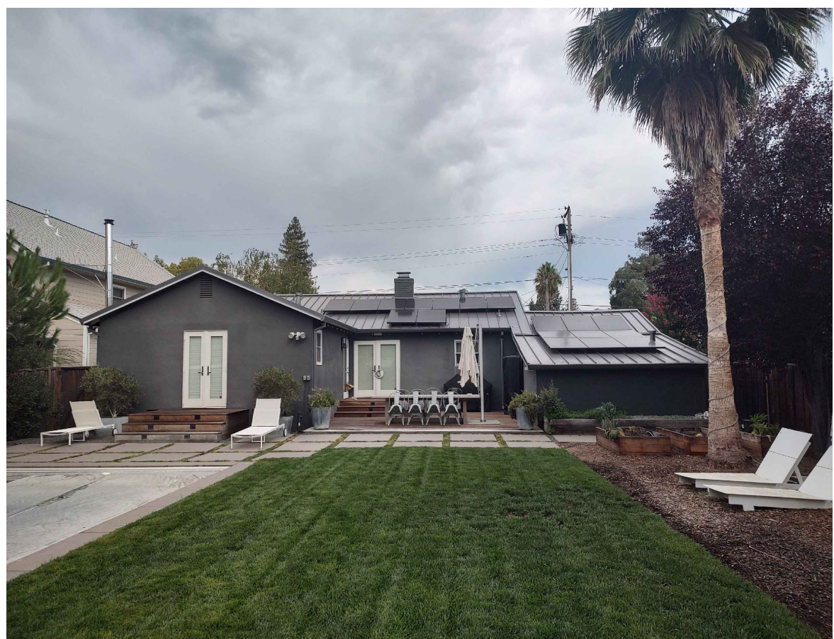
VIEW OF EXISTING RESIDENCE FROM BACKYARD SCALE: N.T.S.
