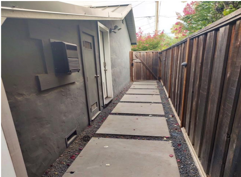
Photograph 5: 1663 Adams St, northeast elevation, camera facing west, August 16, 2022.
