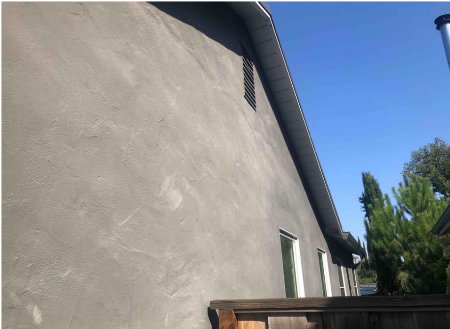
Photograph 7: 1663 Adams St, southwest elevation, camera facing east, August 16, 2022.
