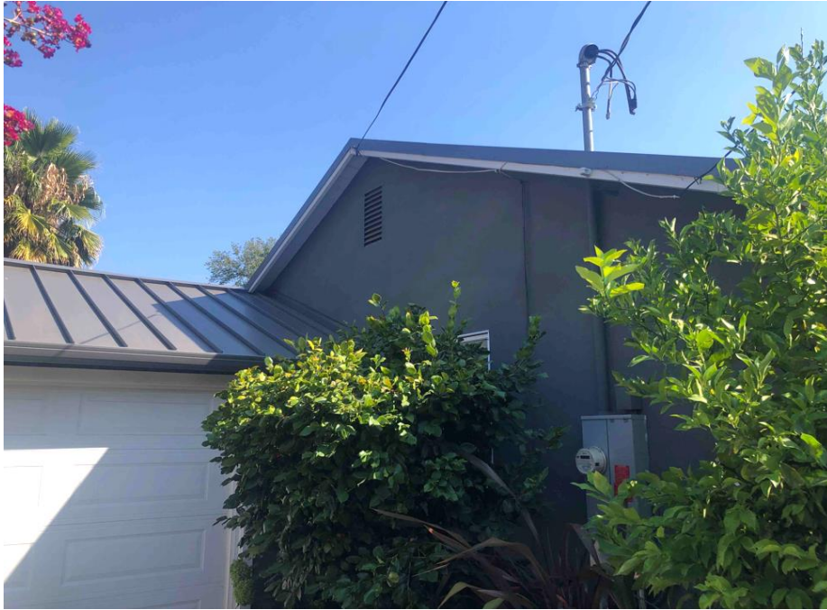
Photograph 4: 1663 Adams St, northwest and northeast elevations, camera facing south, August 16, 2022.
