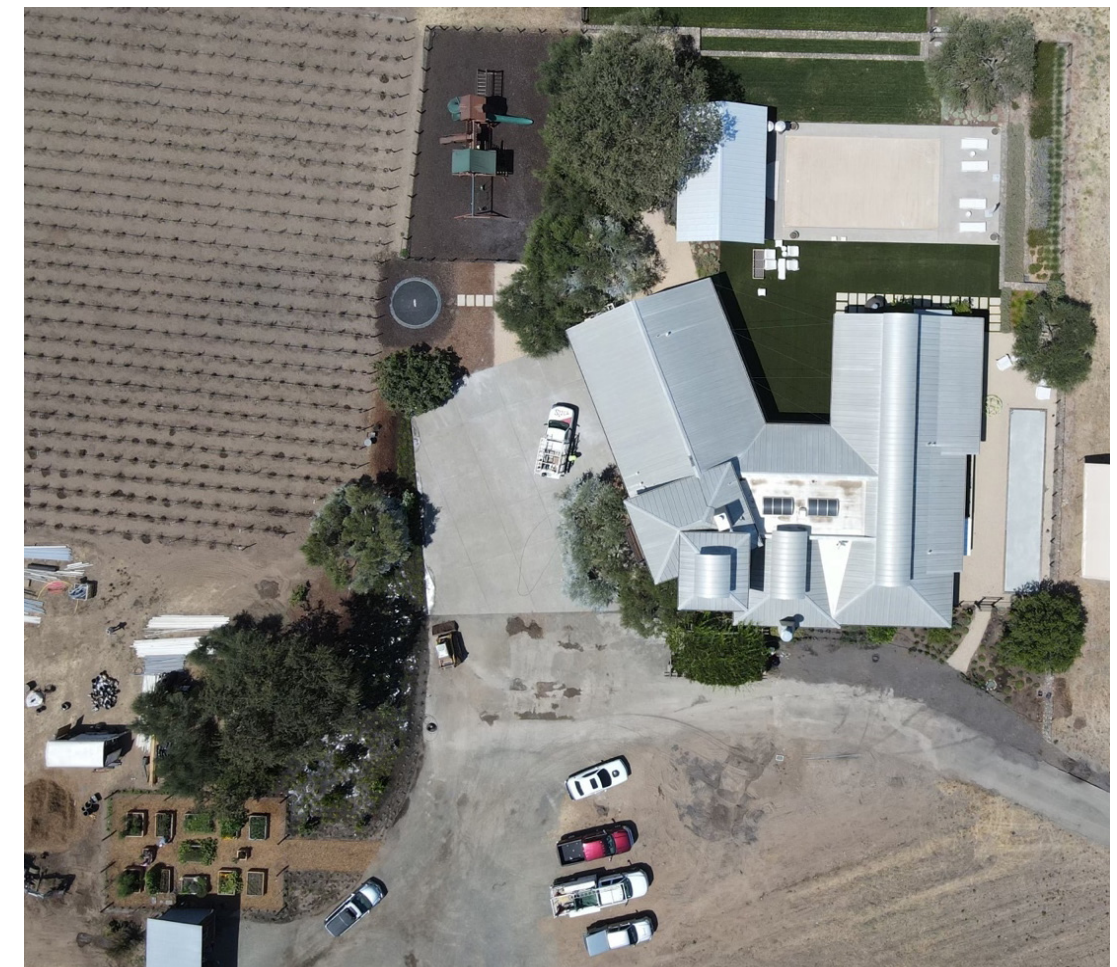
A: (E) MAIN HOUSE, POOL AND PERGOLA
