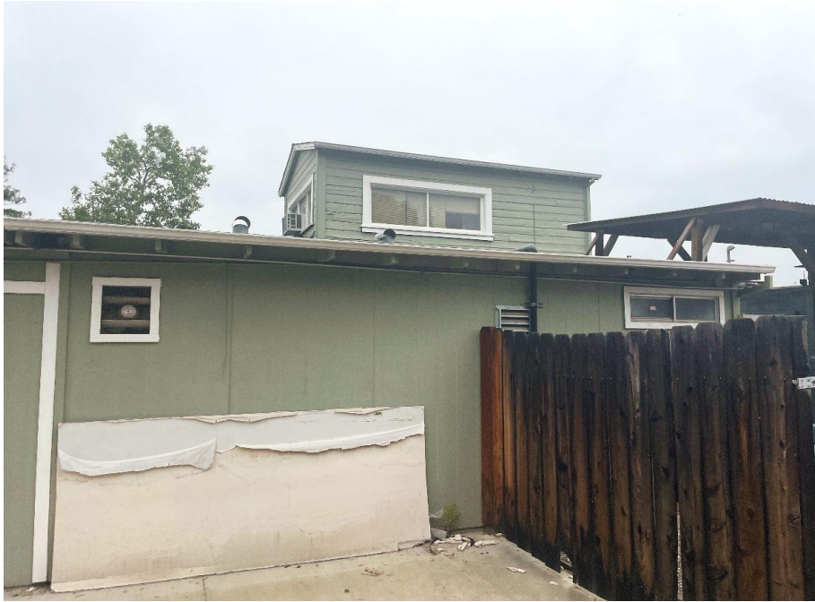
Photograph 4: 61 Main Street, southwest elevation, camera facing northeast, June 17, 2023.
