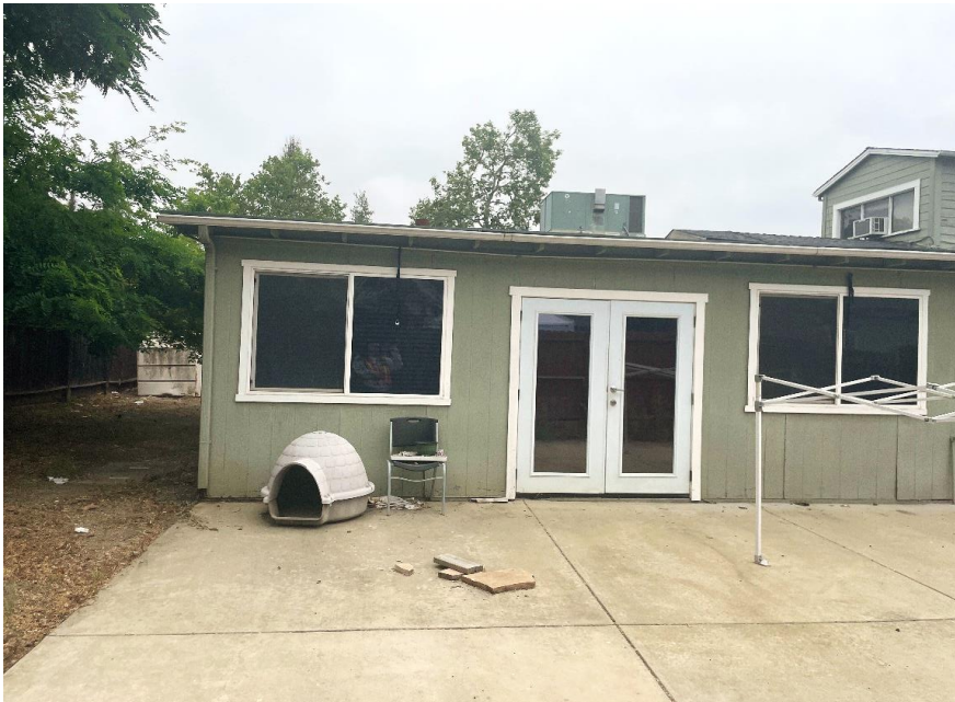
Photograph 3: 61 Main Street, southwest elevation, camera facing northeast, June 17, 2023.
