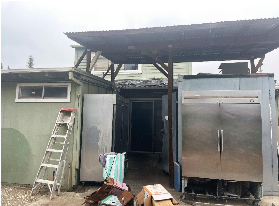
Photograph 5: 61 Main Street, southwest elevation, camera facing northeast, June 17, 2023.
