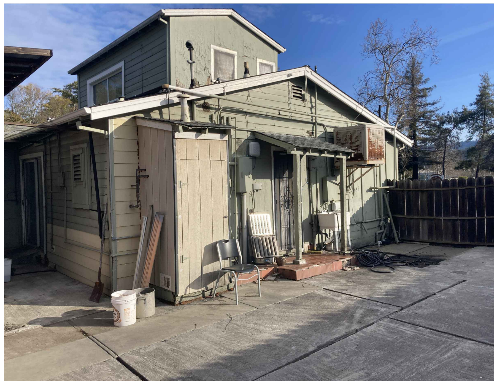
⑦ SIDE YARD, EAST
