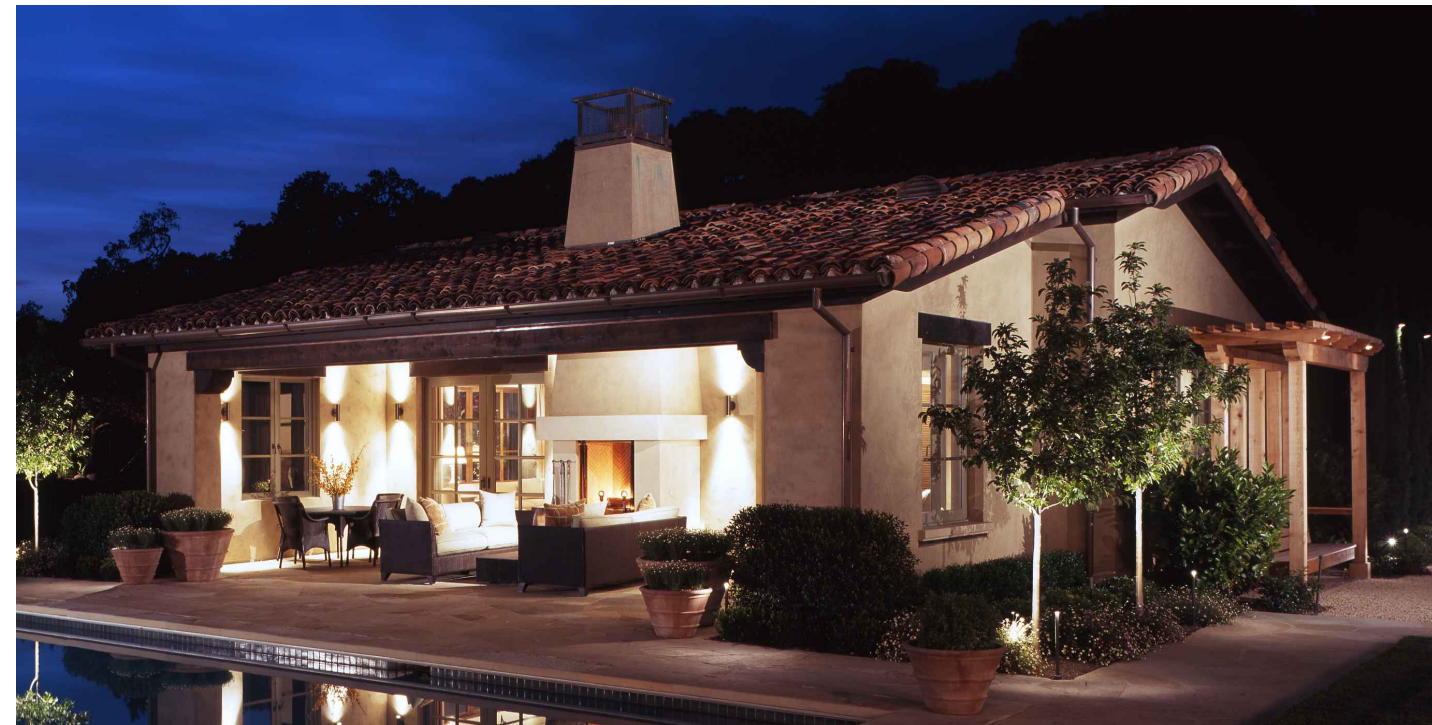
CEMENT PLASTER WALLS
