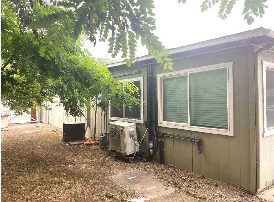
Photograph 2: 61 Main Street, northwest elevation, camera facing east, June 17, 2023.
