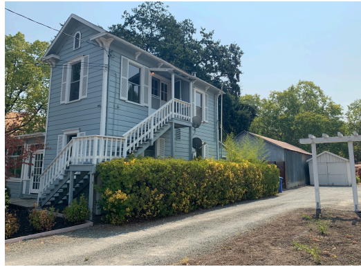
Front west corner of Site showing exterior staircase and driveway for adjacent property at 963 Pope Street
