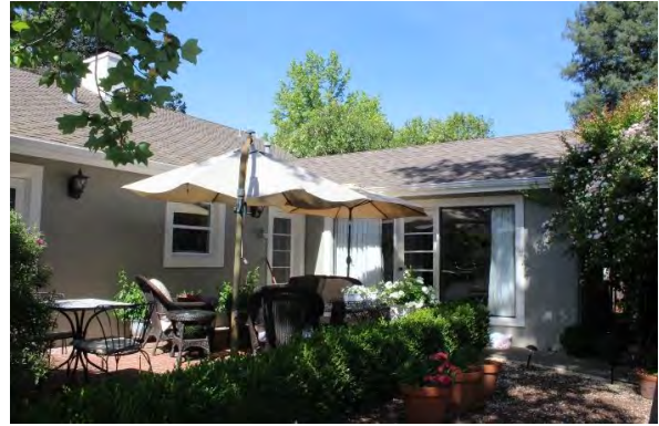
Photograph 7: Rear of house, camera facing west, May 11, 2018.
