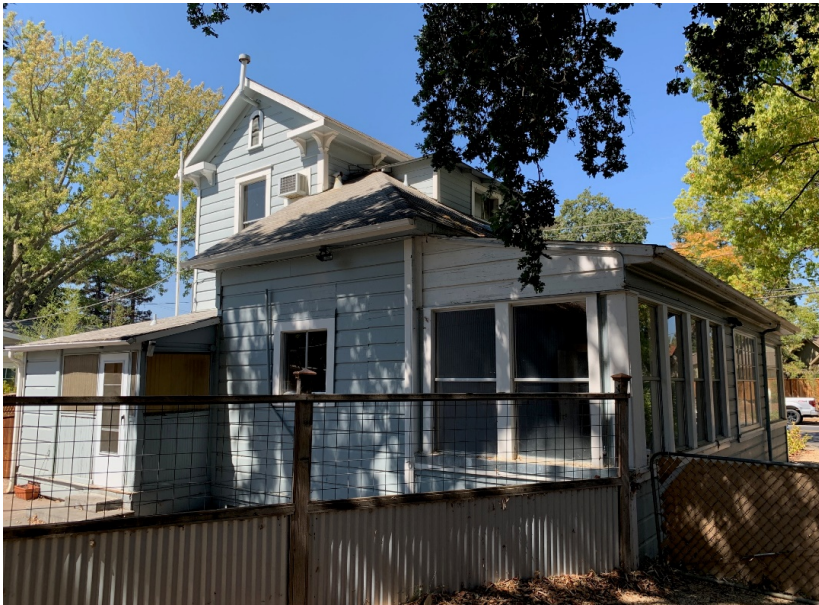
Photograph 5: 951 Pope Street, southeast and northeast elevations, camera facing northwest, September 6, 2021.
