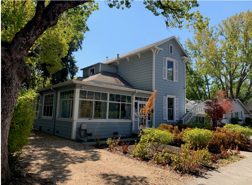
Photograph 6: 951 Pope Street, northeast and northwest elevations, camera facing south, September 6, 2021.
