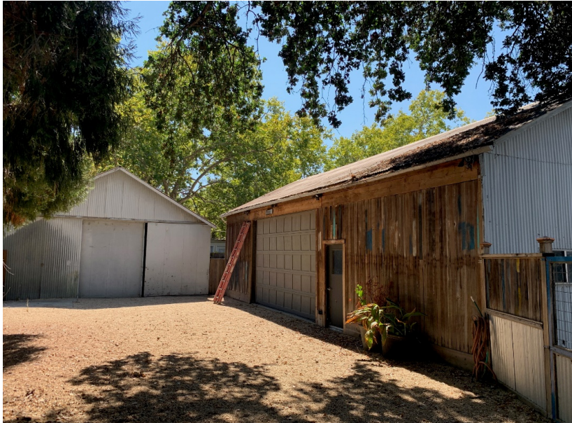
Photograph 8: 951 Pope Street barns, northeast and northwest elevations, camera facing south, September 6, 2021.
