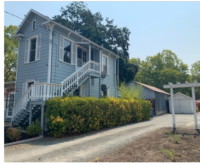
2 Front west corner of Site showing exterior staircase and driveway for adjacent property at 963 Pope Street
