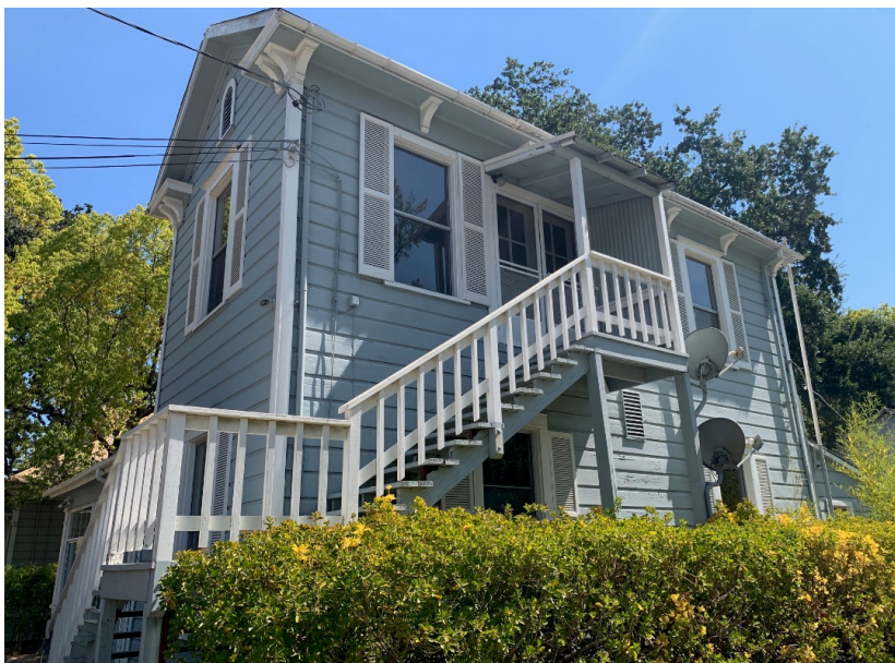
Photograph 3: 951 Pope Street, northwest and southwest elevations, camera facing east, September 6, 2021.
