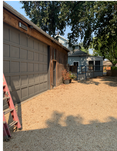
Northeast side of large garage and driveway; residence is in background
