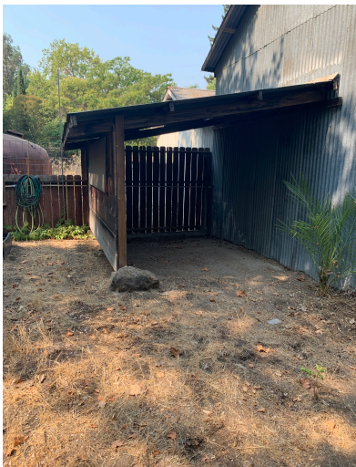
Shed along back side of large garage
