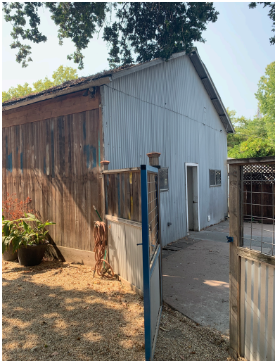
North corner of large garage viewed from driveway; residence is to the right
