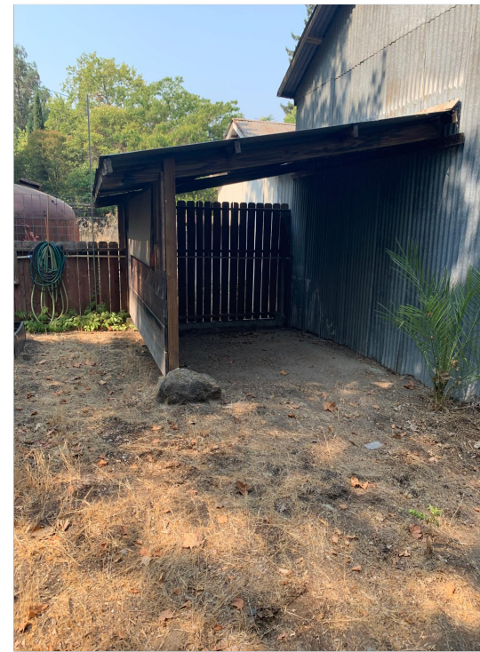
7 Shed along back side of large garage
