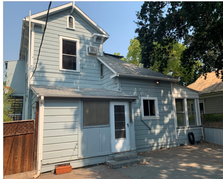
3 Back of residence showing adjacent concrete hardscape; additions are on the right
