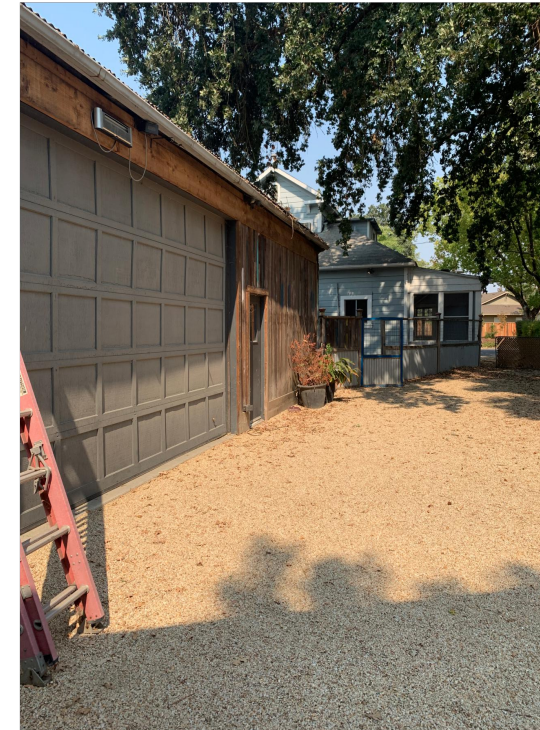
6 Northeast side of large garage and driveway; residence is in background
