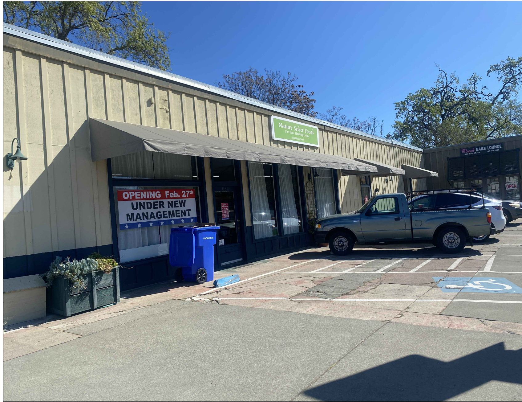
3 A-2.01 EXISTING FRONT VIEW (ST. HELENA HWY) SCALE N.T.S RETAIL AREA
