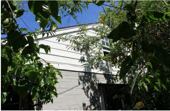
Photograph 6: Southeast elevation, camera facing northwest, May 11, 2018.
