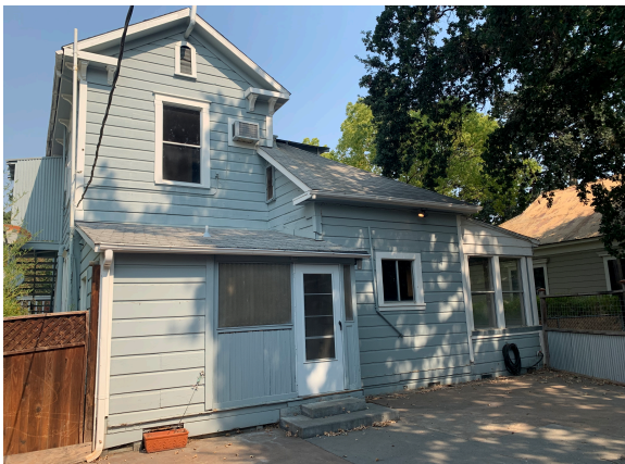
Back of residence showing adjacent concrete hardscape; additions are on the right
