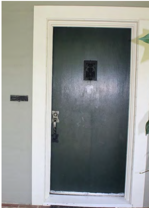
Photograph 4: Detail, front door, camera facing northeast, May 11, 2018.
