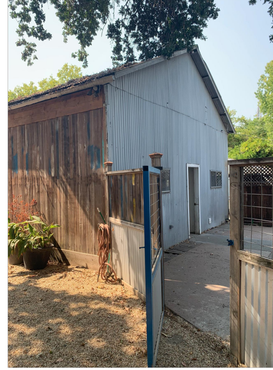
5 North corner of large garage viewed from driveway; residence is to the right
