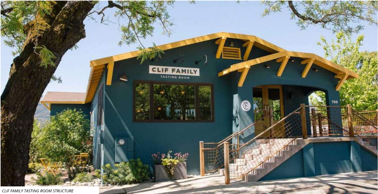
CLIF FAMILY TASTING ROOM STRUCTURE
