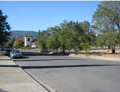
View of Adams Street looking southwest.
