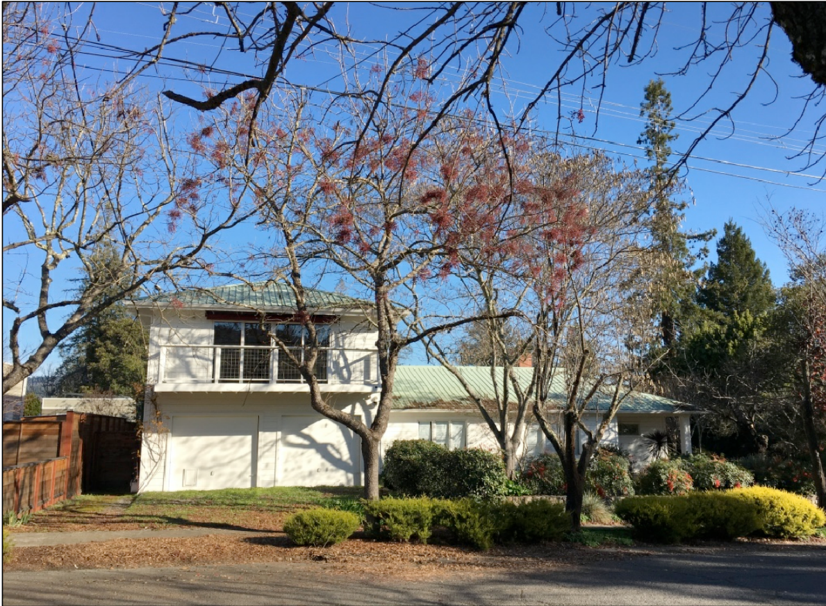
MAIN FACADE, SUBJECT PROPERTY FROM SCOTT STREET
