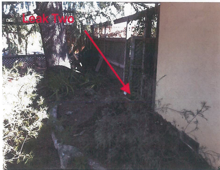
Leak Two: Lateral irrigation line leak located under the potted plant to the right of the entrance to the backyard. ICV that controls this zone is located approximately 5' to the right of the leak location in a Christy Box in front of a crawlspace vent.
