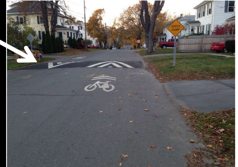
Figure 3.10.2. Speed Hump on Residential Neighborhood Street (Source: Lucy Gibson)
