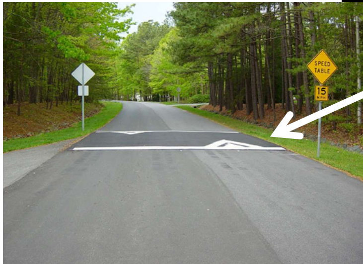
Figure 3.12.1. Typical Speed Table Application (Source: www.pedbikeimages.org / Austin Brown)
