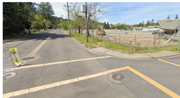
Most curb ramps are not current ADA-compliant
