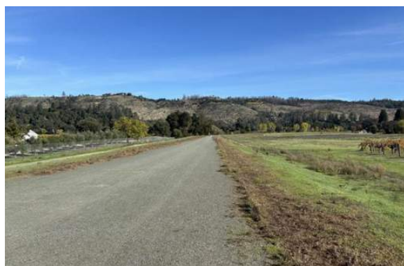
View from top of existing levee looking towards the Napa River
