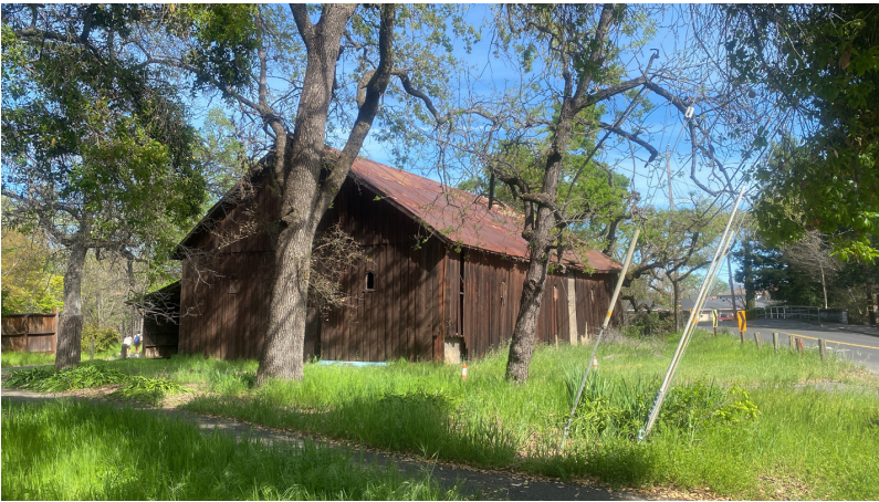
Existing conditions at Signorelli Barn,
