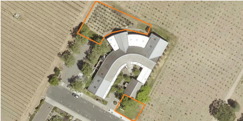
Outdoor space around the Public Library, outlined in orange.
