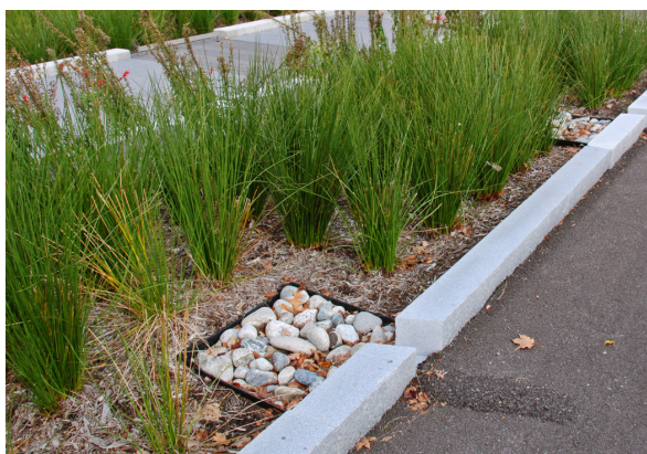
Bioretention Bulbout
