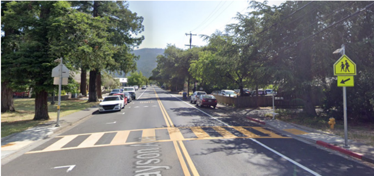
This crossing outside of St. Helena High School includes a high-visibility crosswalk, ADA-compliant curb ramps, and an RRFB
