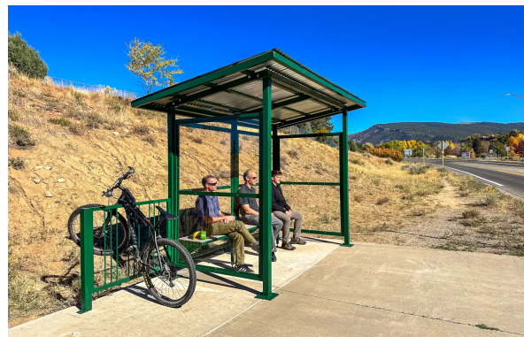
Transit shelters can provide shade and relief from the elements, aiding cyclists in transitioning to buses or other forms of public transportation
