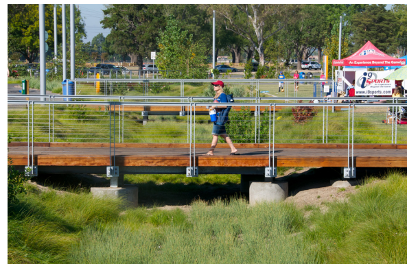
Elevated walkway over bioswale, Irvine, CA
