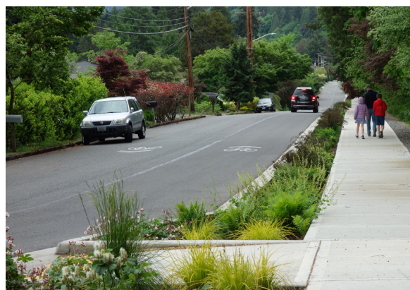
Bioretention Strip, Bellevue, Washington
