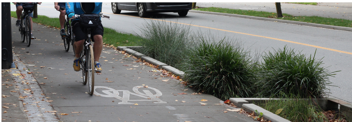
Biofiltration System, Vancouver, BC
