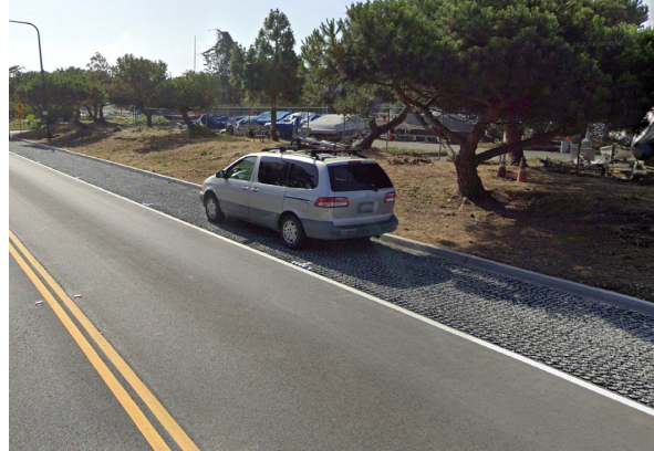
Pervious parking lane, Oakland, CA
